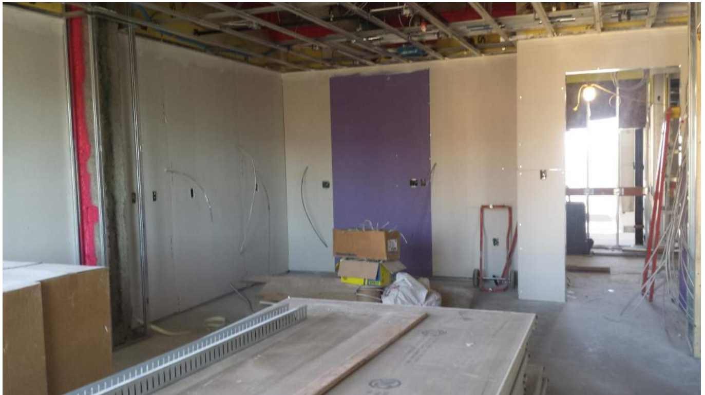
Level 5 typical unit progress (unit 1501 shown)
