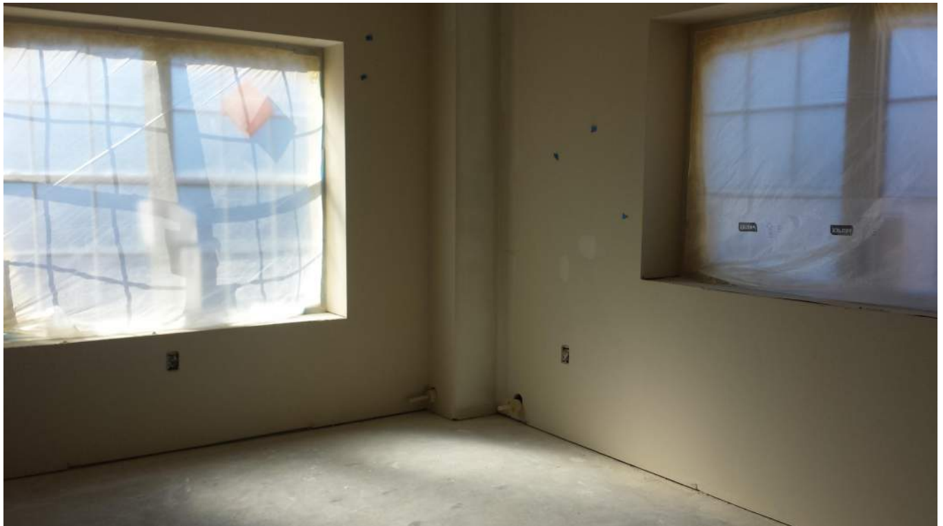
New tower construction at end of West wing looking south east
