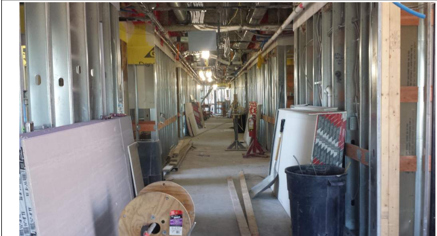
New tower construction level 5 west wing
