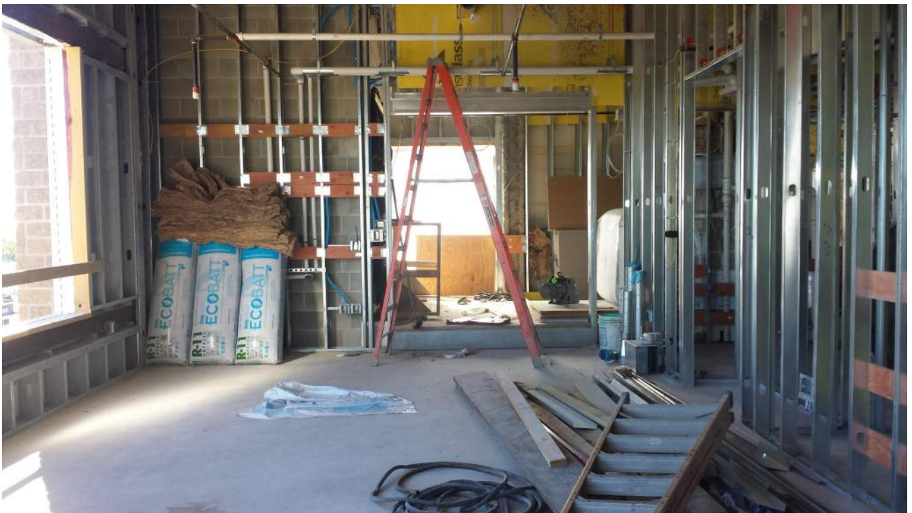
Level 5 community room
