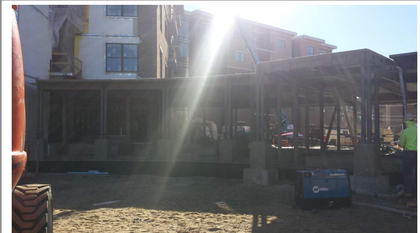
Connector construction, entry side
