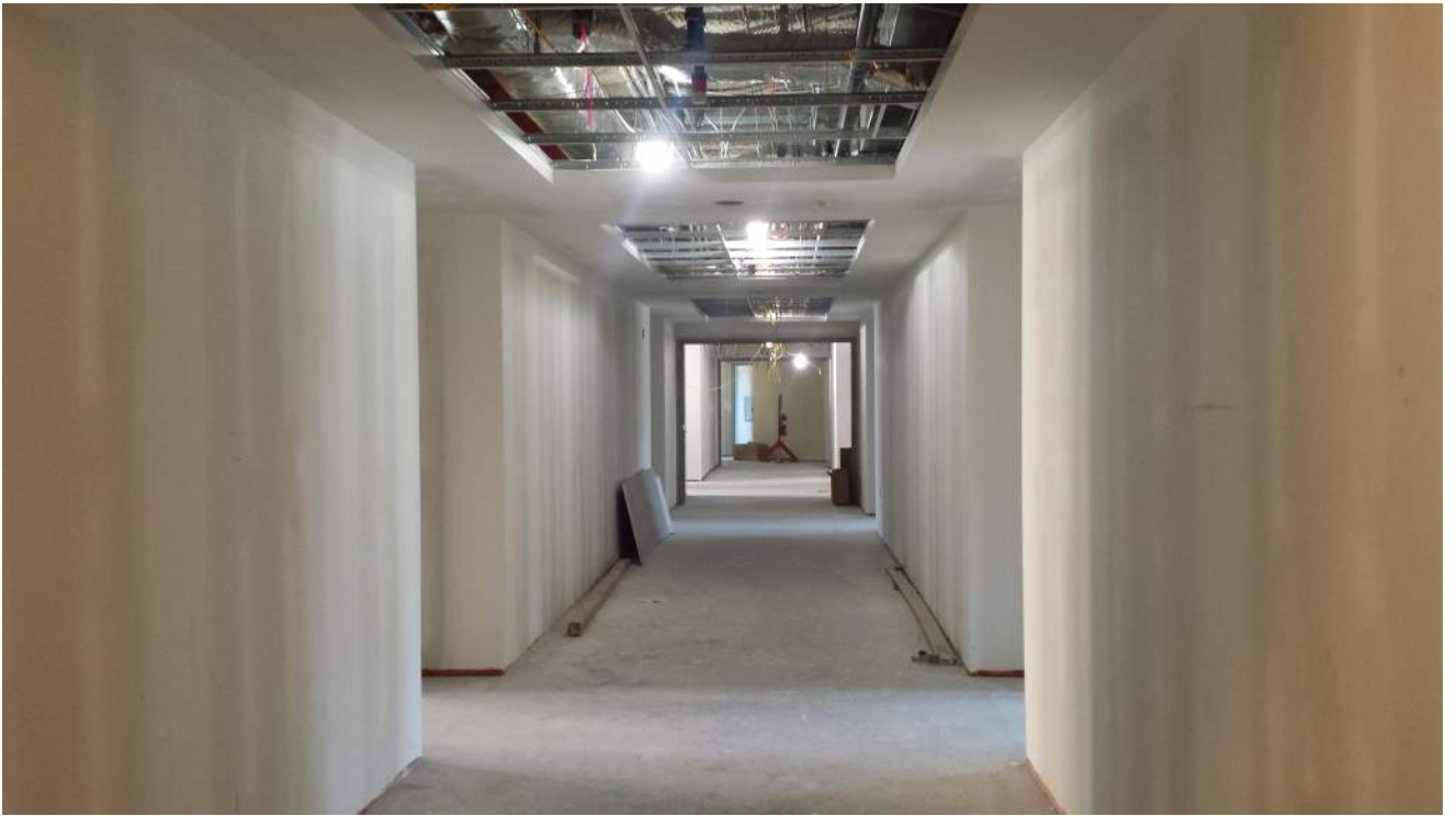
New tower construction level 2 corridor east wing
