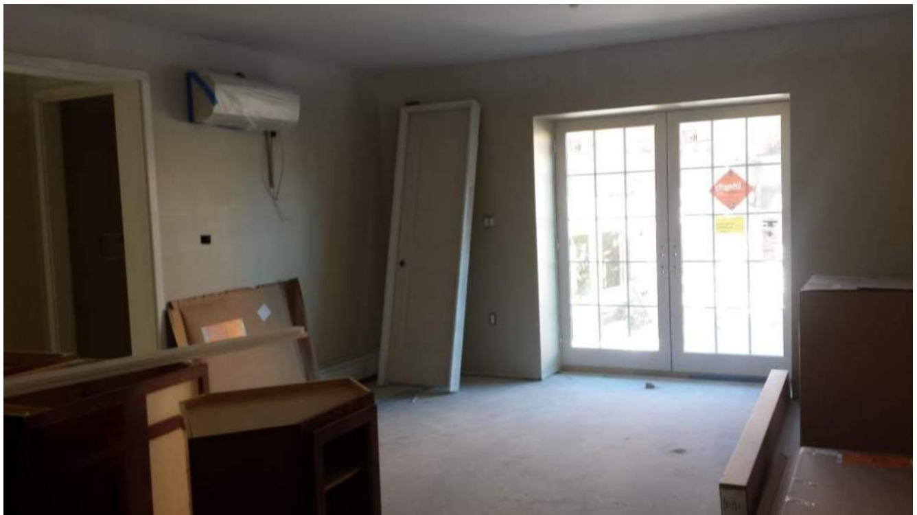
Level 1 typical unit progress (unit 1111 shown)
