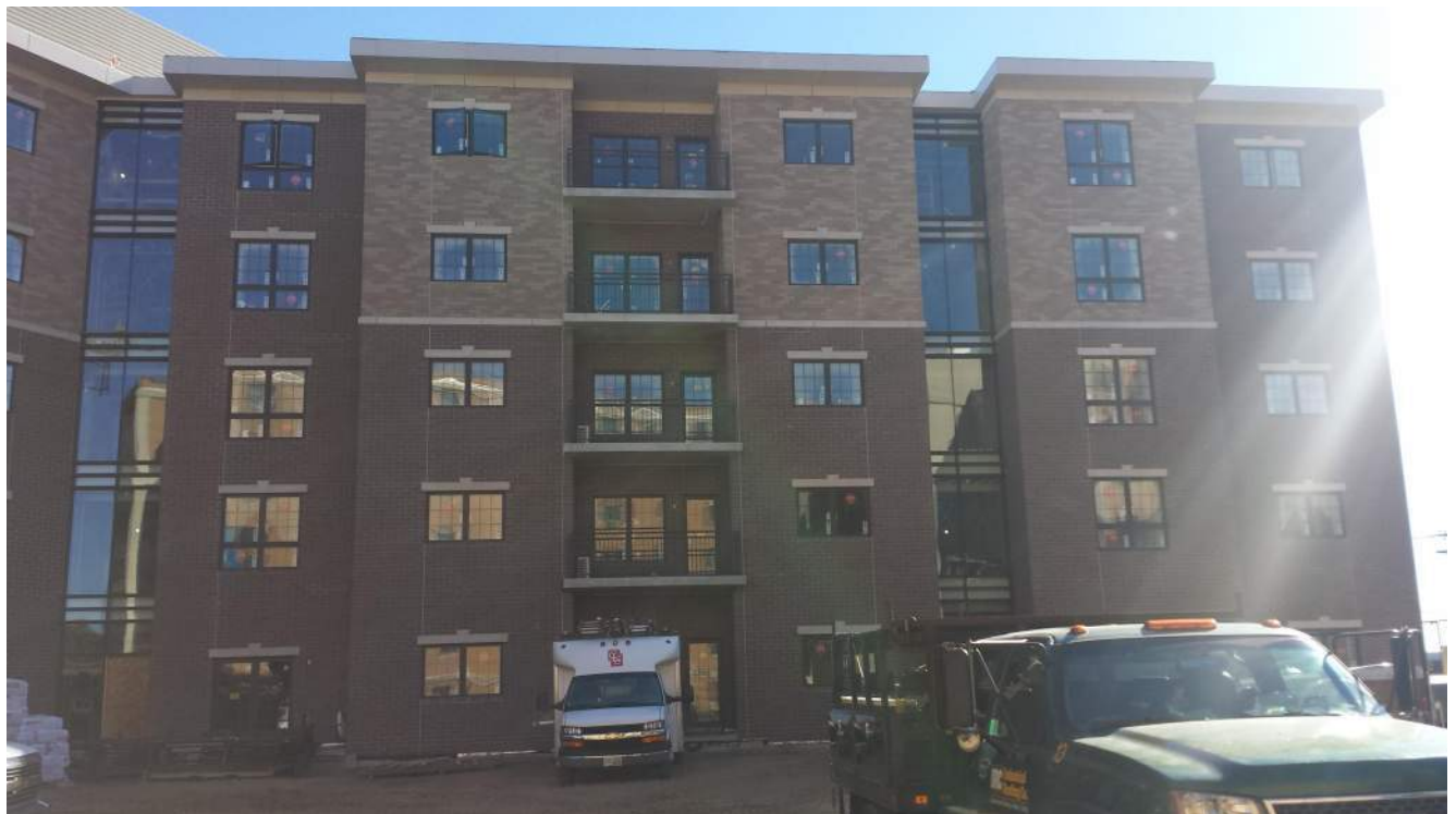
New tower construction east wing (courtyard side)
