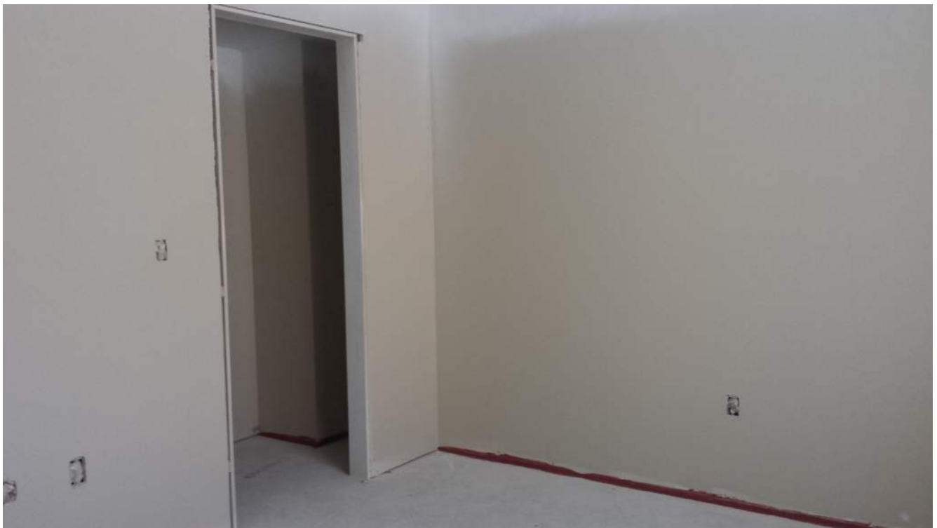
Level 3 typical unit progress (unit 1301 shown)
