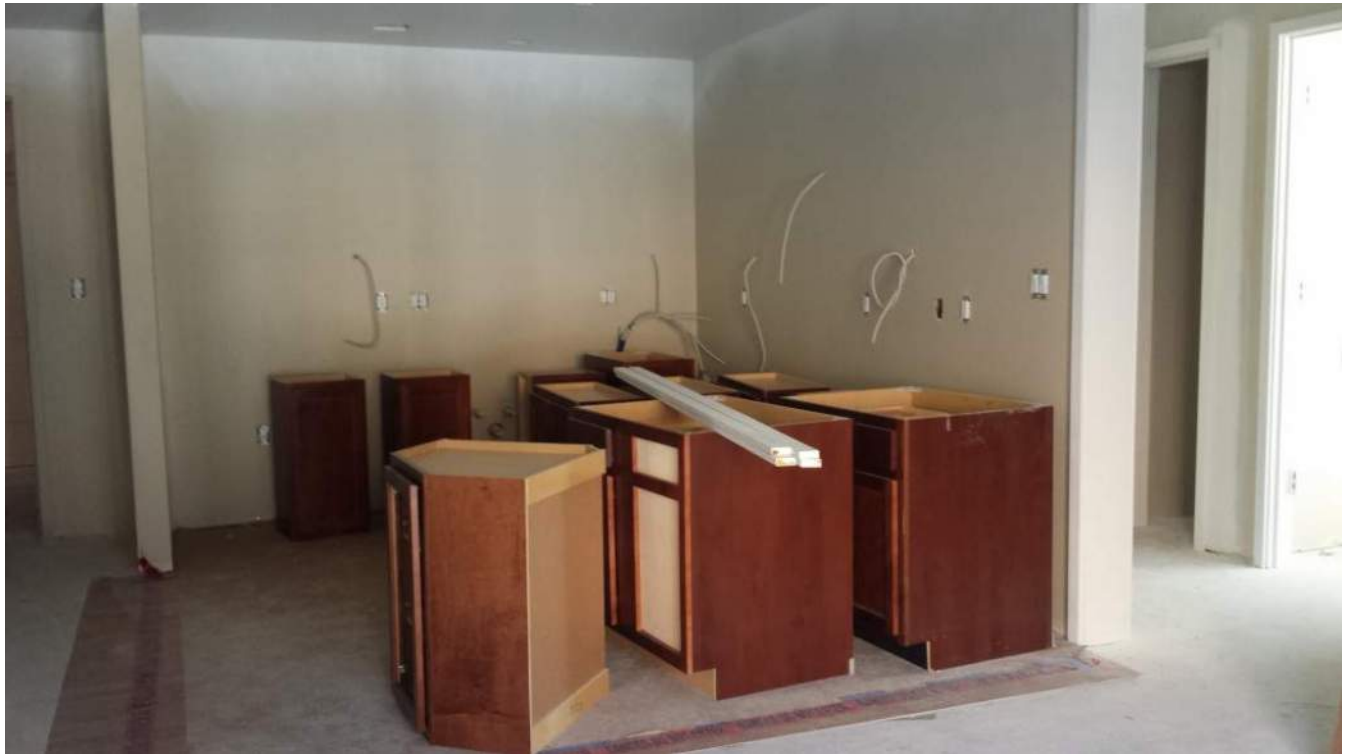
Level 1 typical unit progress (unit 1111 shown)
