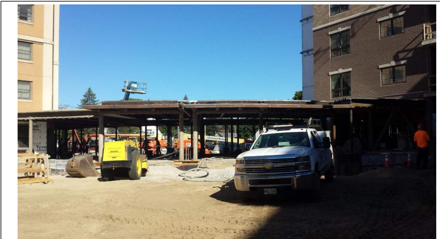
Connector construction, courtyard side
