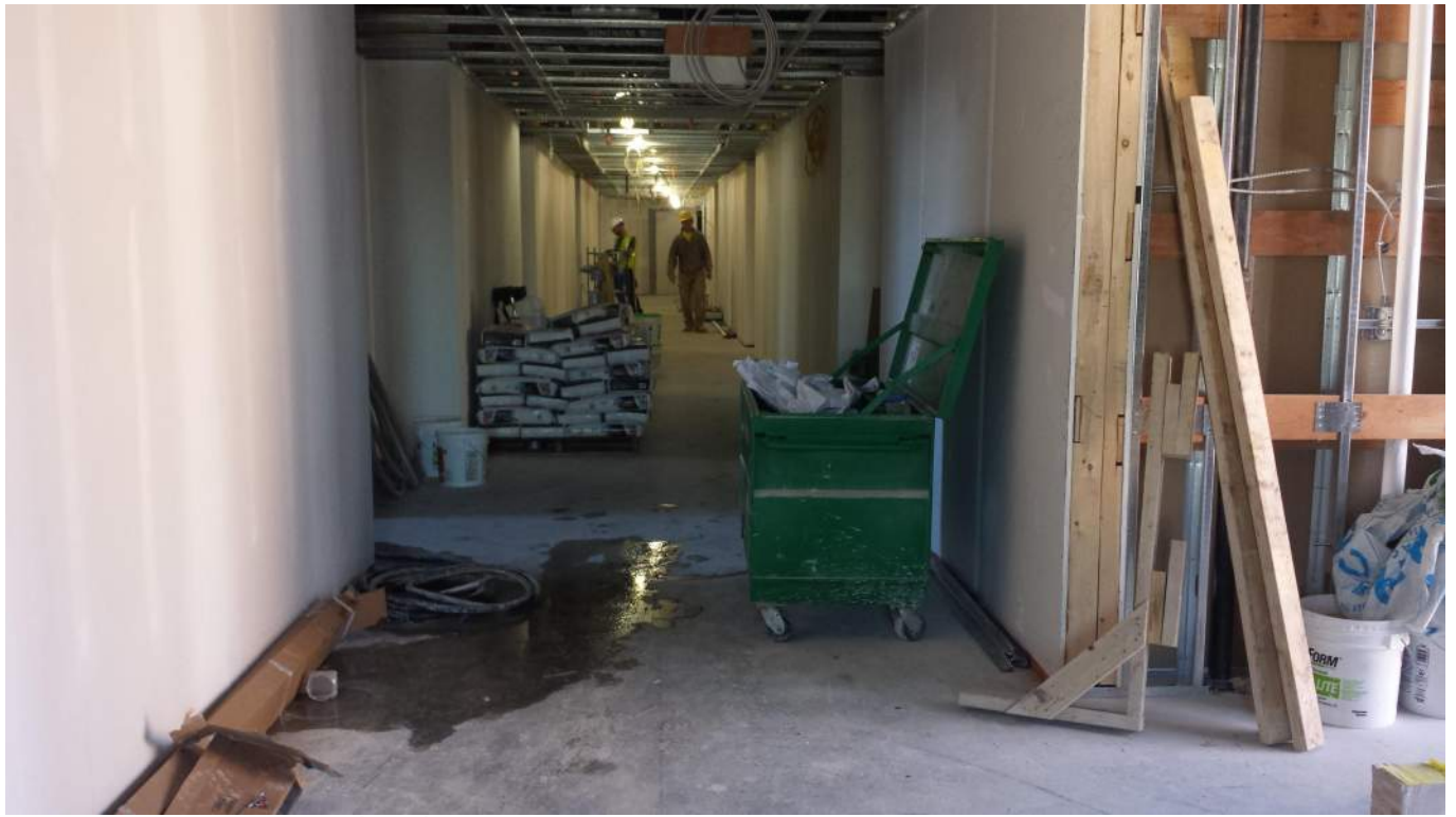
New tower construction level 3 west wing
