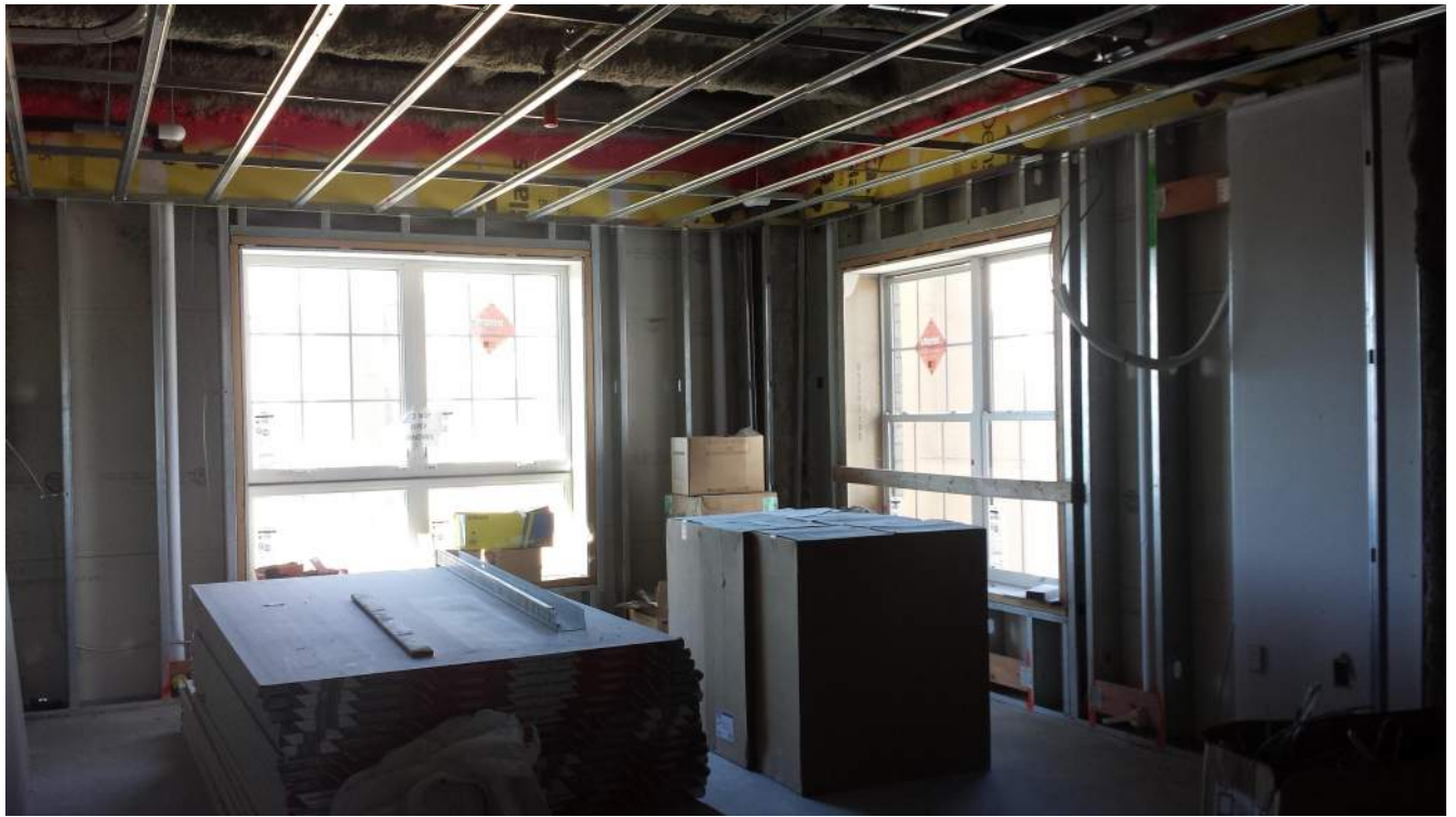
Level 5 typical unit progress (unit 1501 shown)
