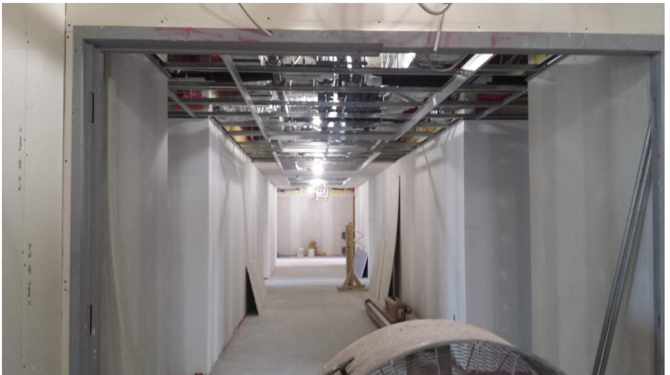
New tower construction level 3 east wing
