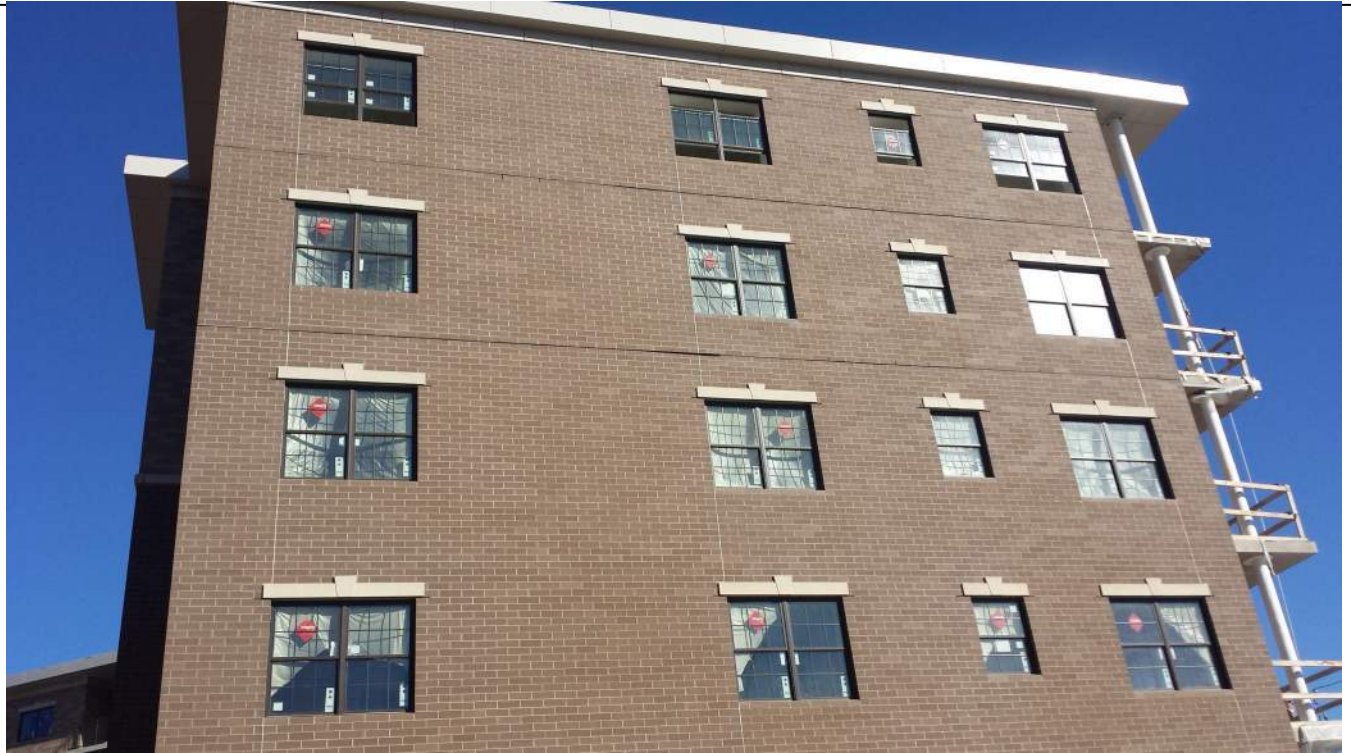
New tower construction east wing over garage entrance
