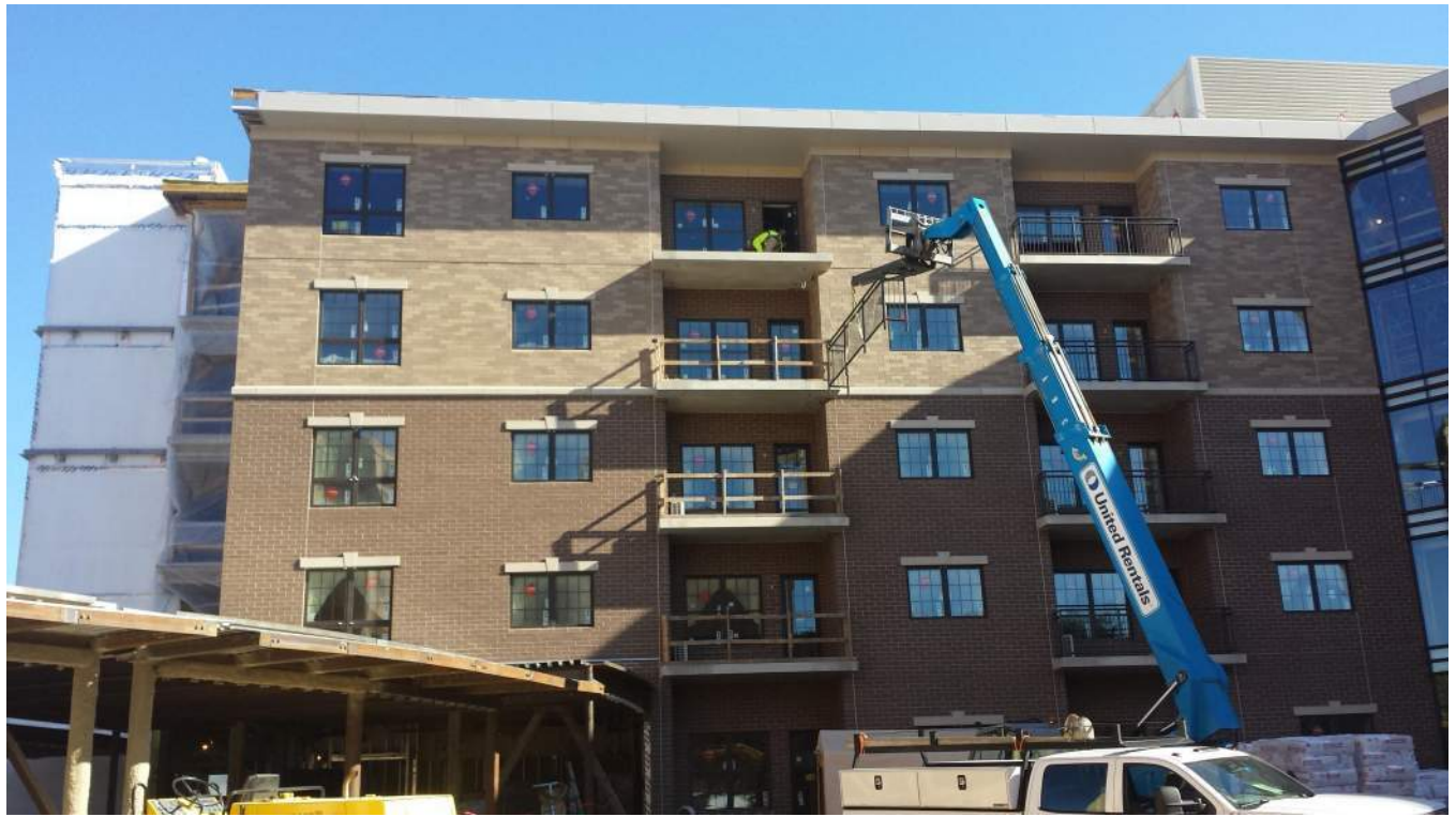
New tower construction west wing (courtyard side)
