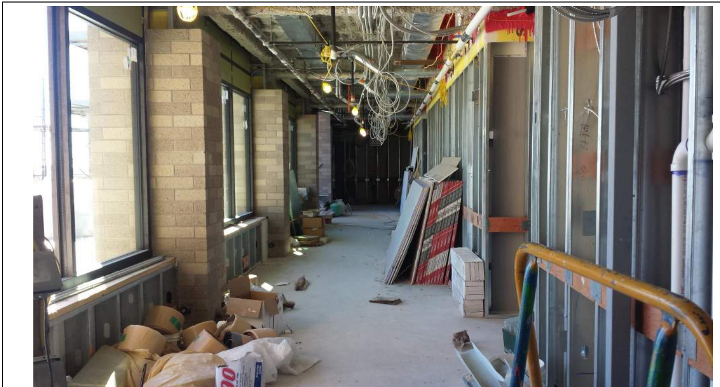
New tower construction level 5 east wing
