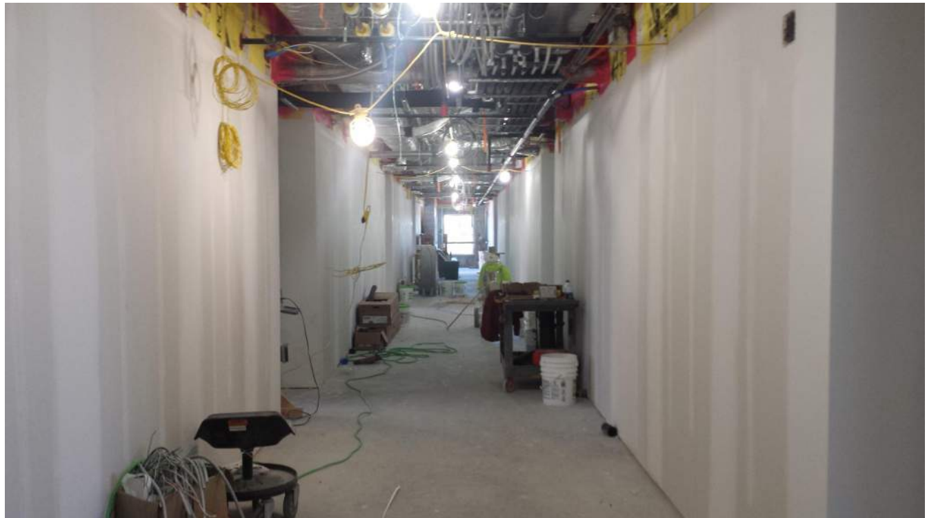
New tower construction level 4 west wing
