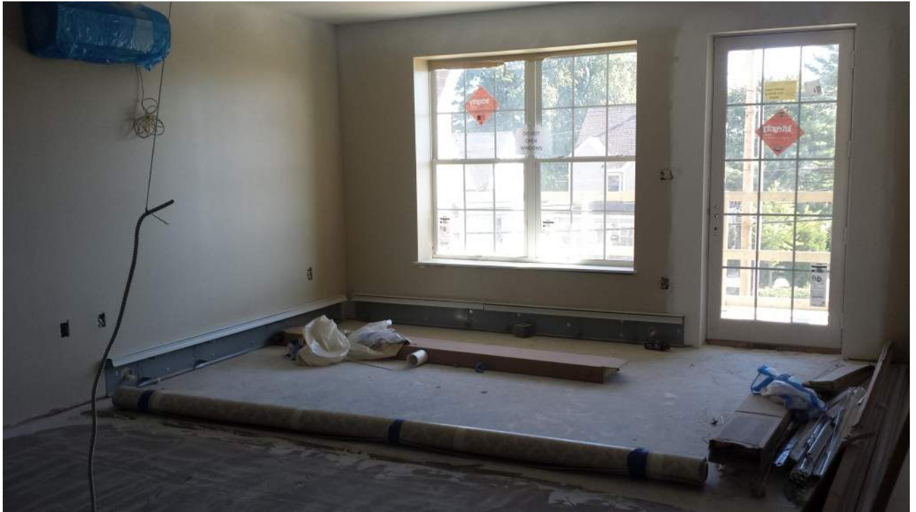
Level 2 typical unit progress (unit 1210 shown)
