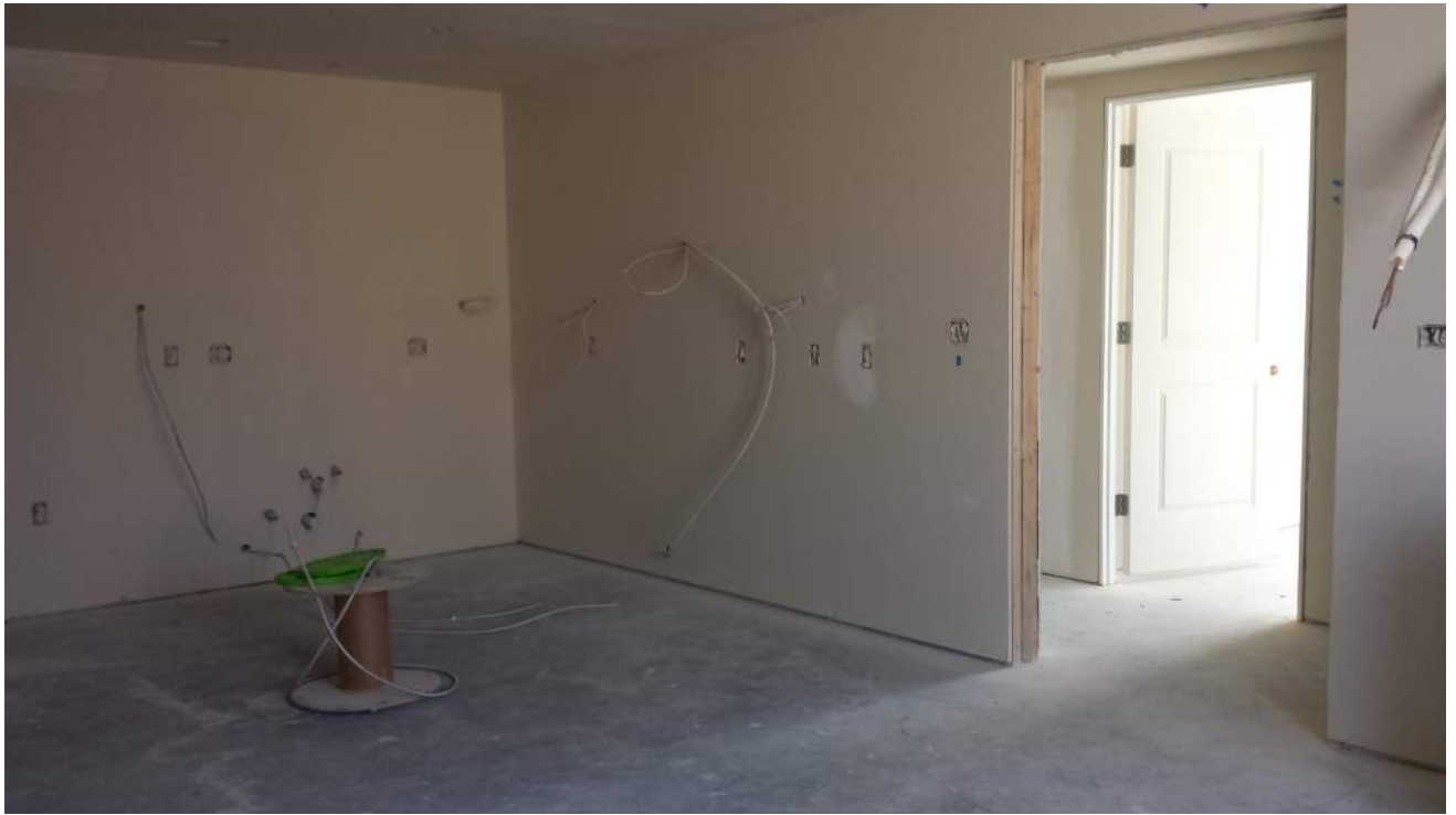
Level 4 typical unit progress (unit 1411 shown)
