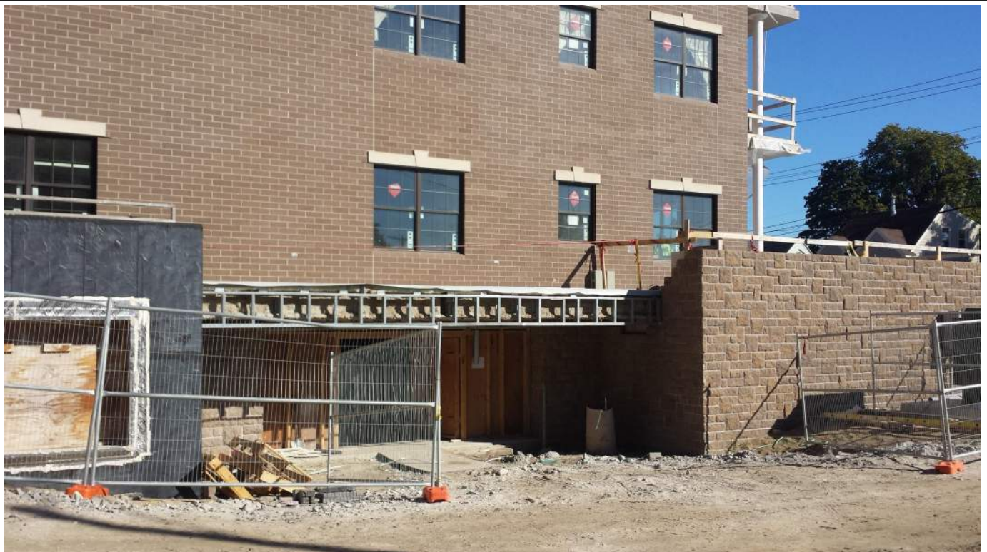
New tower construction east wing garage entrance
