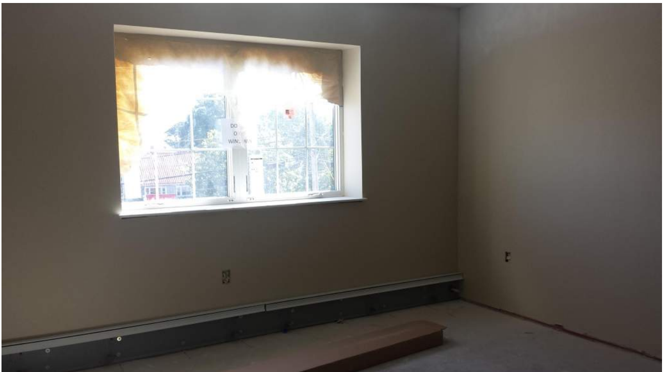
Level 2 typical unit progress (unit 1210 shown)
