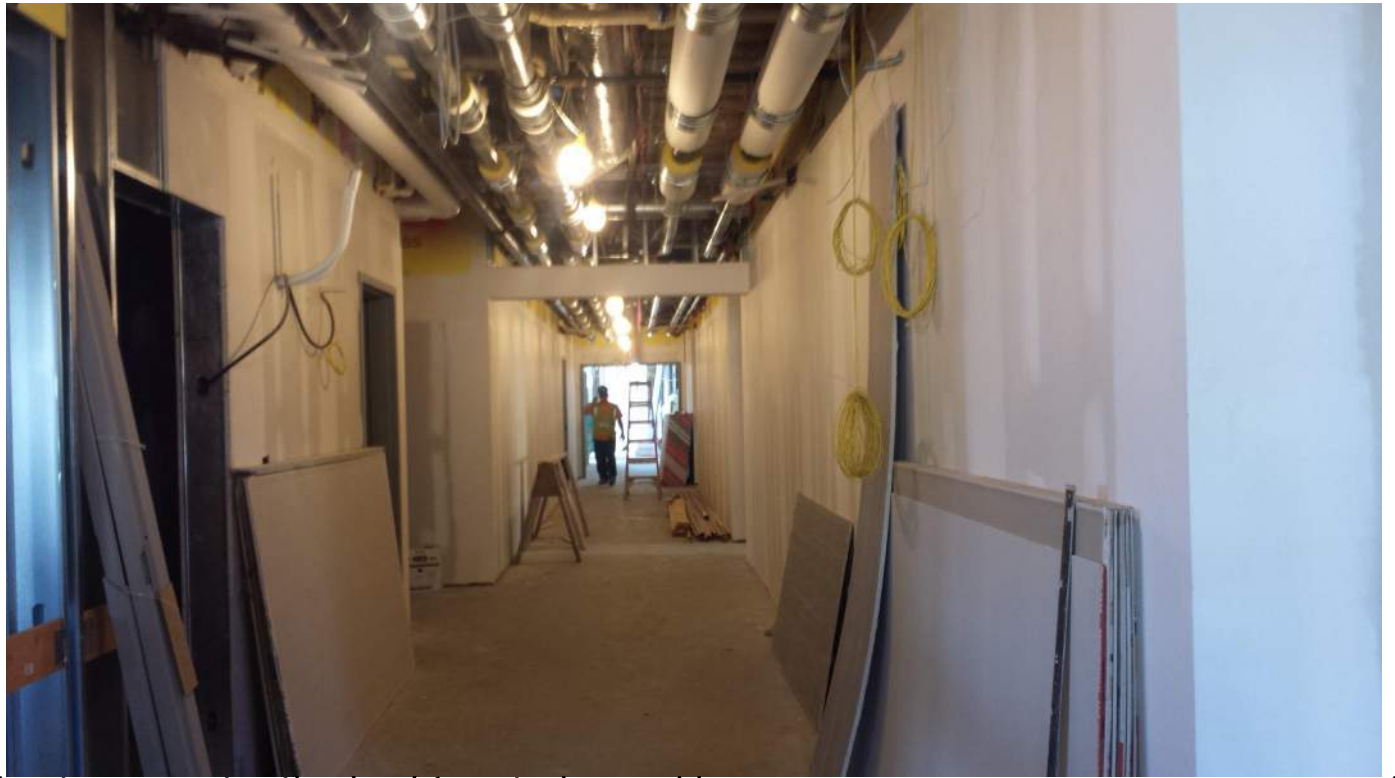
New tower construction level 1 west wing corridor
