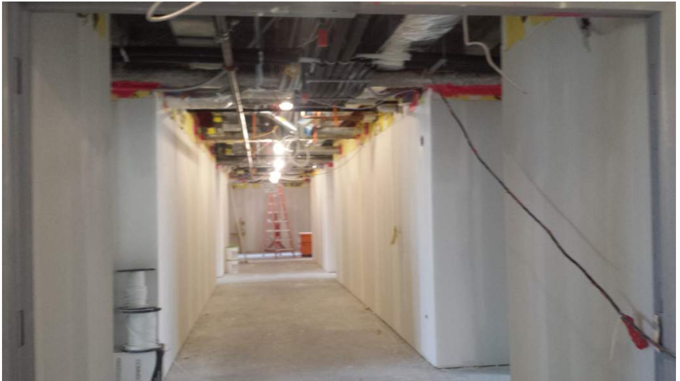
New tower construction level 4 east wing
