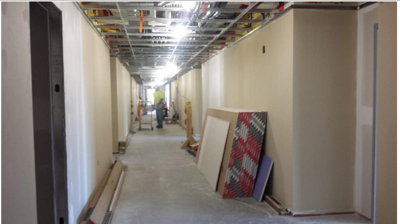
New tower construction level 2 corridor west wing
