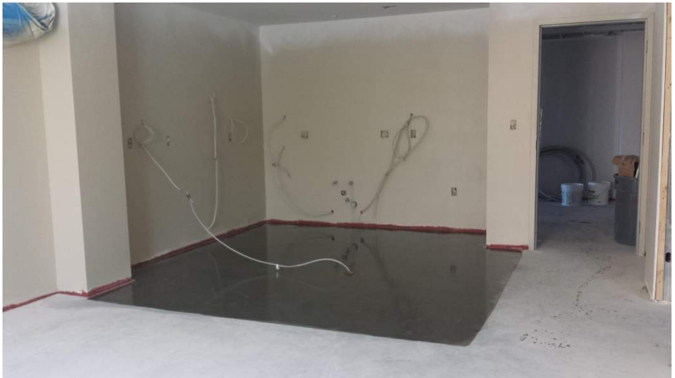
Level 3 typical unit progress (unit 1301 shown)
