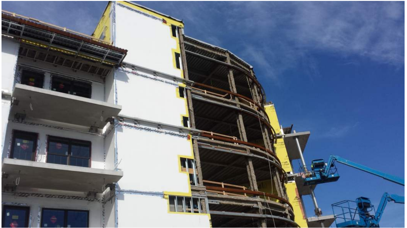
NEW TOWER CONSTRUCTION AT KNUCKE (FOREST AVE. SIDE)
