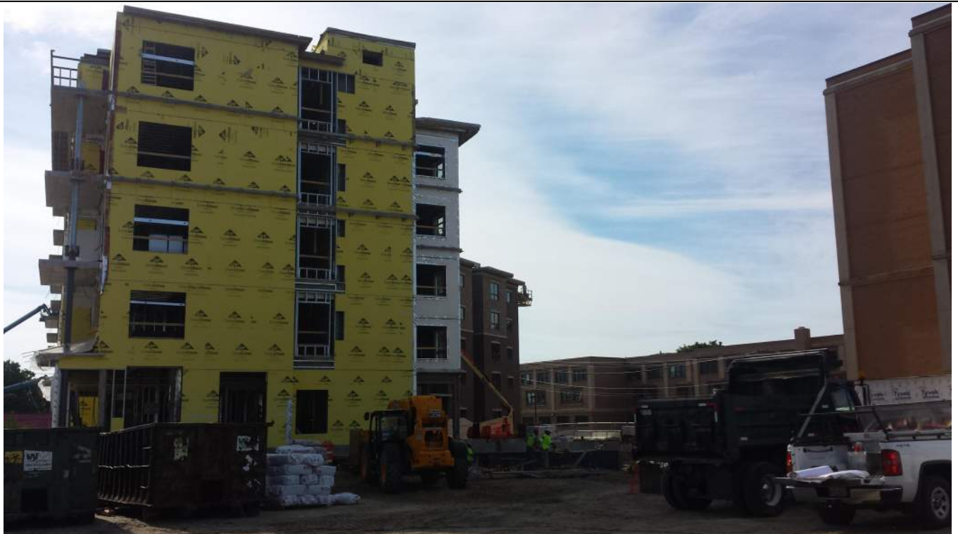
new tower construction from Arbor St. looking South
