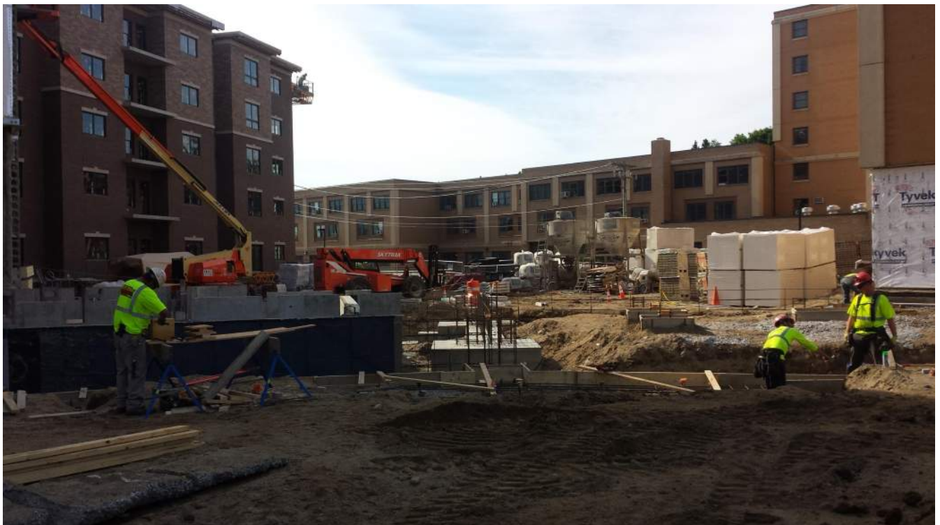
CONNECTOR CONSTRUCTION FROM TRAFFIC CIRCLE
