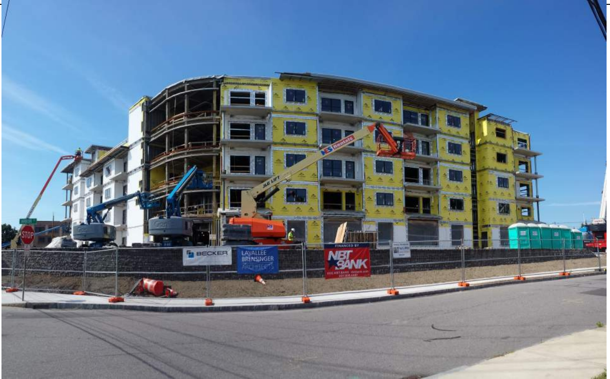
New tower construction from Forest Ave at Arbor St.
