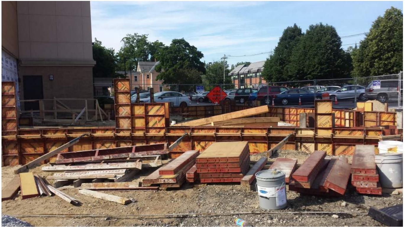
CONNECTOR CONSTRUCTION FROM TRAFFIC CIRCLE
