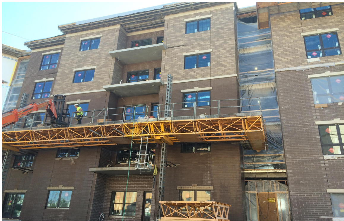
East Tower (Courtyard Side) brick cleaning in progress
