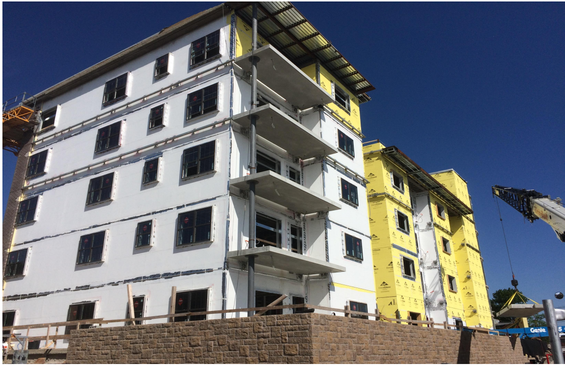
Brick Progress and Forest Ave precast balcony progress
