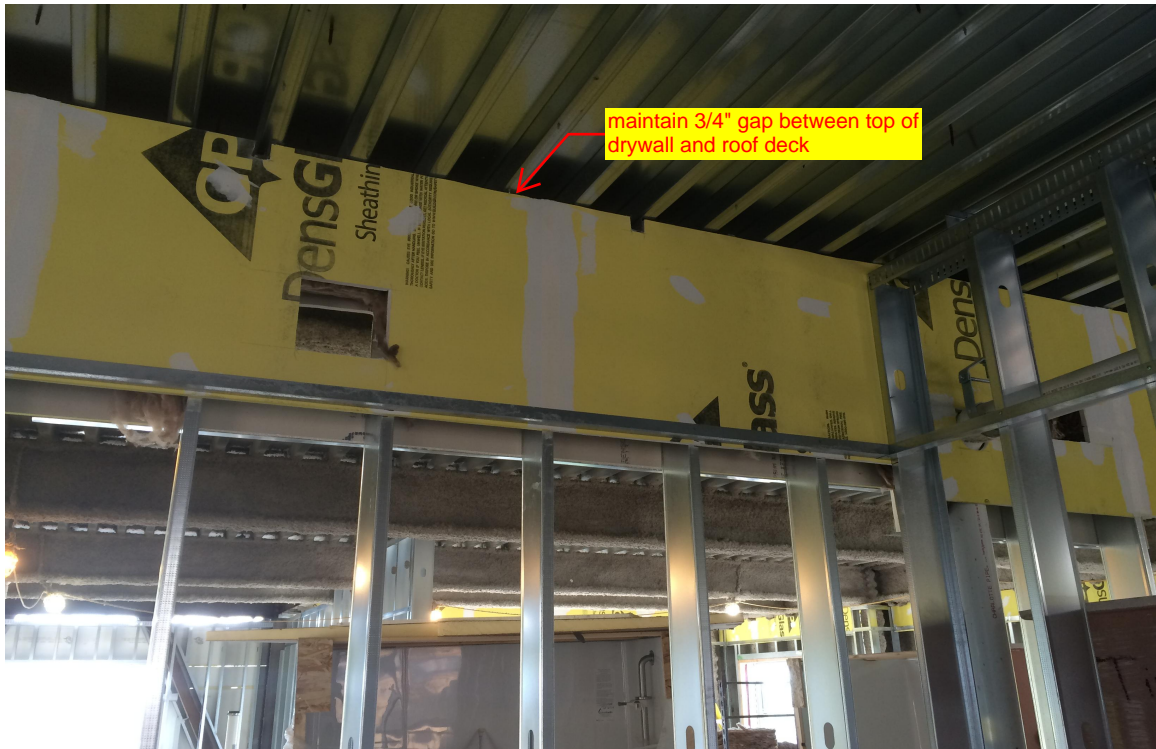
Top of wall detail - Level 5
