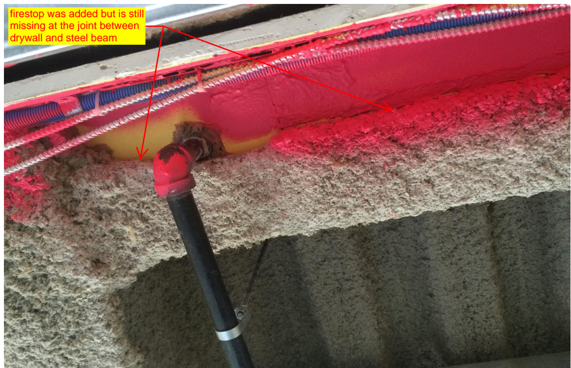
Top of wall detail above door 1111
