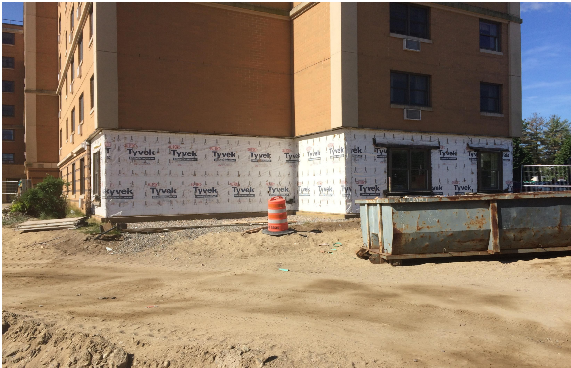
Selective demolition of existing building where new work intersects
