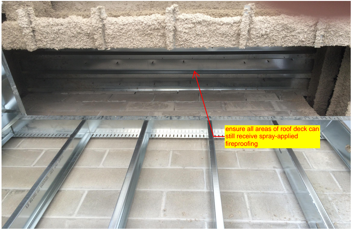
Elevator B top of shaft
