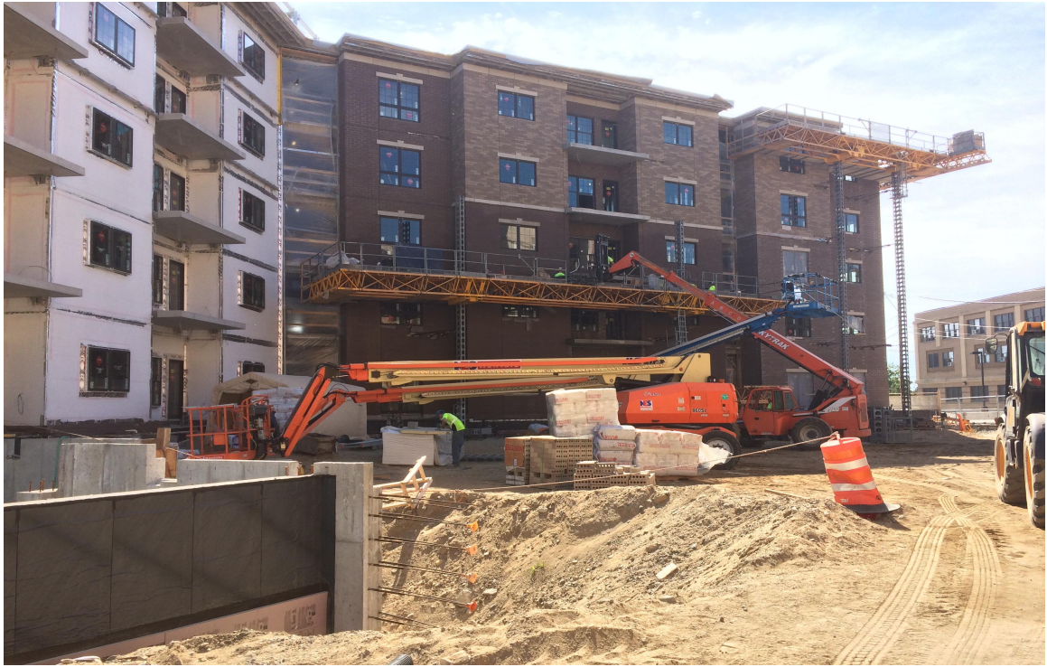
Brick progress East Tower (courtyard side)
