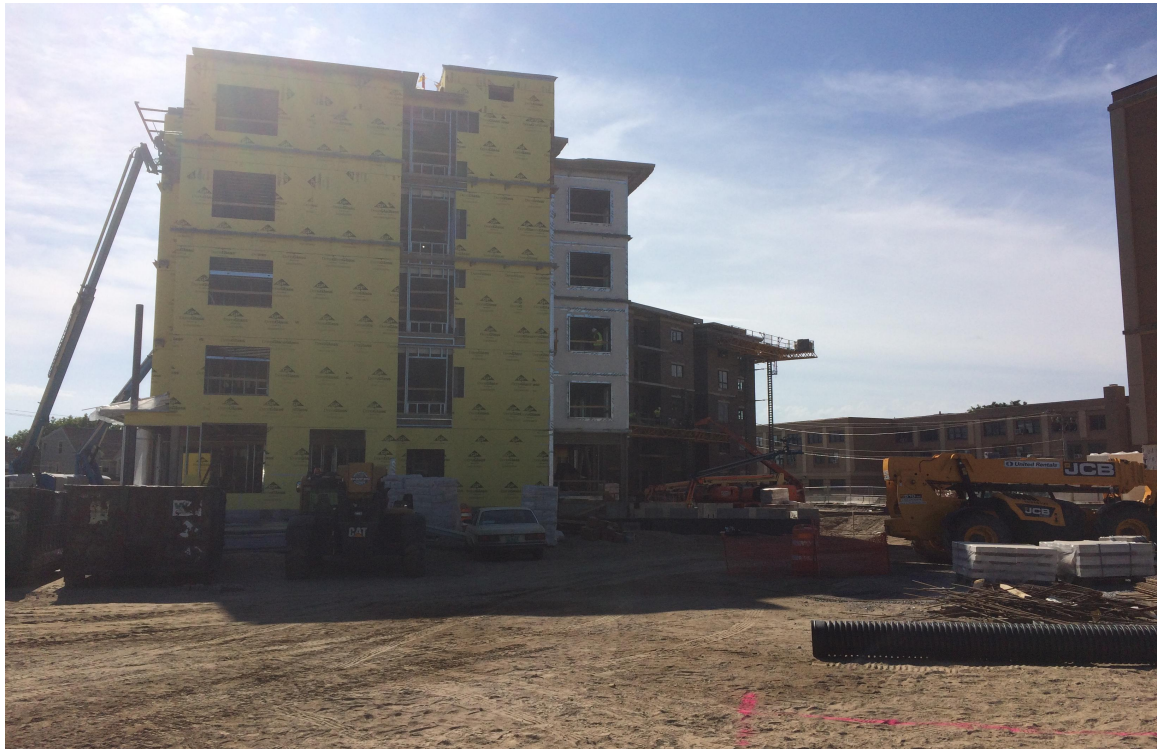
Tower construction site (from Arbor Street looking South)
