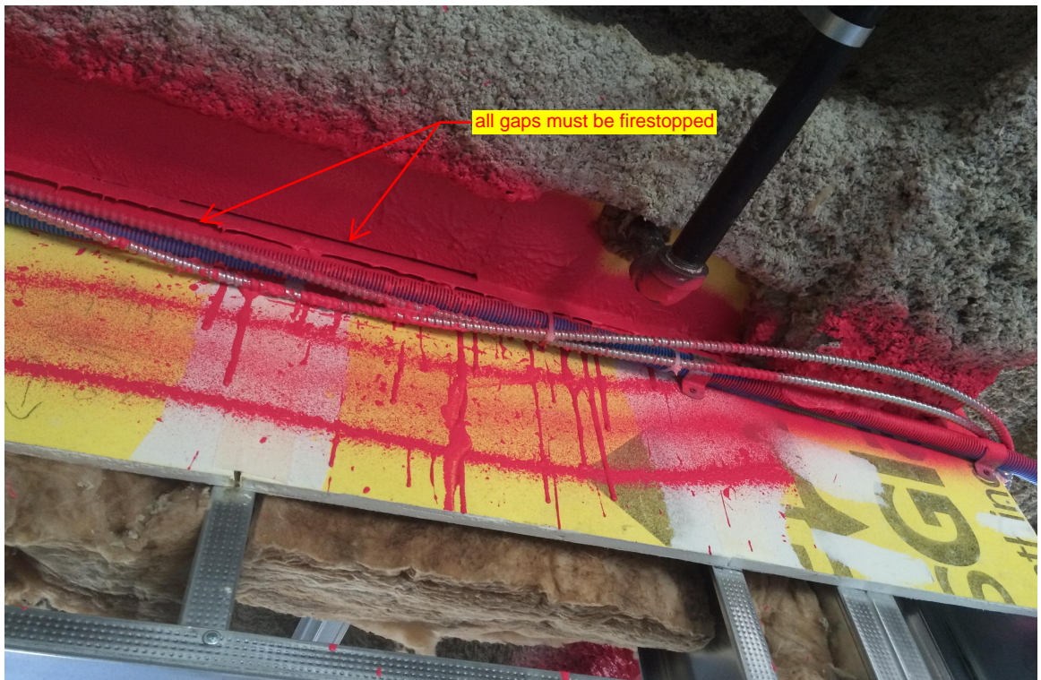
Top of wall detail above door 1111
