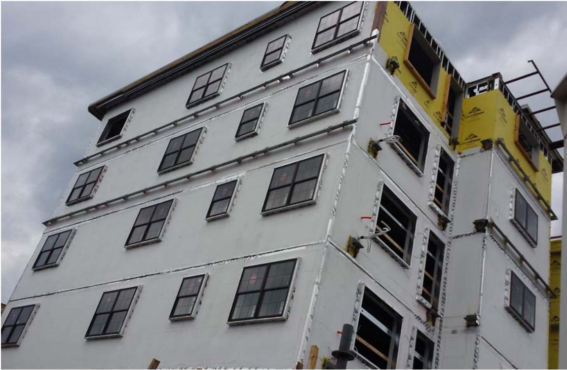
Tower east wing construction
