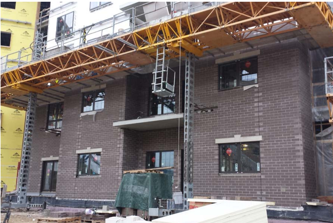
Courtyard side tower east wing masonry work.
