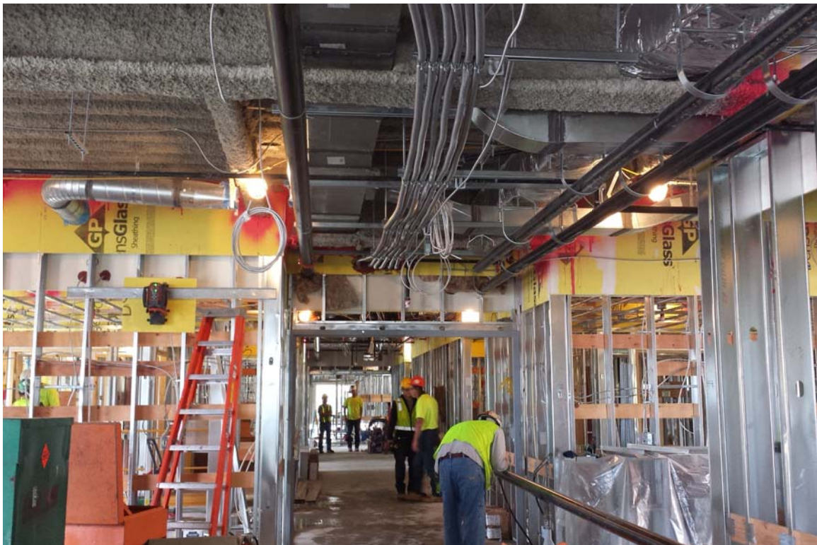
New tower construction, level 1, east wing
