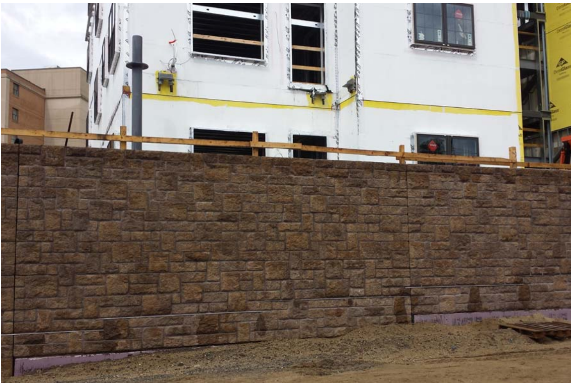
Terrace wall at Forest Ave.
