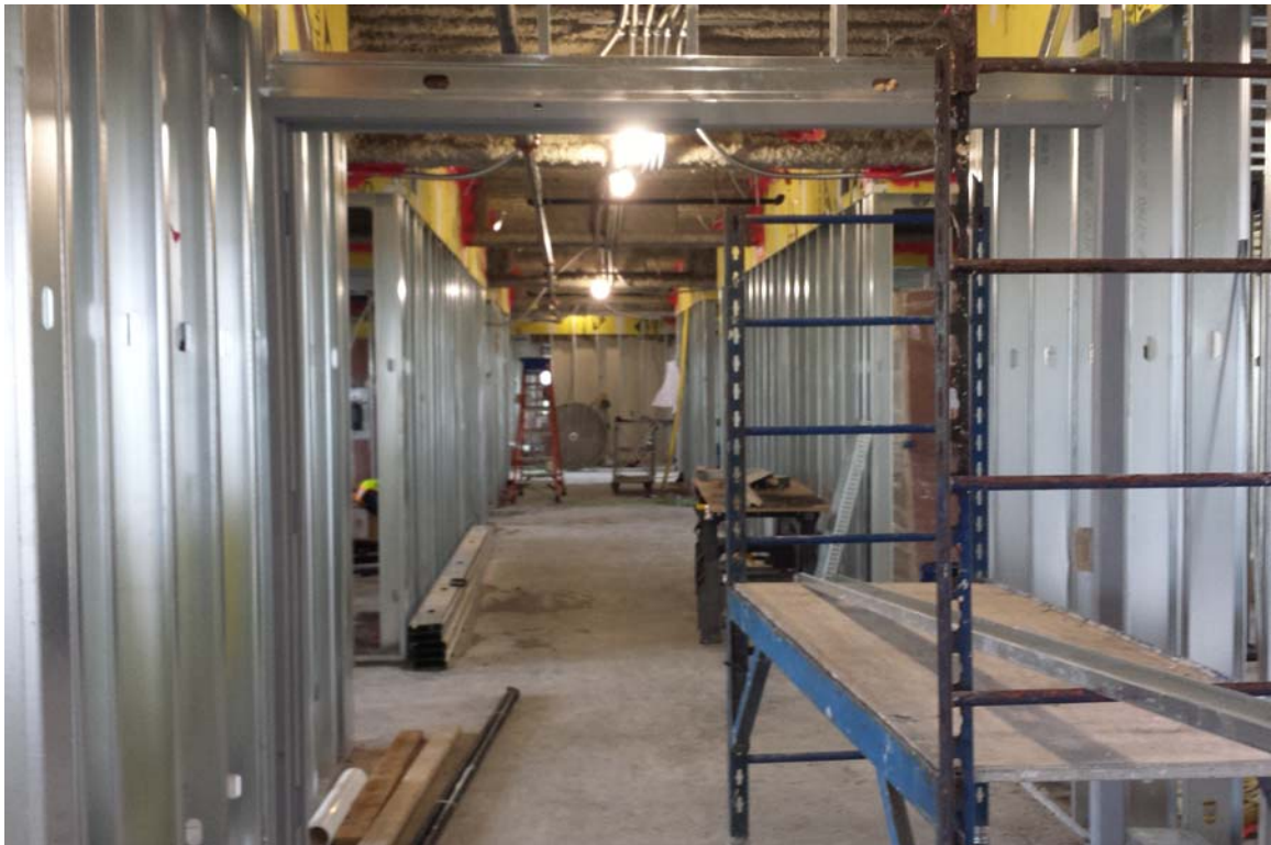
New tower construction, level 4, east wing
