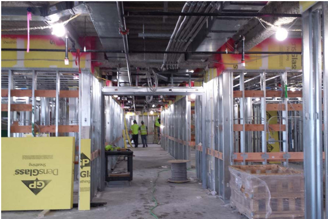
New tower construction, level 2, west wing
