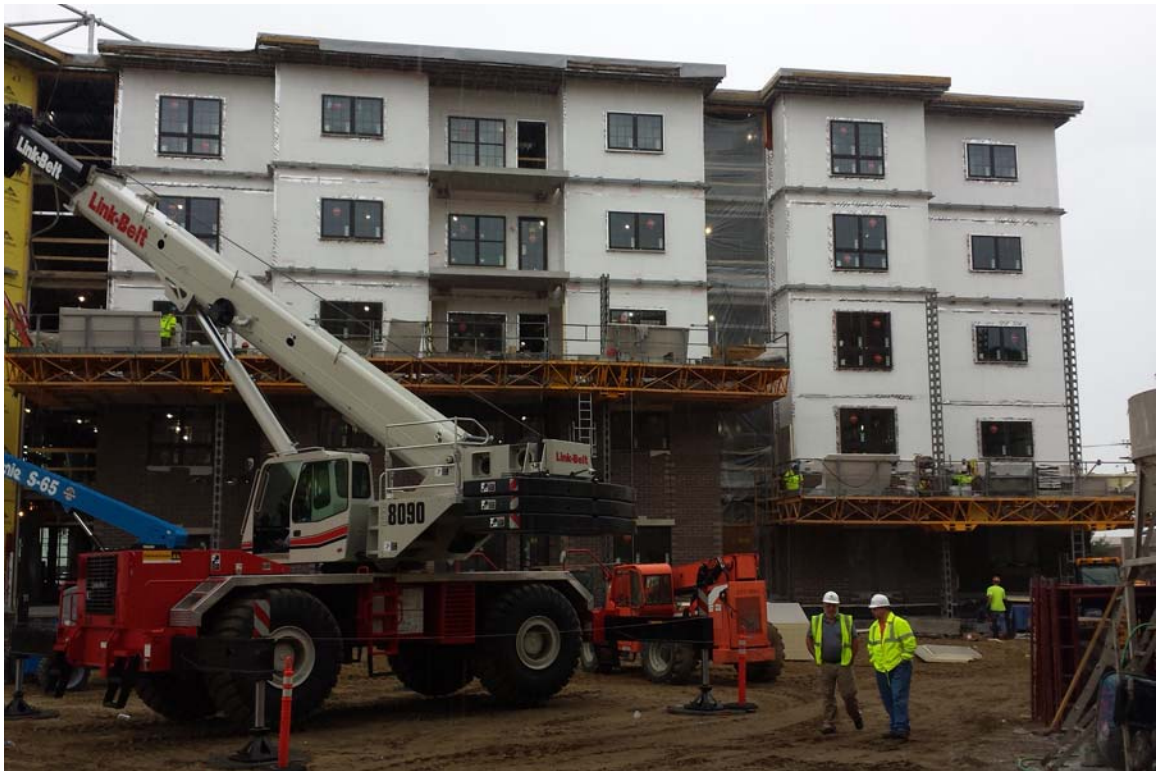
Tower east wing construction courtyard side
