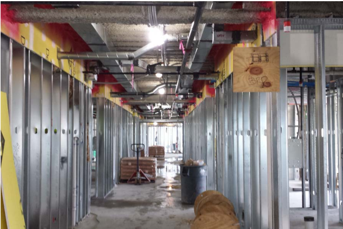
New tower construction, level 3, east wing
