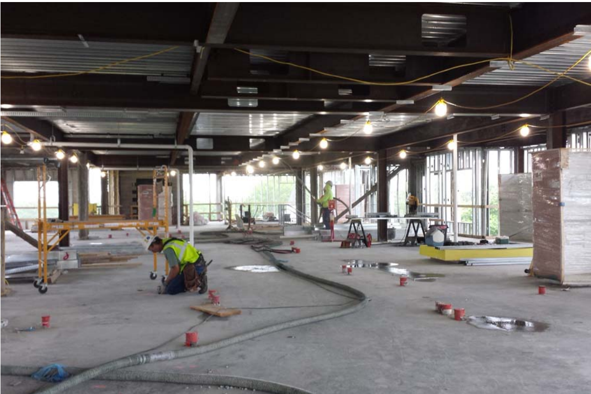
New tower construction, level 5, west wing
