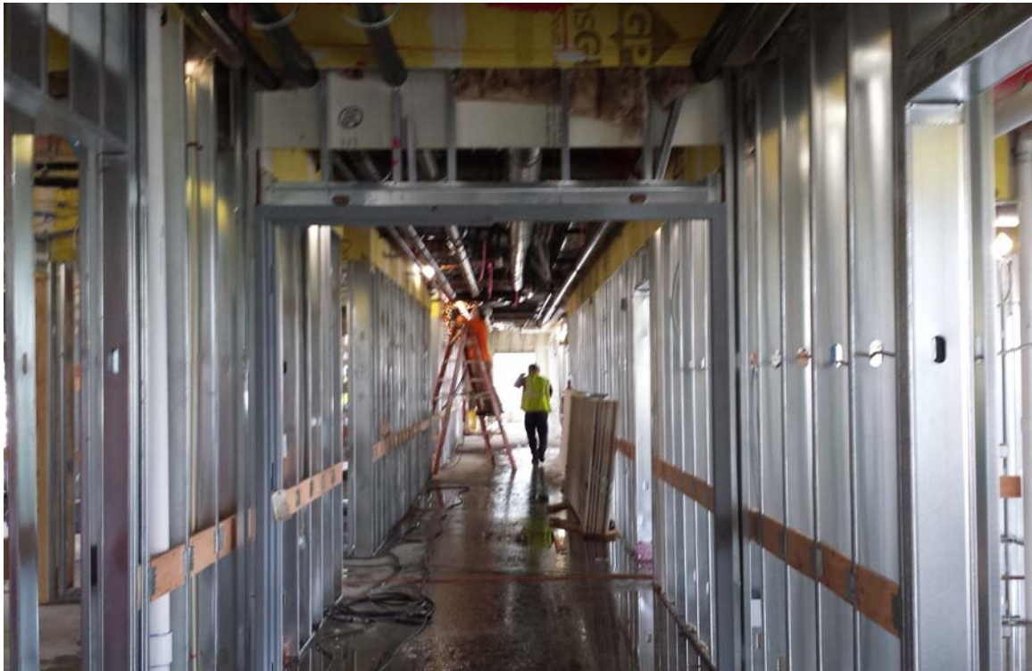
New tower construction, level 1, west wing
