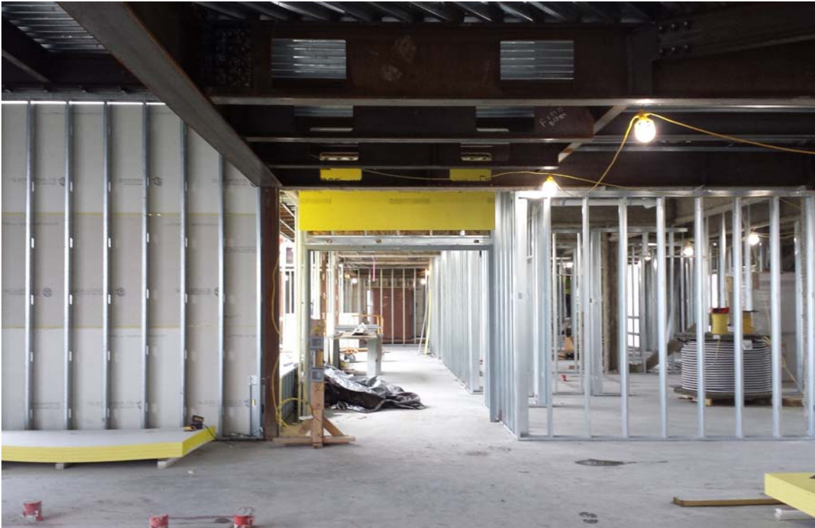
New tower construction, level 5, east wing
