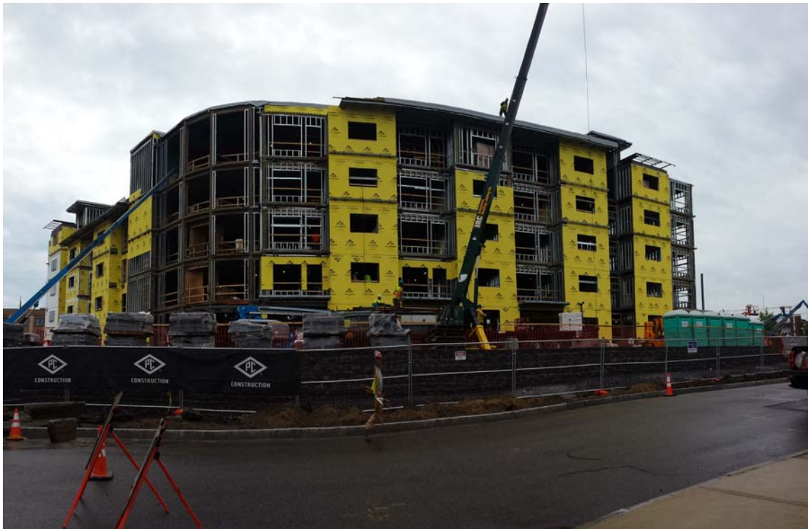
New tower construction at Forest Ave and Arbor Street
