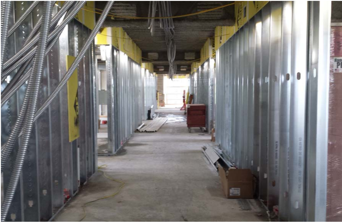
New tower construction, level 4, west wing
