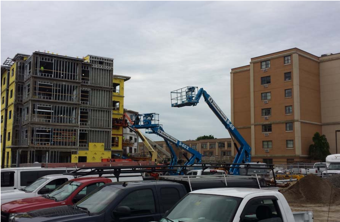
Tower west wing looking southeast
