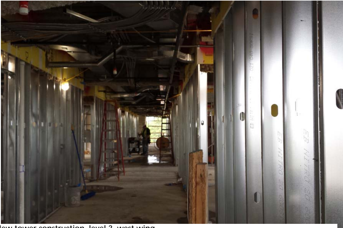
New tower construction, level 3, west wing
