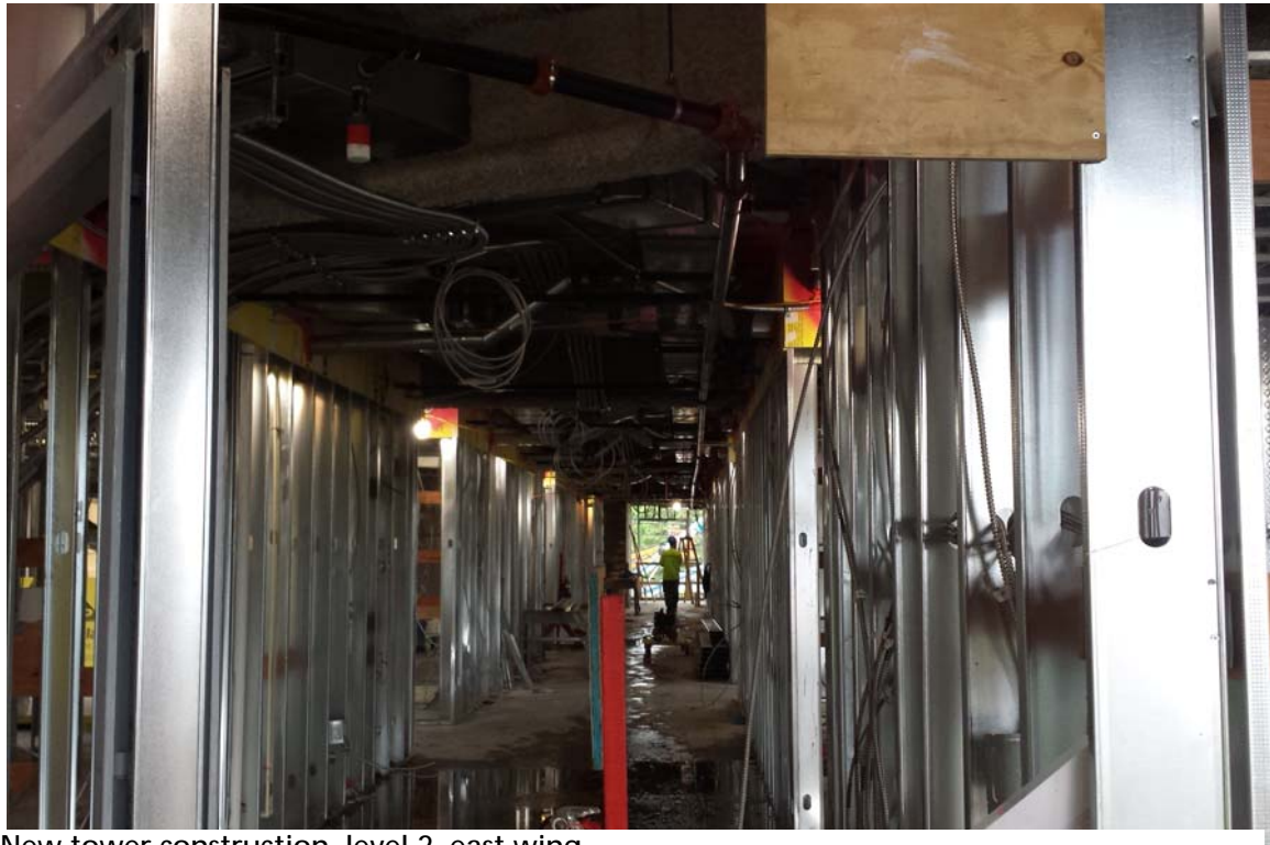
New tower construction, level 2, east wing
