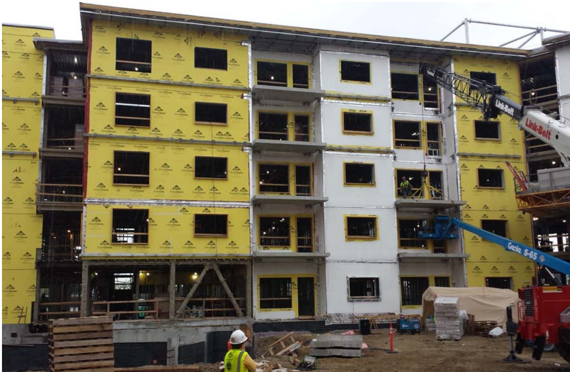
Tower west wing construction courtyard side
