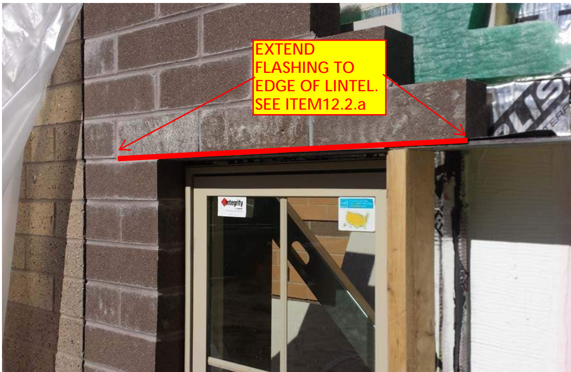
Mock up wall
