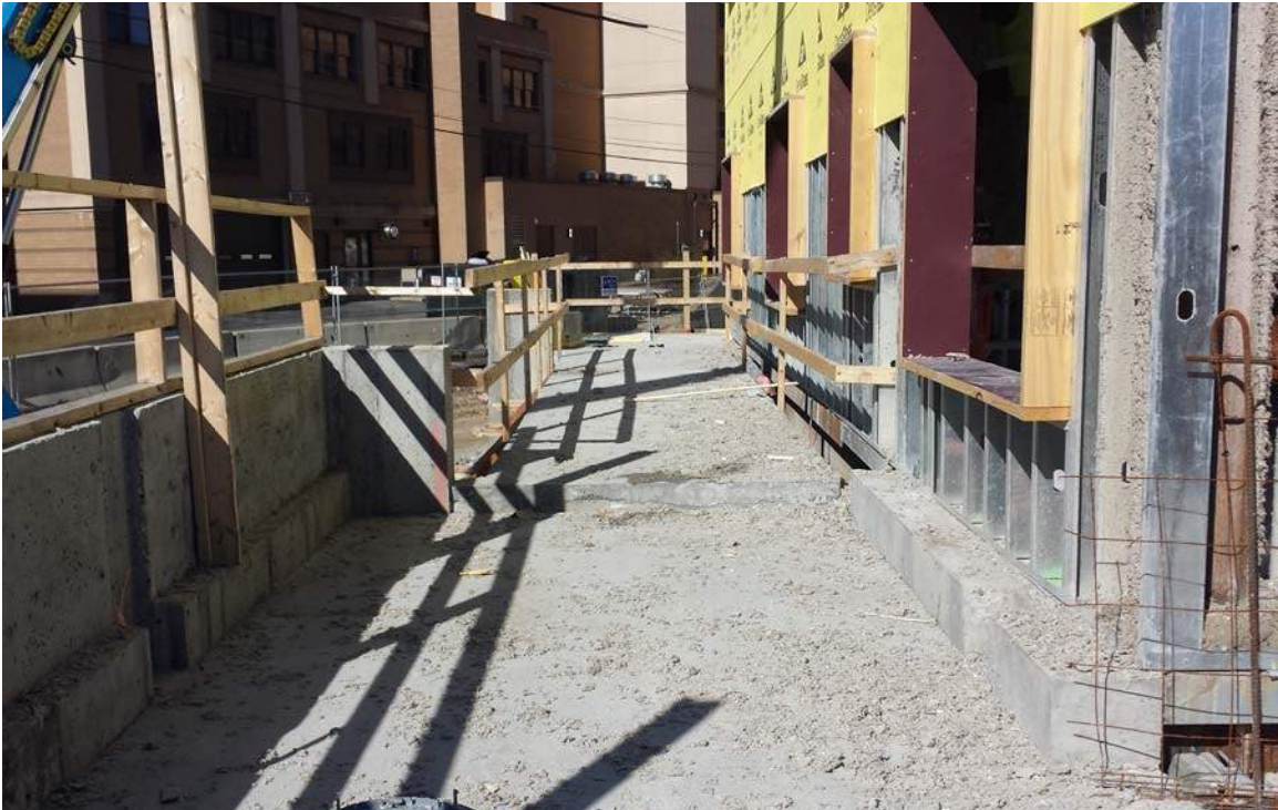
Terrace over garage entrance
