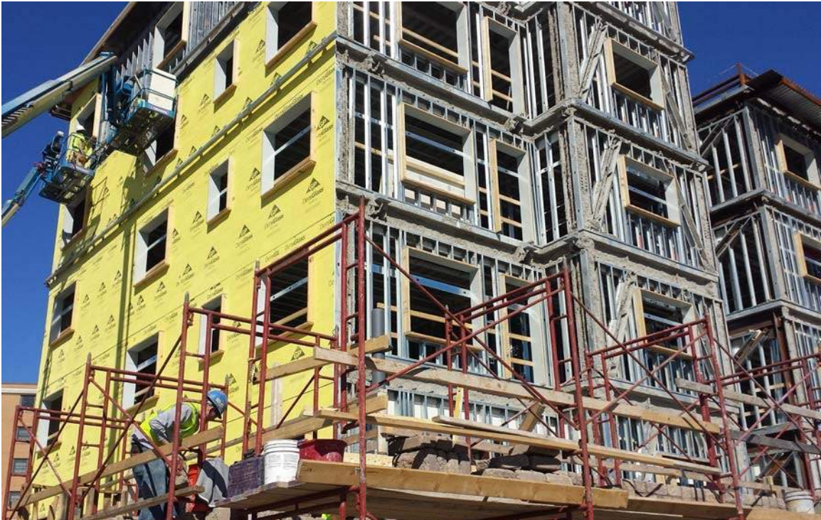
Tower east wing looking south west
