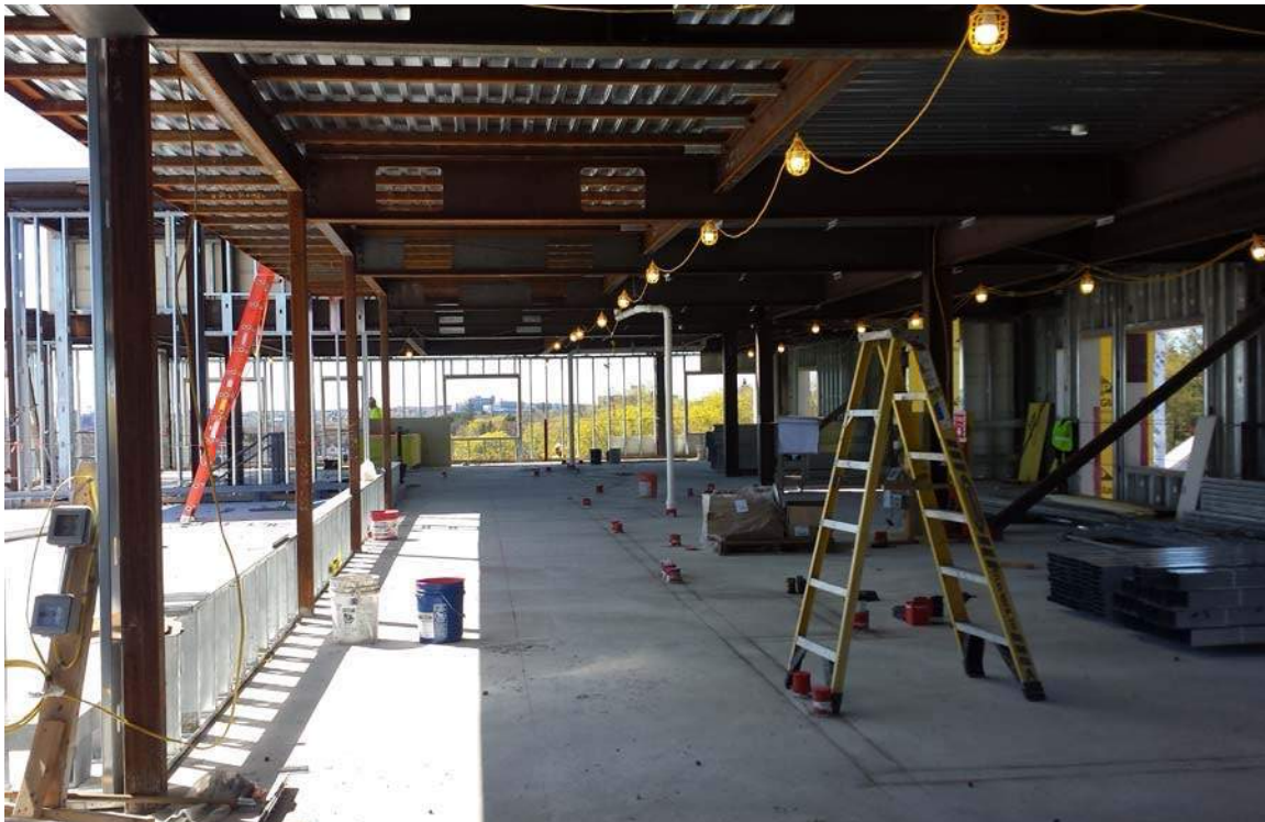
Level 5 of tower, east wing
