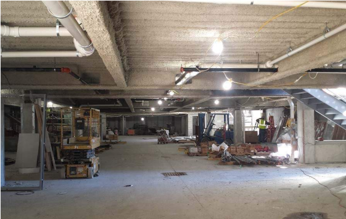
Garage level east wing
