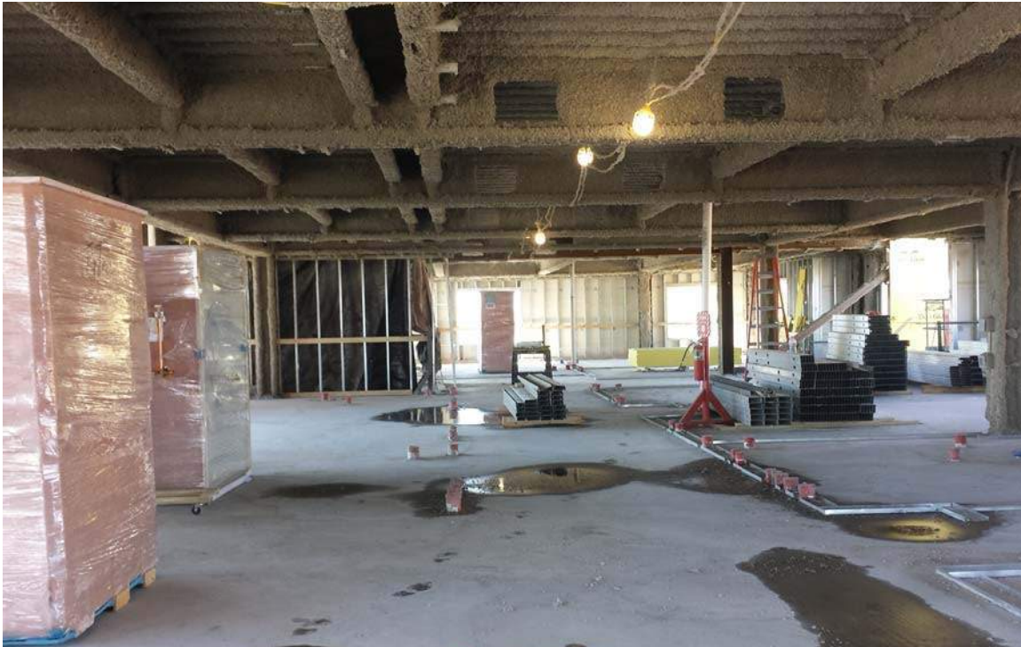
Level 4 of tower, east wing
