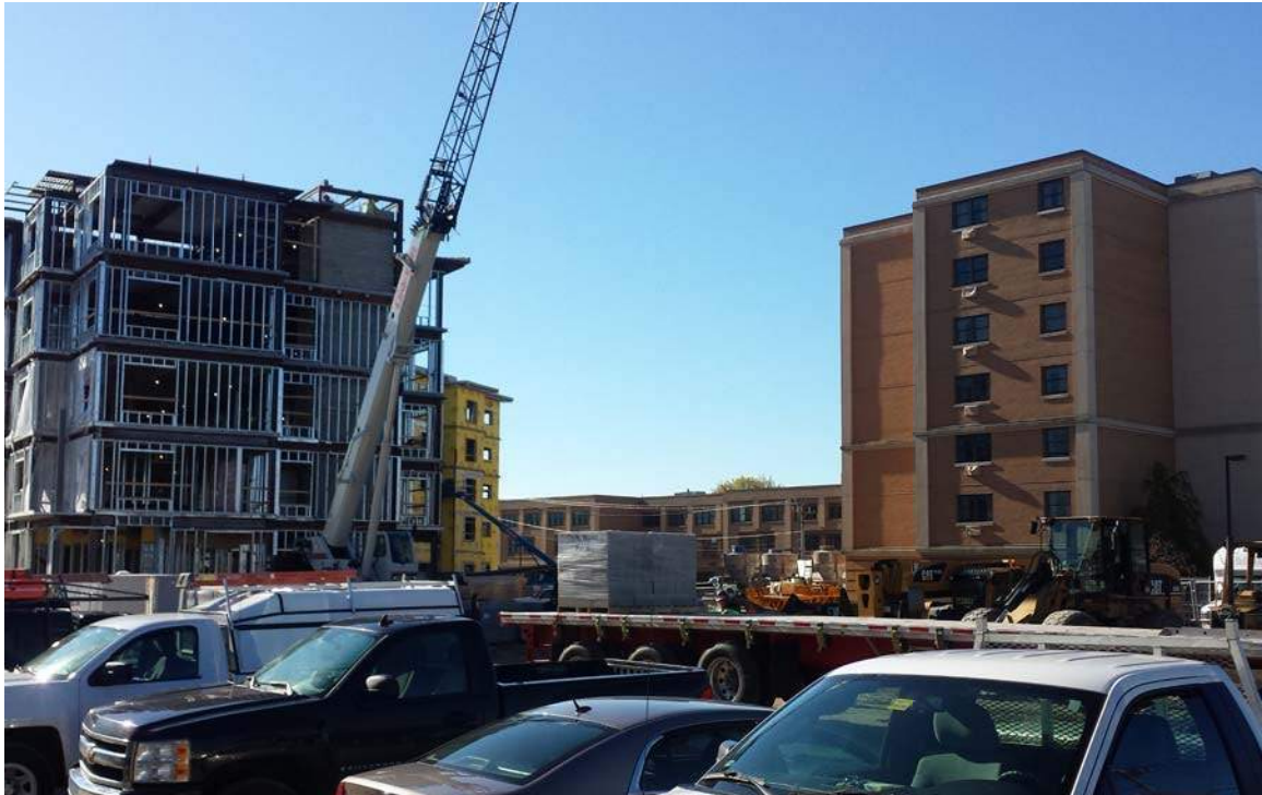
New Tower Construction looking southeast
