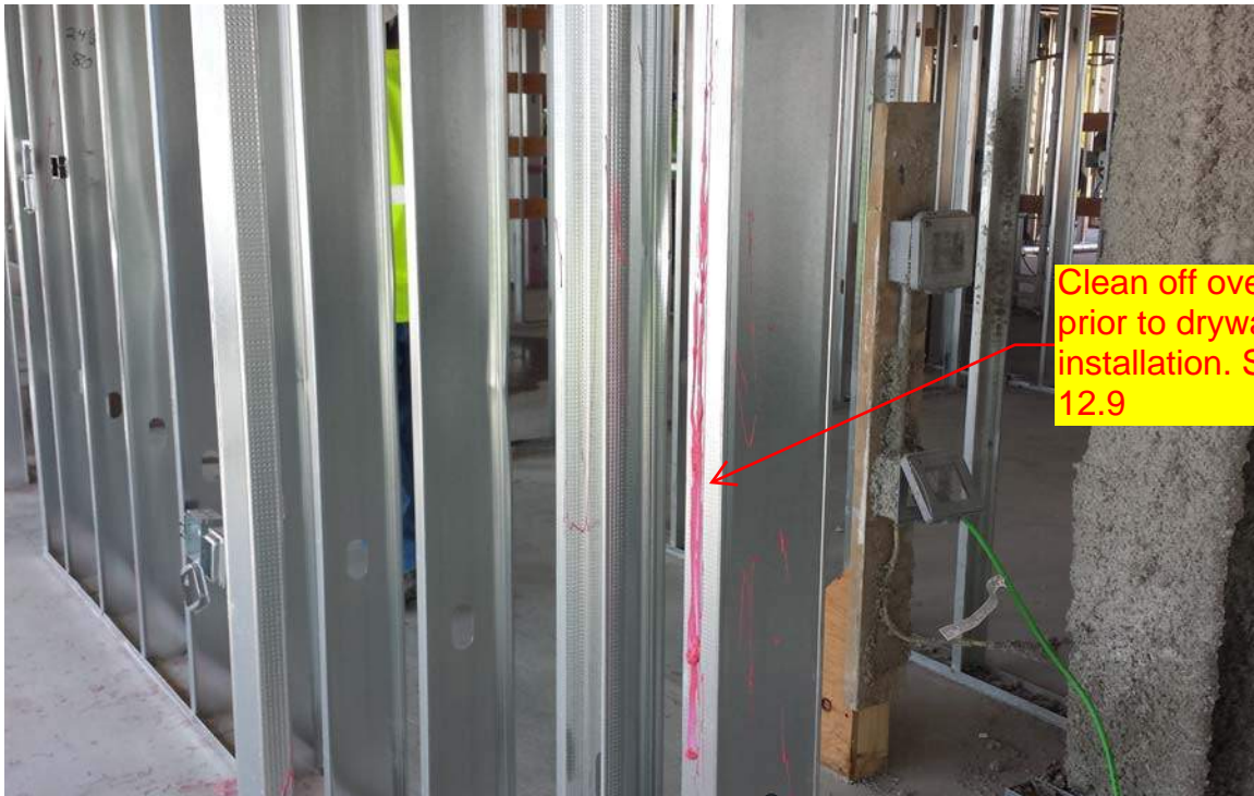
Level 1 of tower, west wing, administrative area
