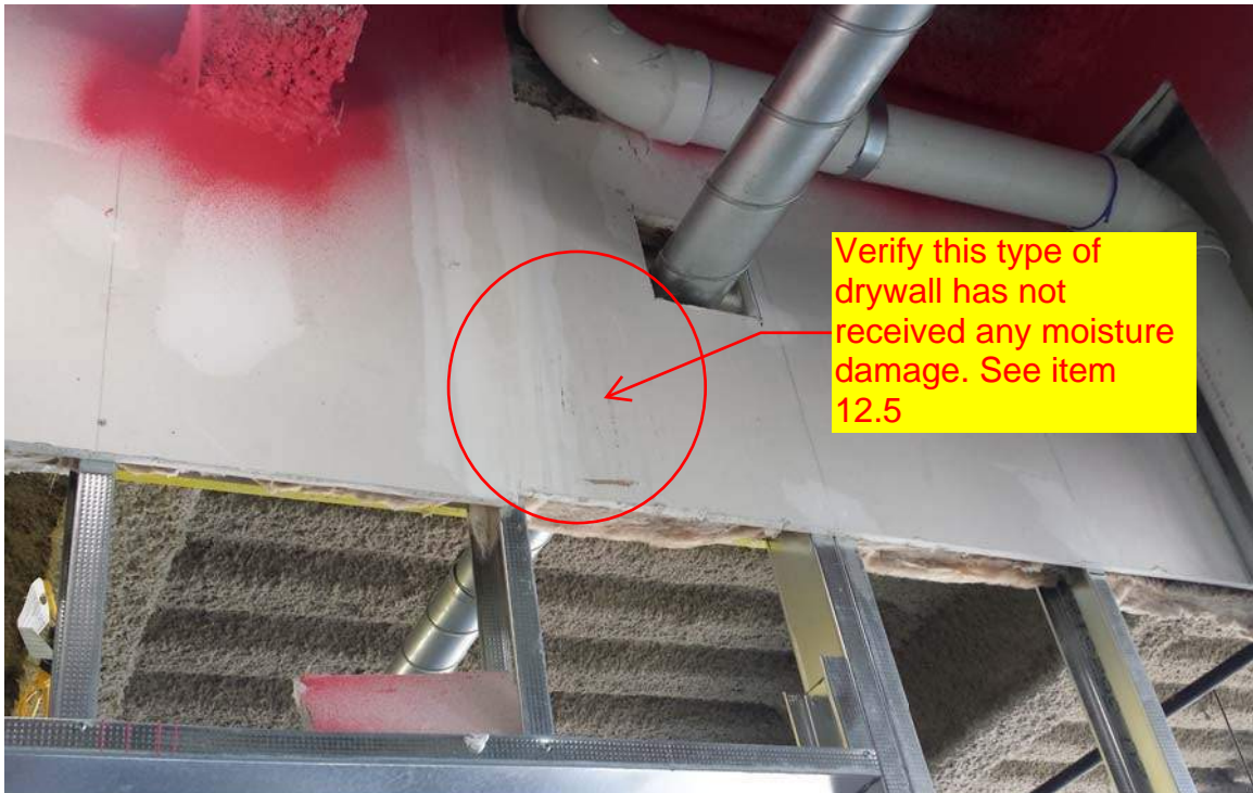
Level 1 of tower, west wing, administrative area
