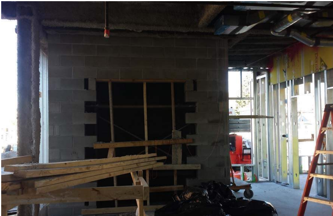
Level 1 of tower, west wing, Elevator A
