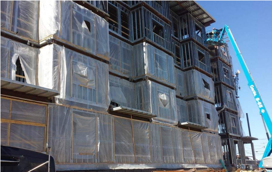
tower west wing looking west
