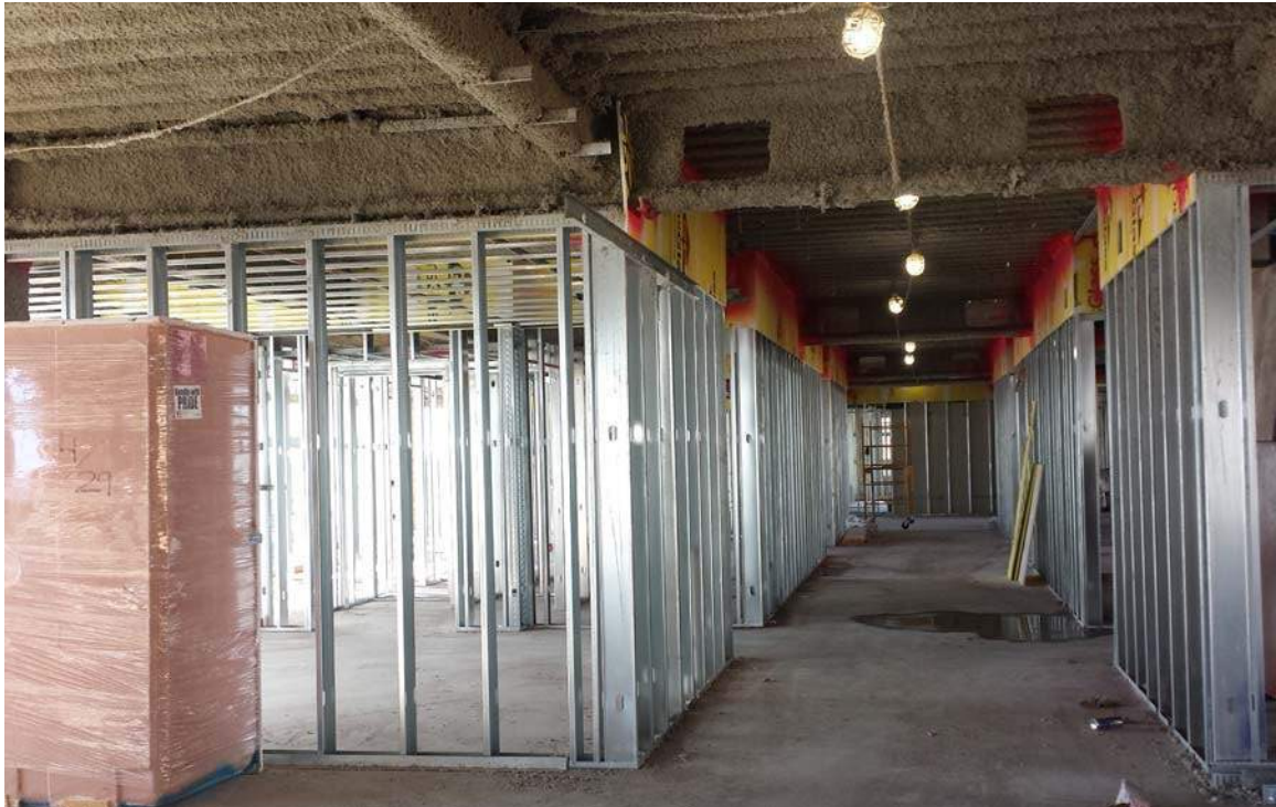
Level 3 of tower, east wing
