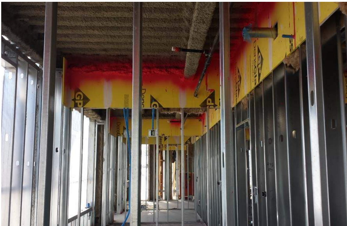
Level 1 of tower, west wing, administrative area
