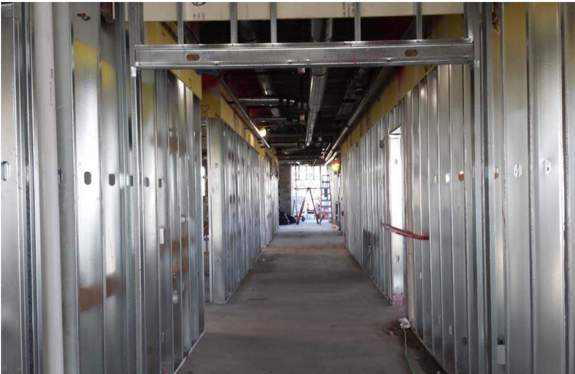
Level 1 of tower, looking west
