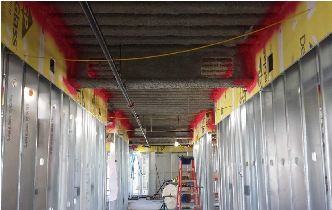
Level 2 of tower, east wing
