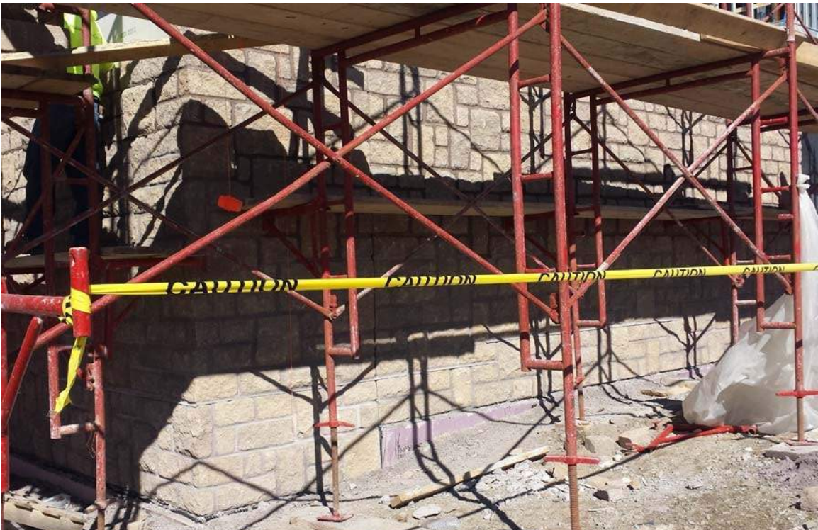
Masonry at Forest Ave Terrace/Electrical room exterior
