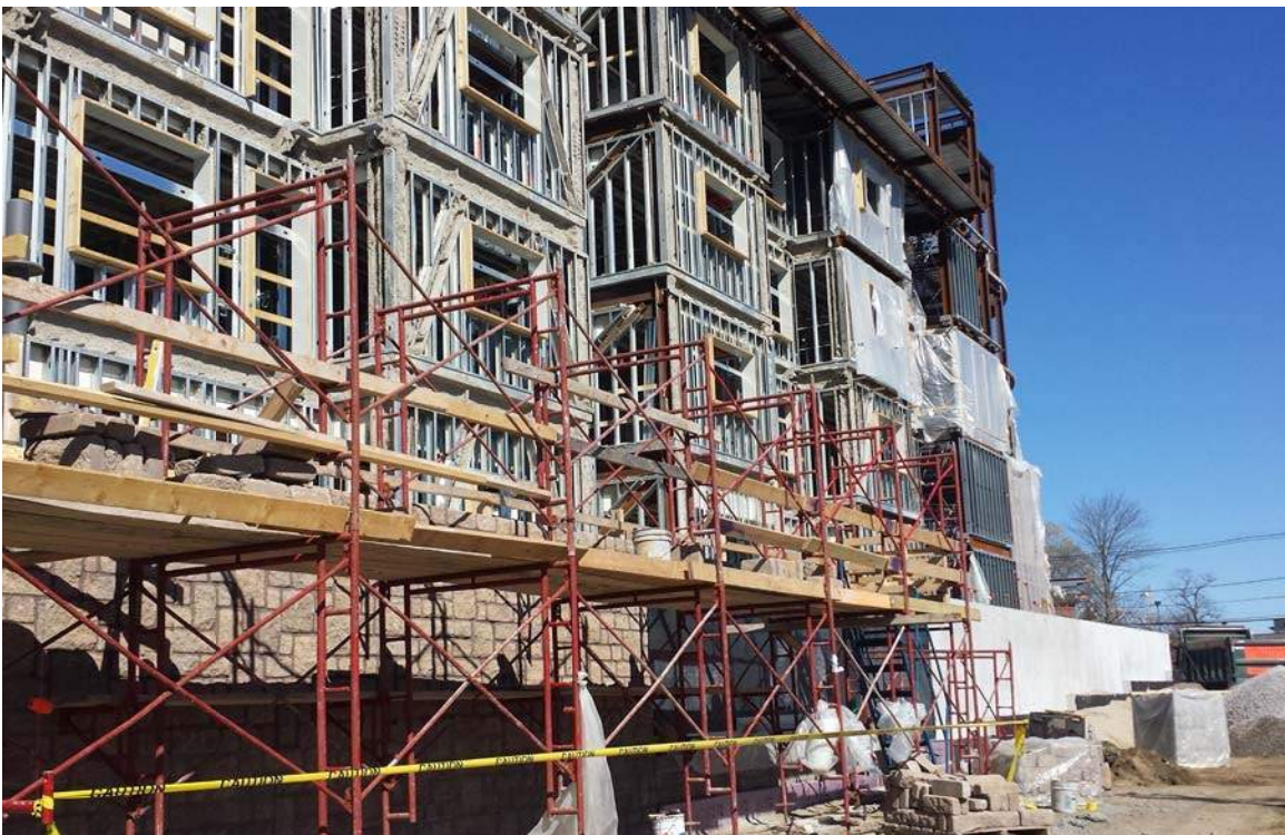
Tower east wing looking north
