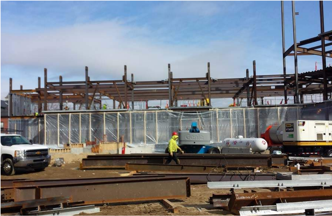
West Wing from courtyard side
