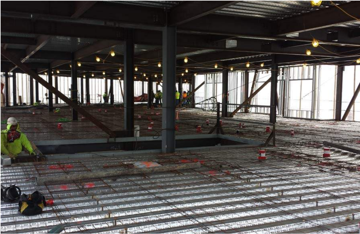
Level 1 Steel decking and reinforcement.
