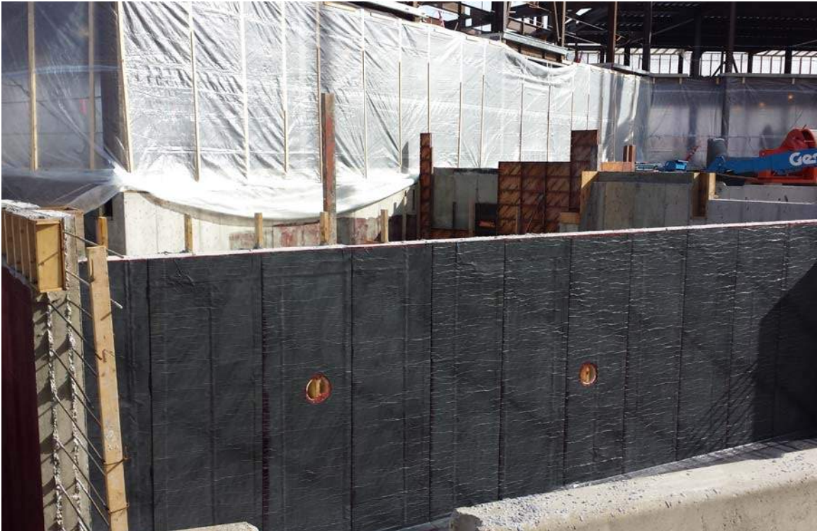
Boiler Room foundation walls
