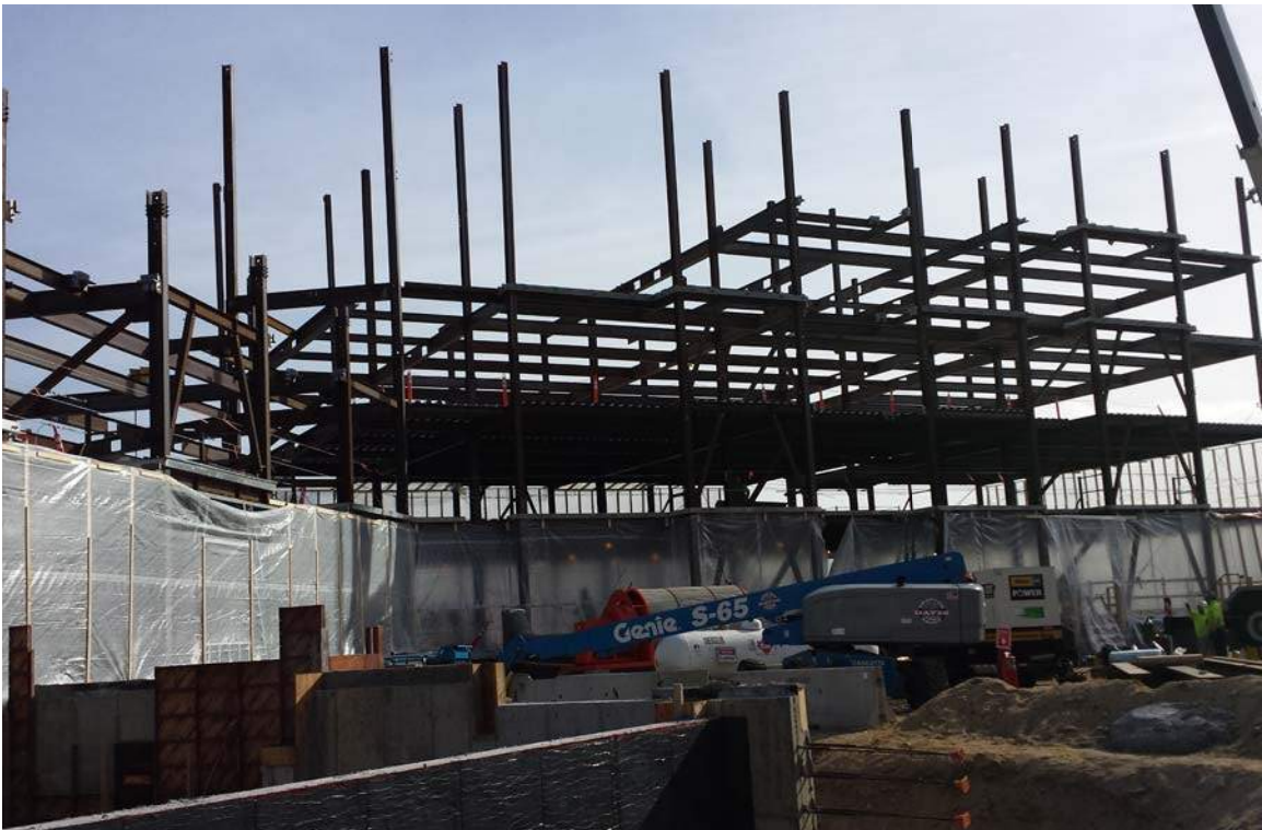
East Wing from courtyard side
