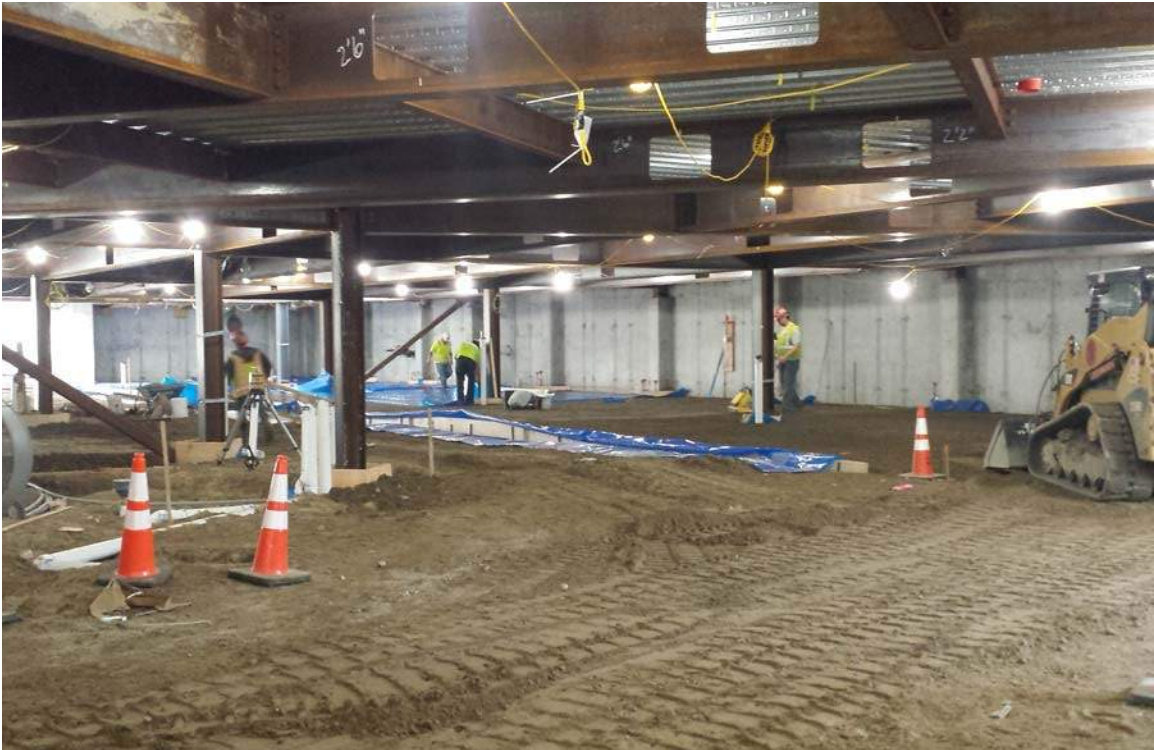
Garage Level concrete slab prep.
