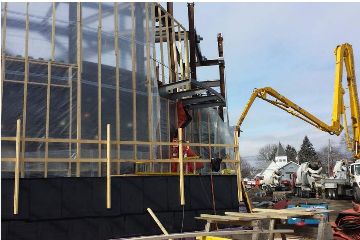
Tower knuckle at canopy from Forest Ave.
