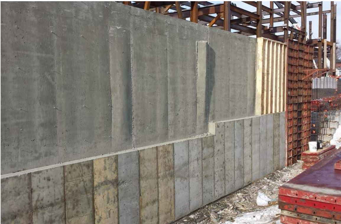
Exterior of electrical room, Forest Ave elevation (Reference Item 6.2)
