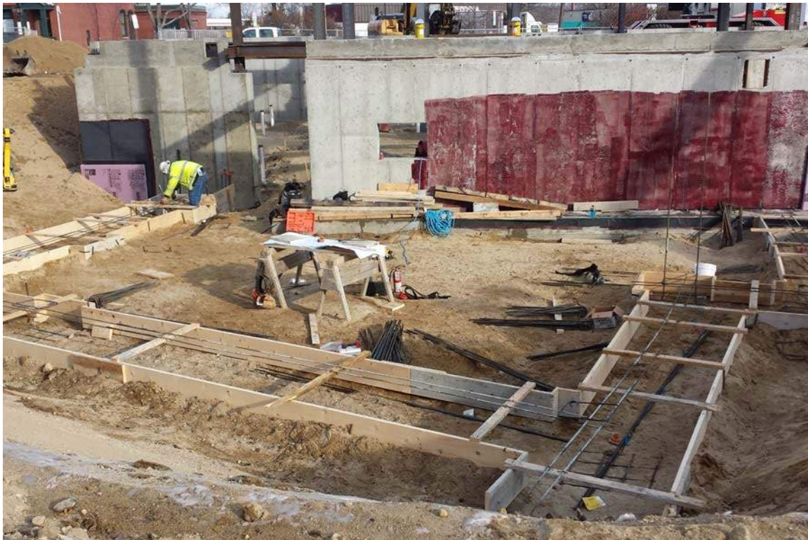
Boiler Room foundation footing formwork off of west wing garage
