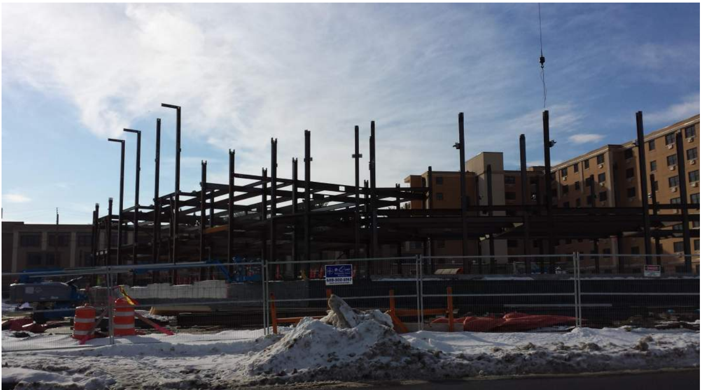
Tower from corner of Forest Ave and Arbor Street
