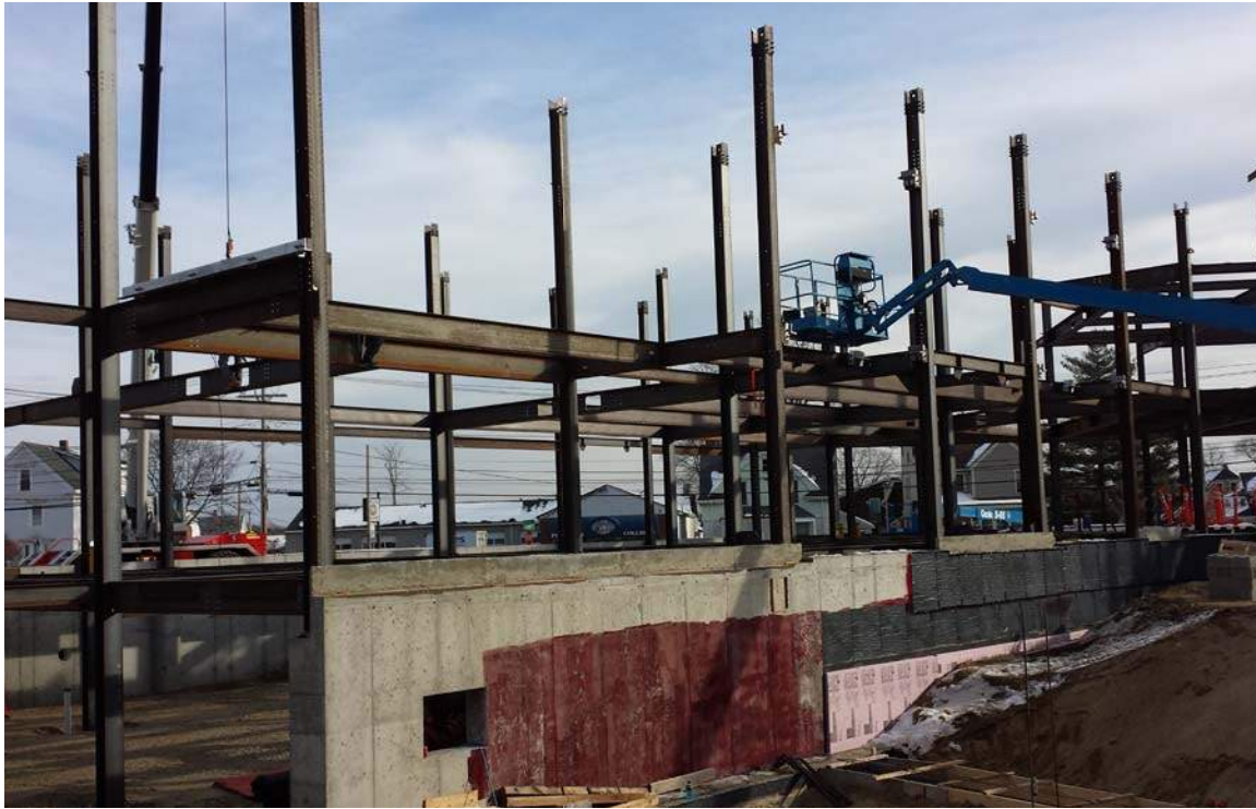
Steel progression at west wing, tower
