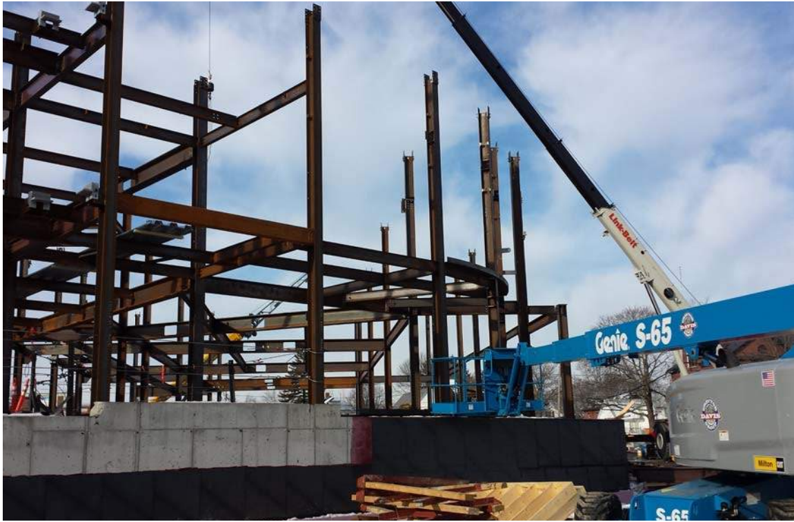
Tower Steel progression at building knuckle from Forest Ave.
