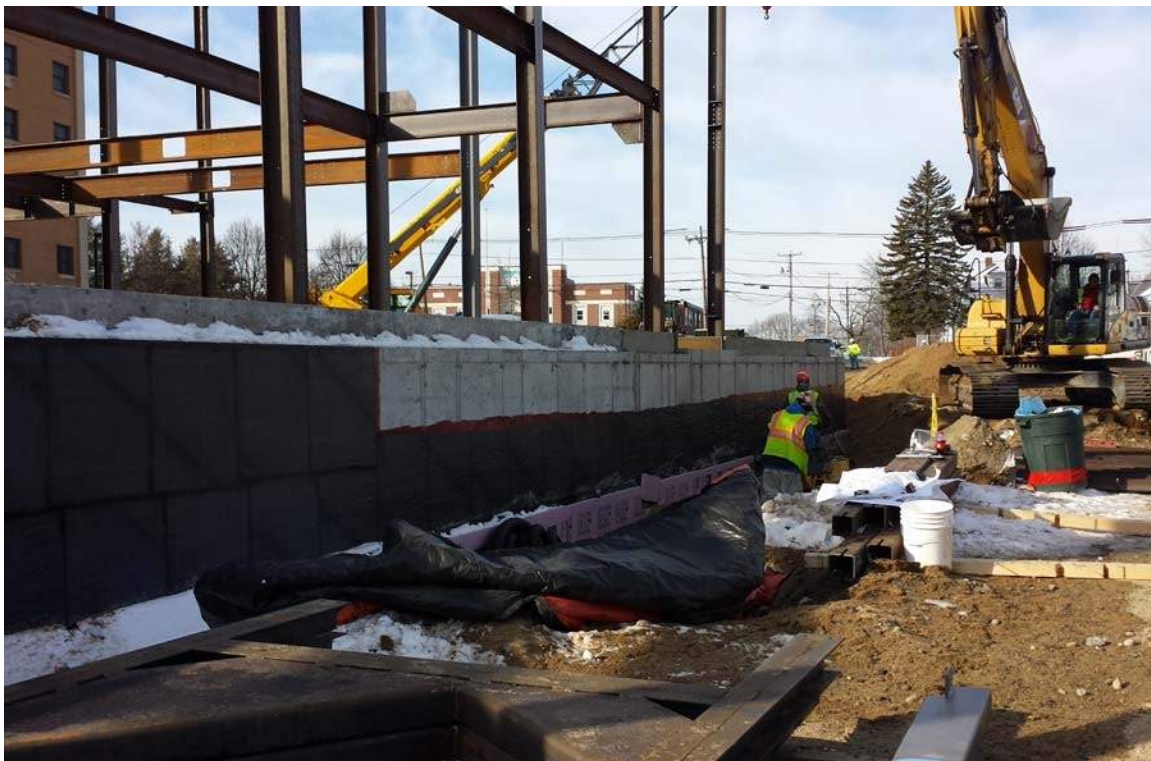
Foundation and waterproofing progress along Arbor Street elevation
