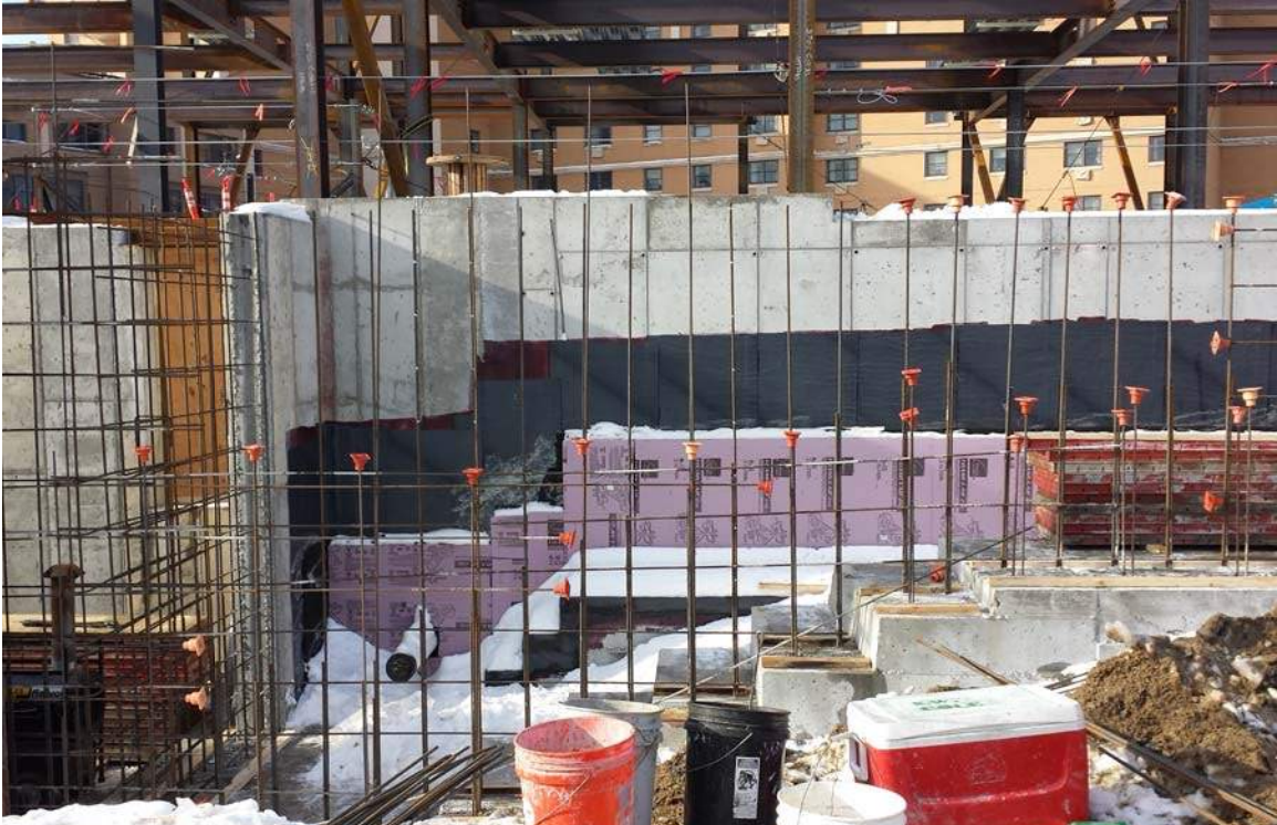
Terrace wall reinforcing and foundation wall waterproofing, Forest Ave.
