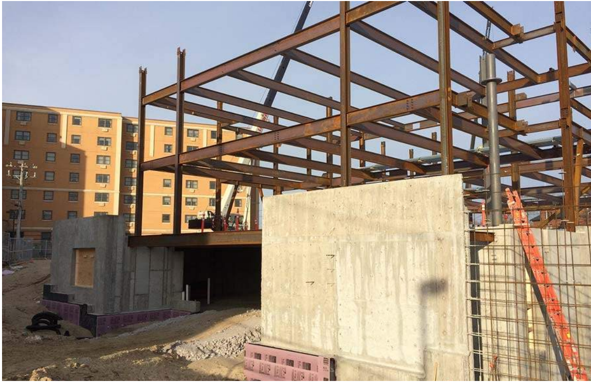
Southeast building elevation & garage entrance
