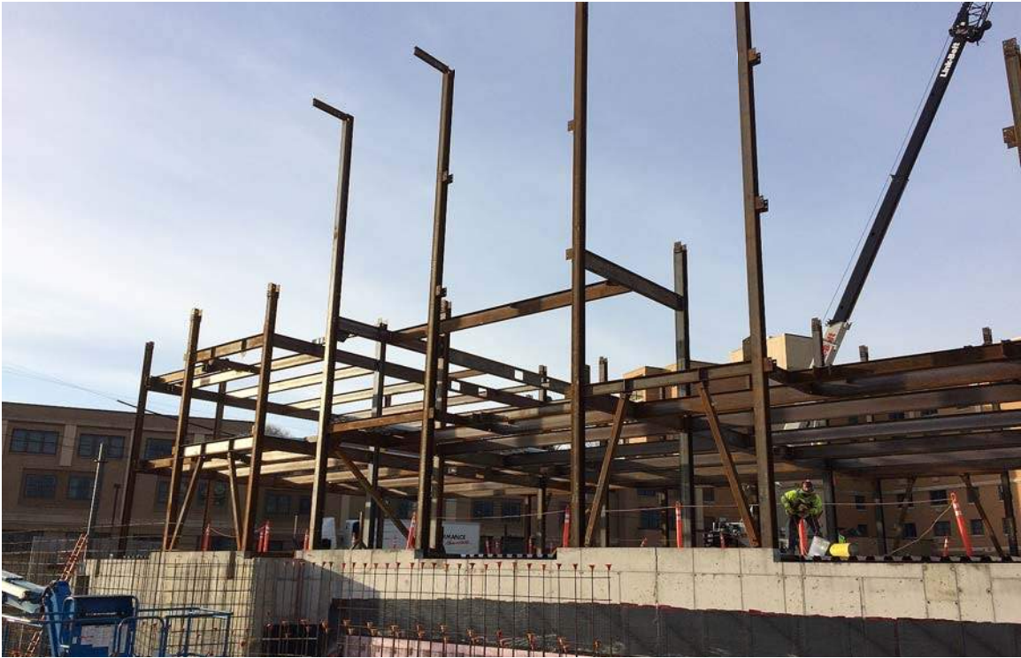
Steel progress as viewed from Forest Ave.
