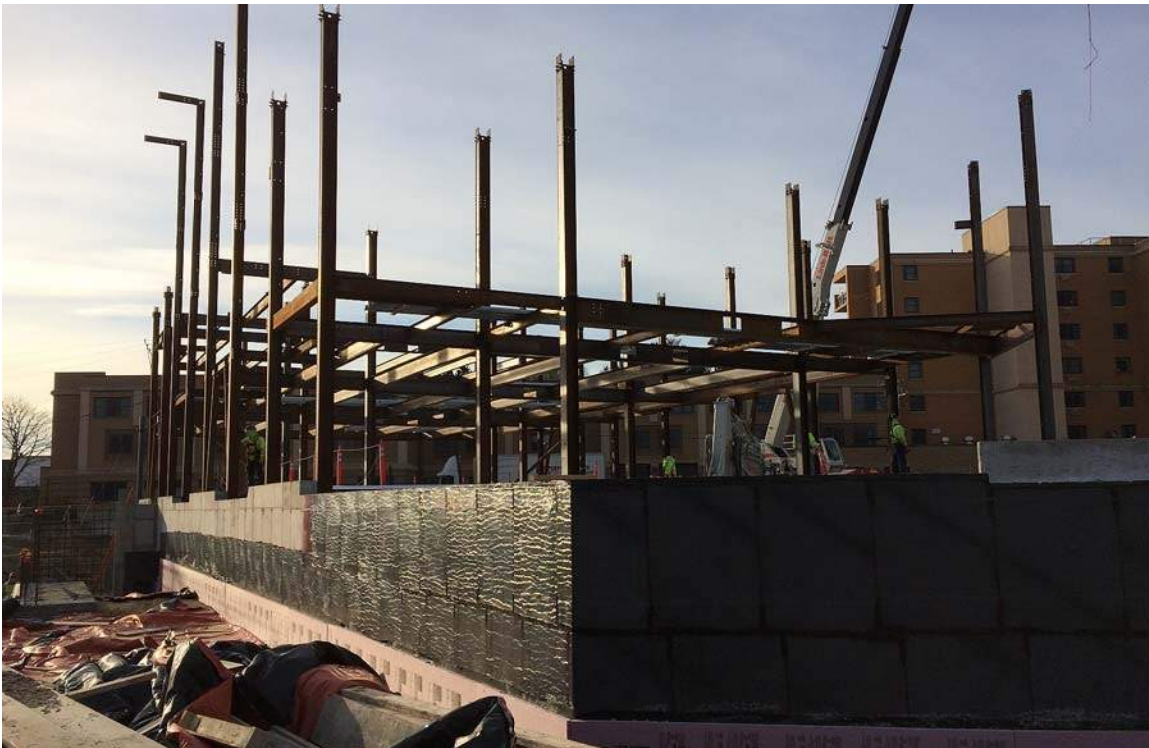
Steel progression at east wing, tower.
