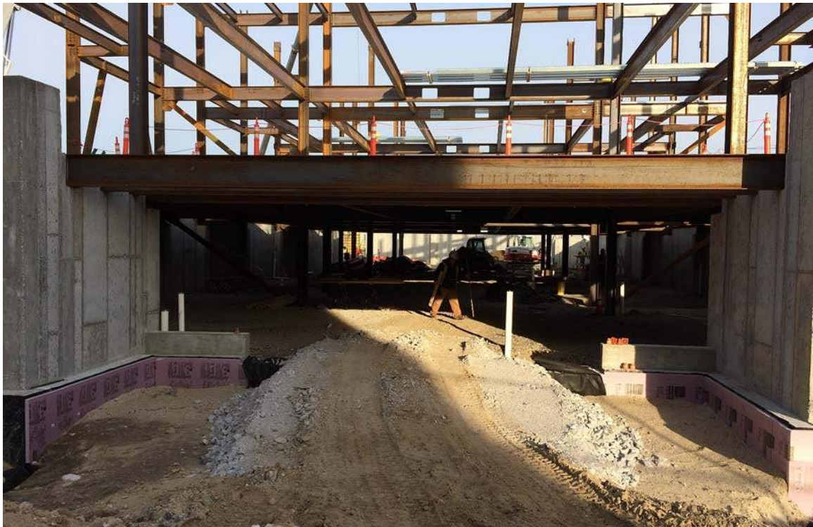
Garage entrance/ garage level
