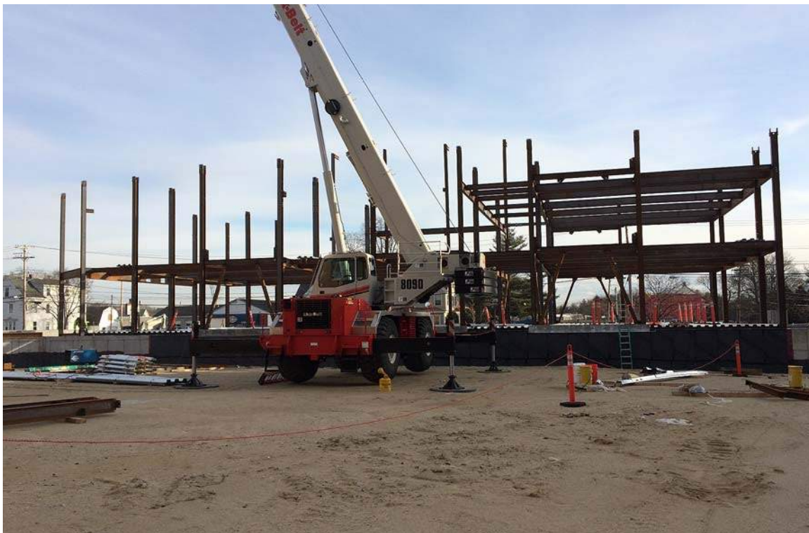
East wing of tower as viewed from courtyard-side
