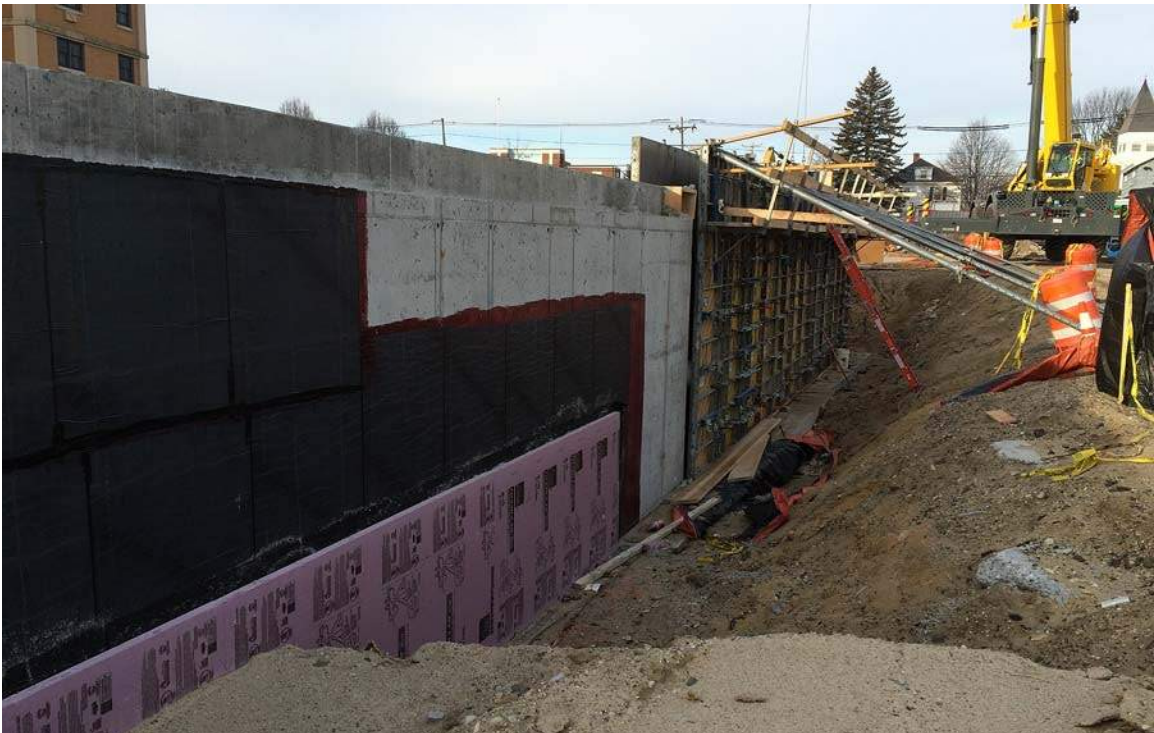
Foundation progress along Arbor Street elevation
