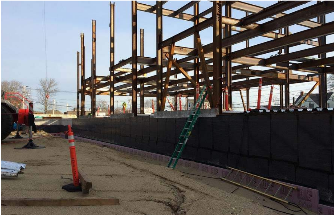
Foundation waterproofing, courtyard-side
