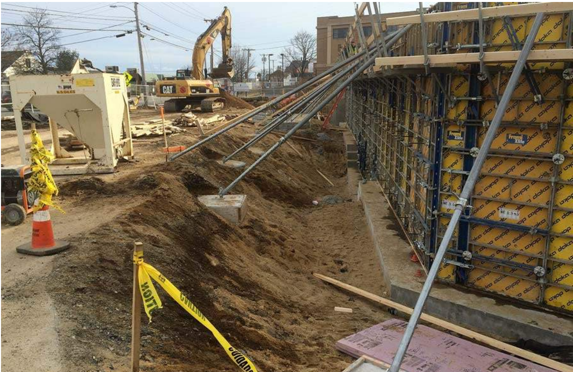
Wall formwork along E-Line
