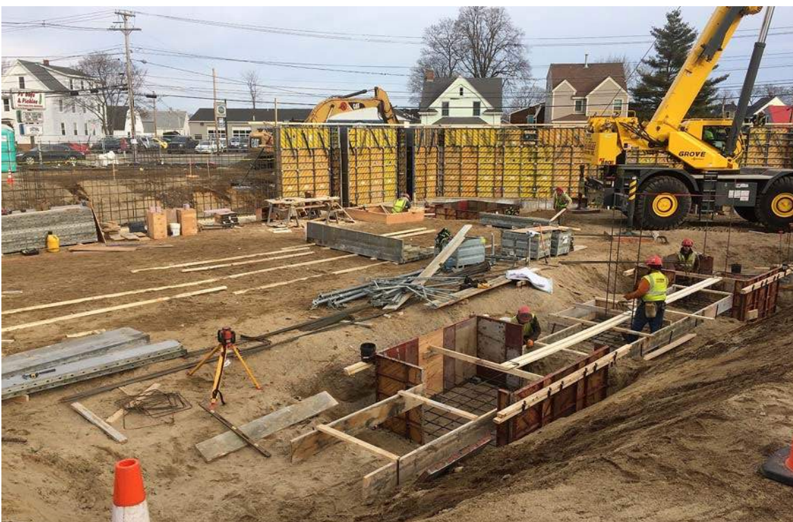
Progress of foundations along west wing of tower.
