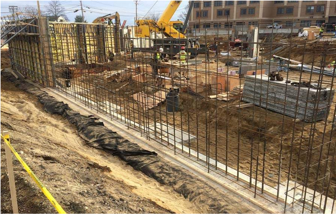
CIP footing and wall reinforcement along A-Line
