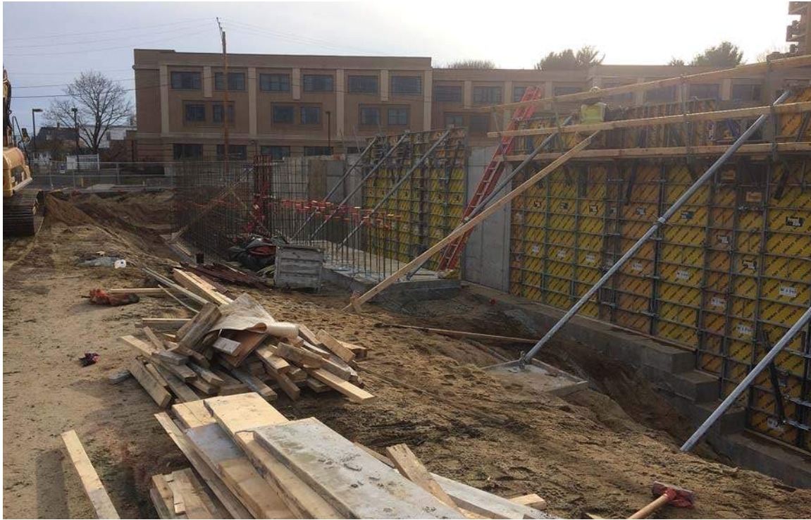
Wall formwork along E-Line
