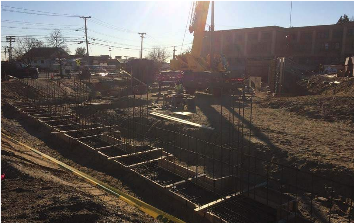
Footing formwork and reinforcing along A-Line
