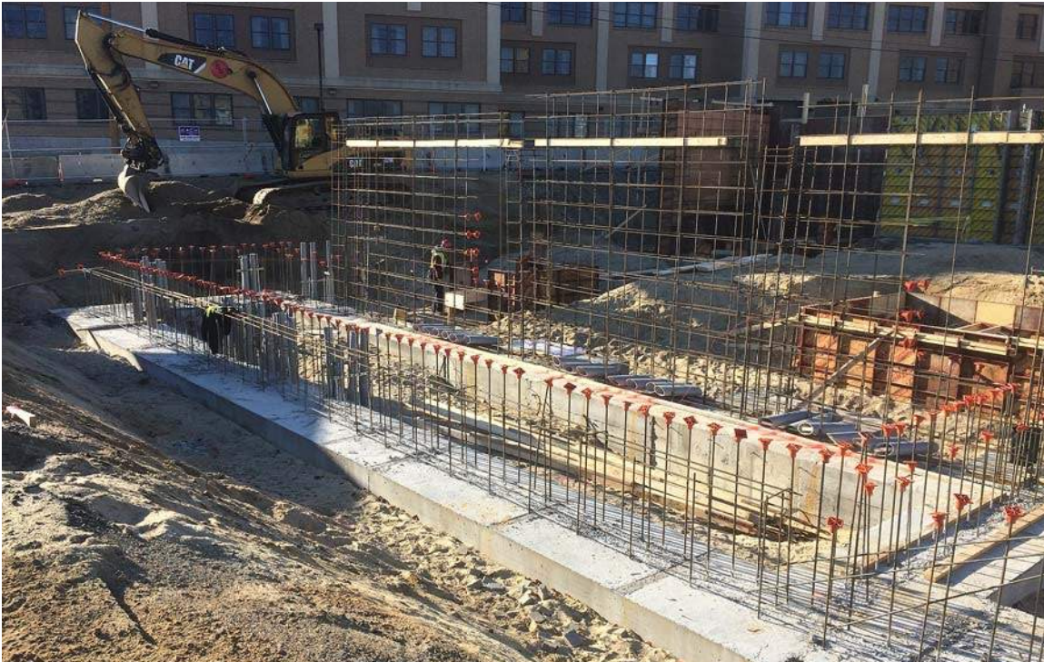
Foundations along E-Line near Main electrical room G013
