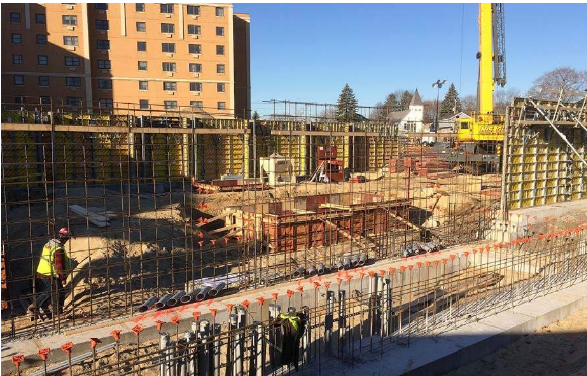
Wall formwork progress along H-Line (courtyard side)
