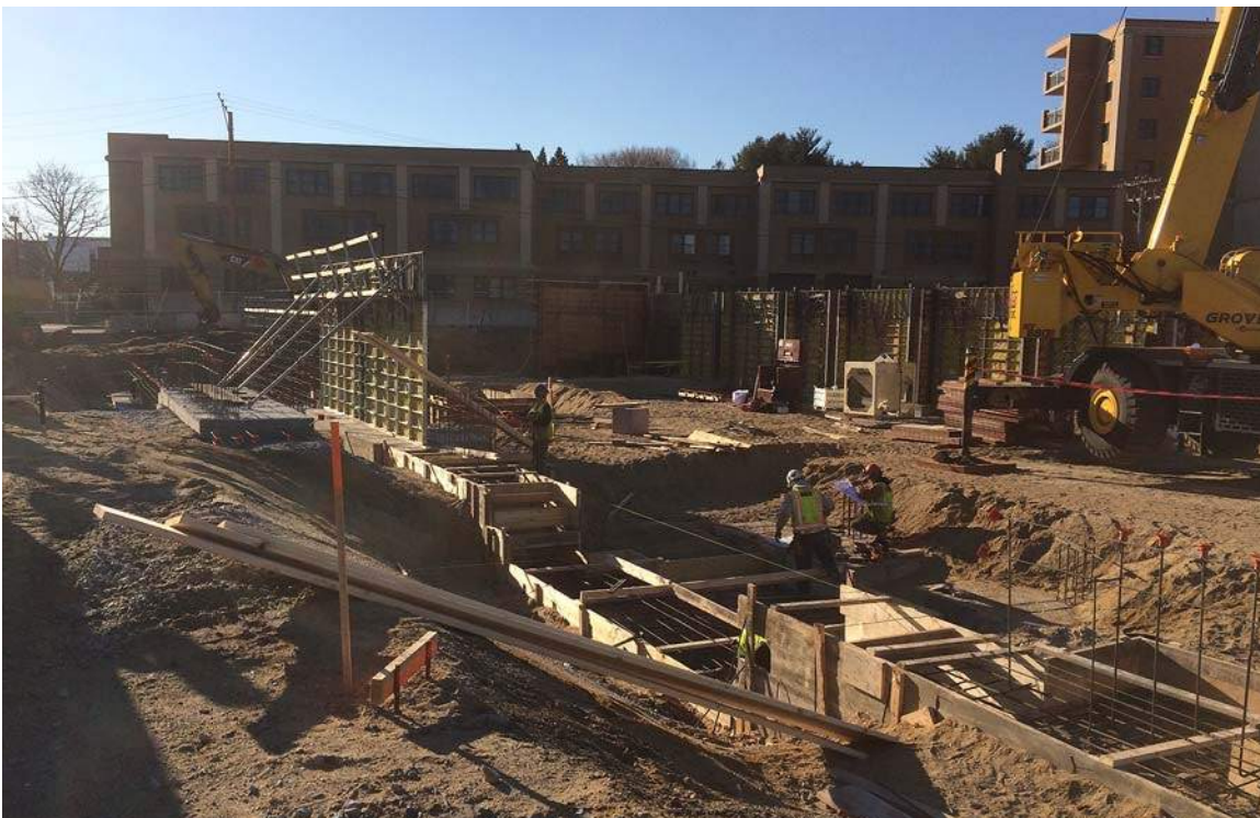
Foundations along E-Line (elevator B shaft is center of view)
