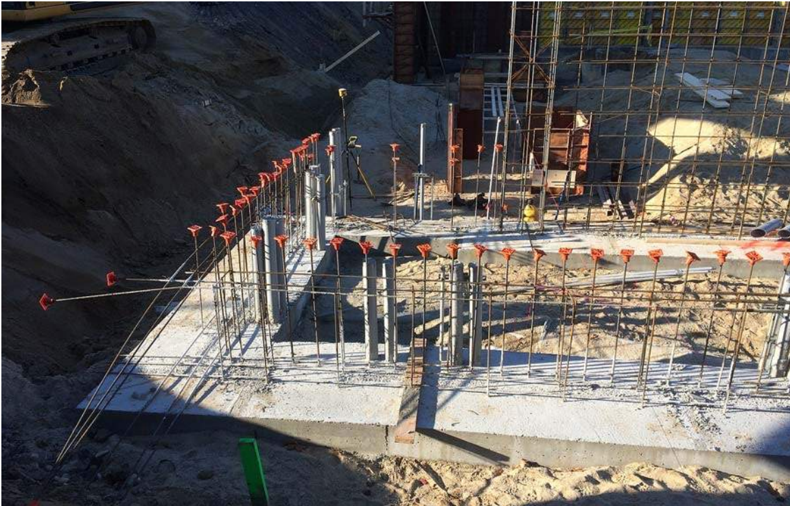
Footing placement at Main Electrical Room G013
