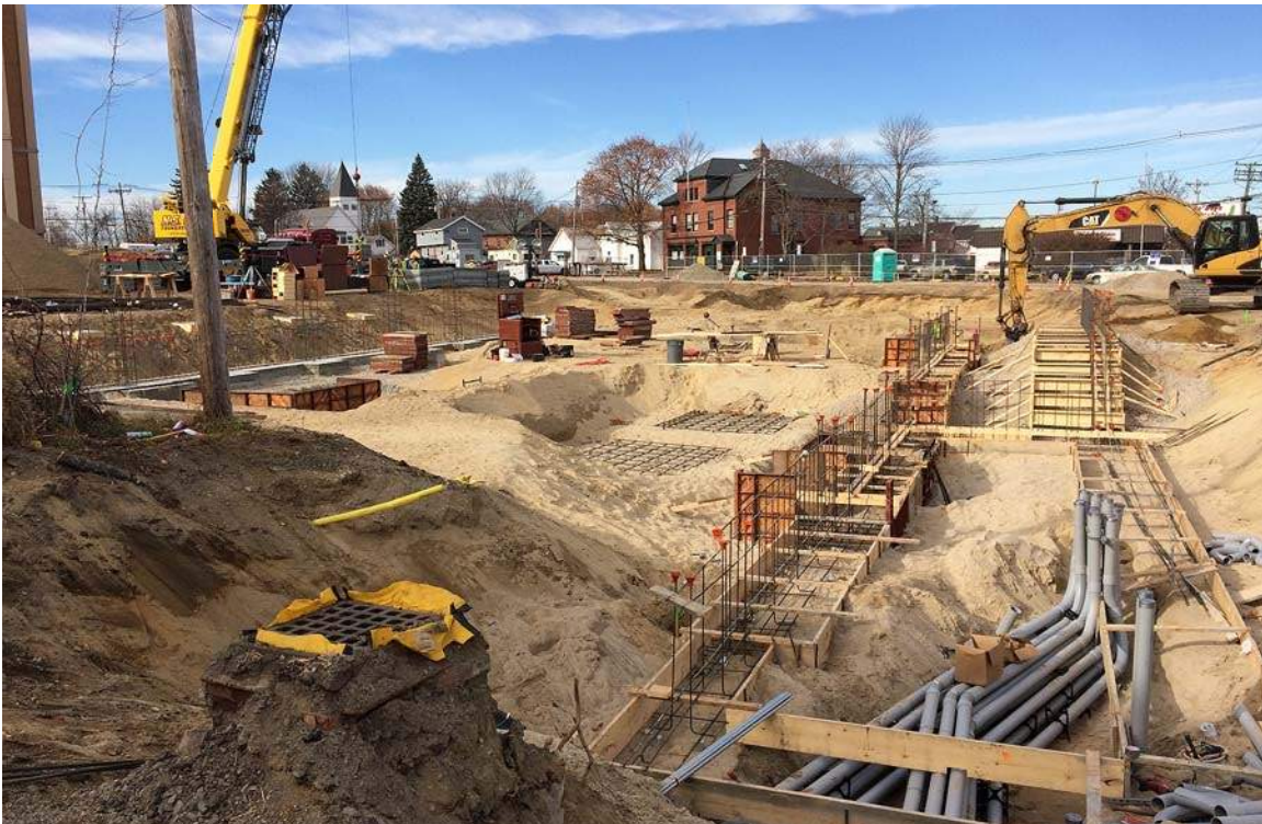
View from existing service drive looking north - northwest
