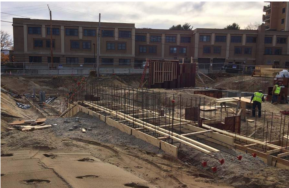
Forest Ave terrace footings
