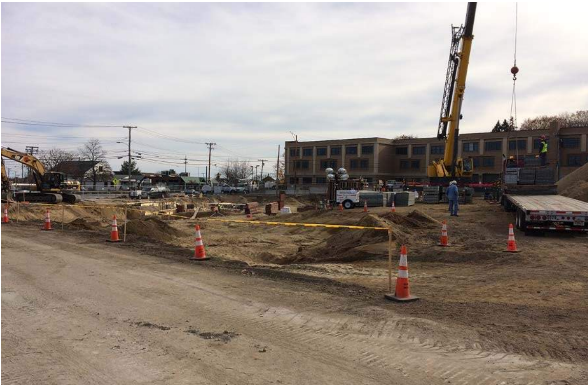
Tower construction site (from Arbor Street looking south)
