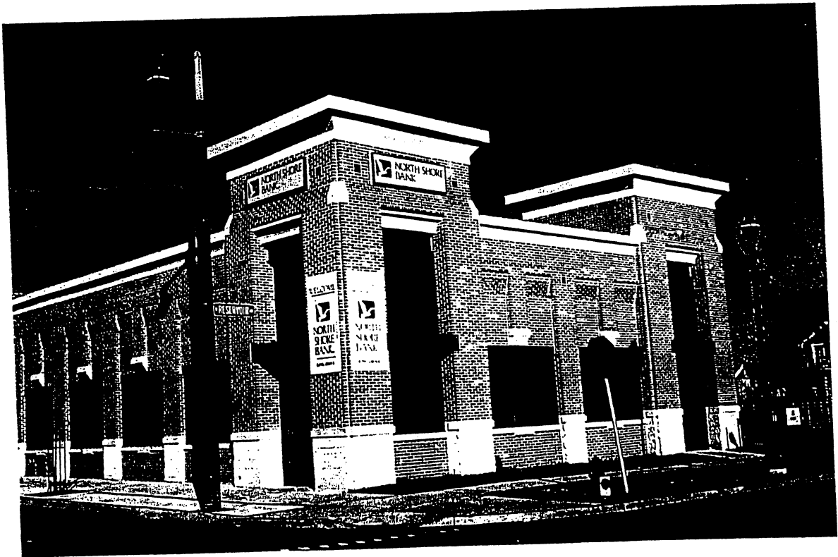
North Shore Bank, Architect: Eppstein Keller Uhen - Contractor: Hopkins & Hopkins Masonry
