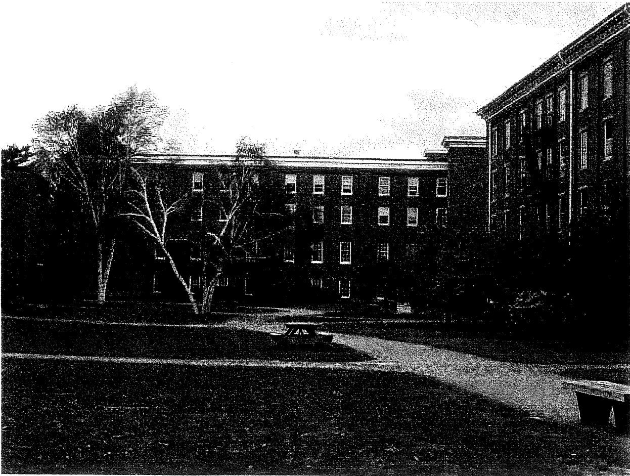
B. view of Proctor Hall (4-story building at rear of quadrangle) where proposed Lecture Hall will be constructed
