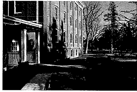
Goddard Hall renovations were completed in late 2011, making this historic building the administrative home for the College of Dental Medicine.
