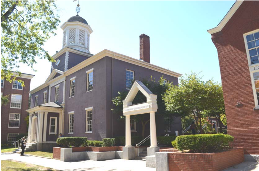
Entrance to Courtyard shared with McArthur
