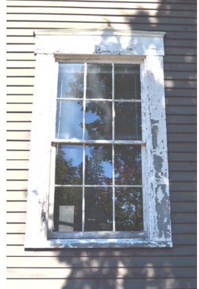
Typical Annex Window
