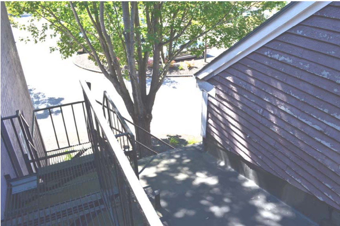
Roof top connection between Alumni and Annex
