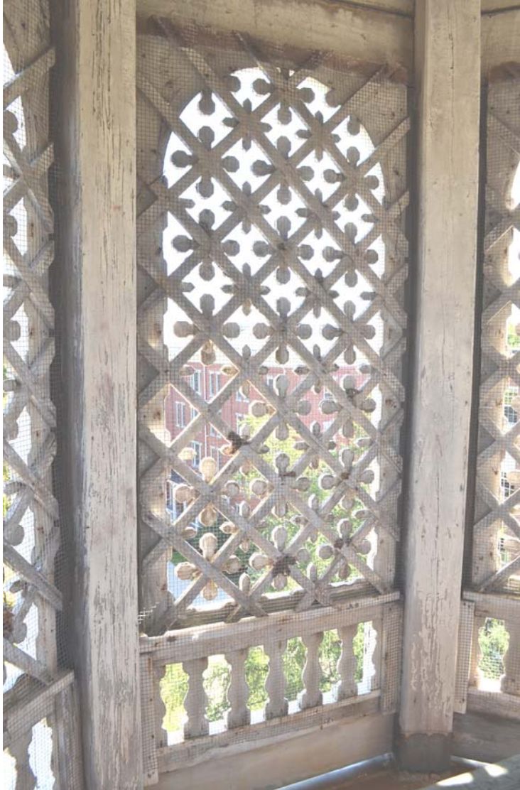
Lattice and Bell in the Cupola
