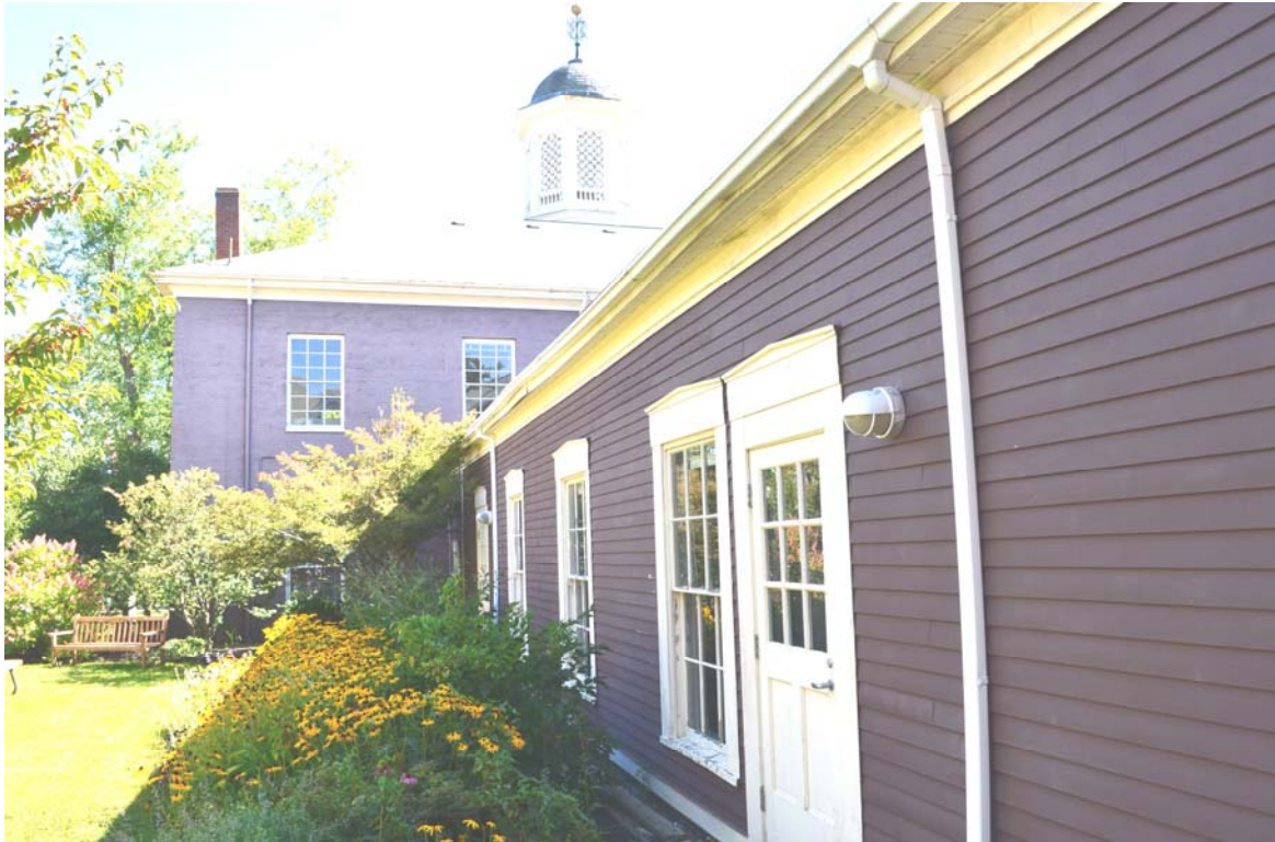
The Annex from the Courtyard
