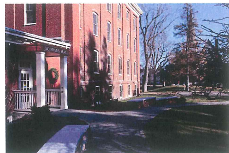
Goddard Hall renovations were completed in late 2011, making this historic building the administrative home for the College of Dental Medicine.
