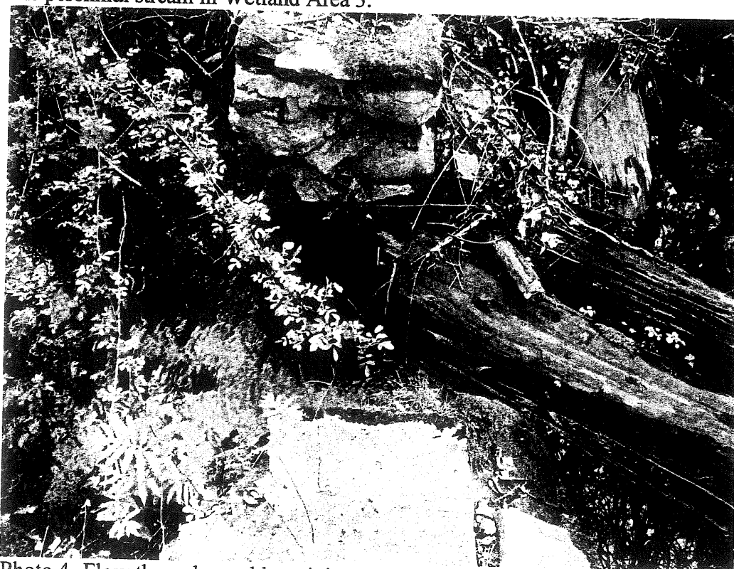
Photo 4- Flow through an old retaining wall at the outlet of Open Water Area 2. The wall constricts flow.
