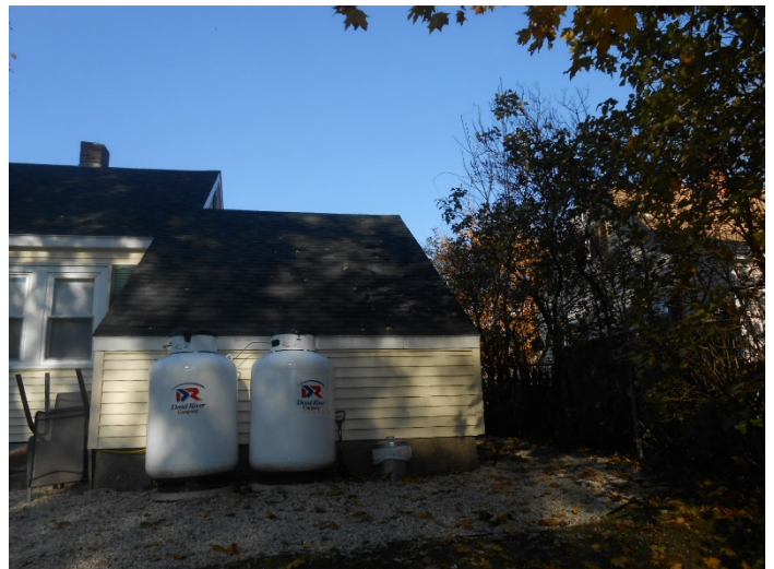
Back garage elevation
