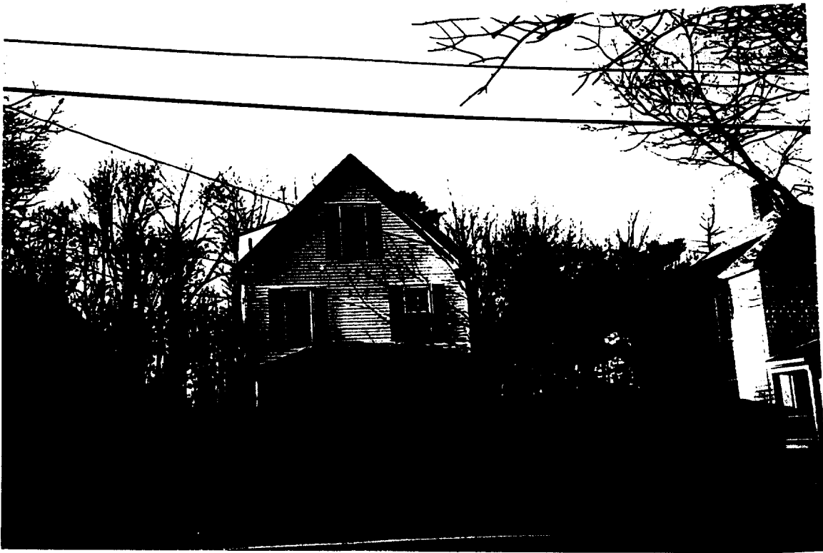
FRONT VIEW SHOWING NEIGHBORS (2)
