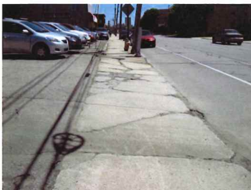
Northern curb cut and apron (to be closed)
