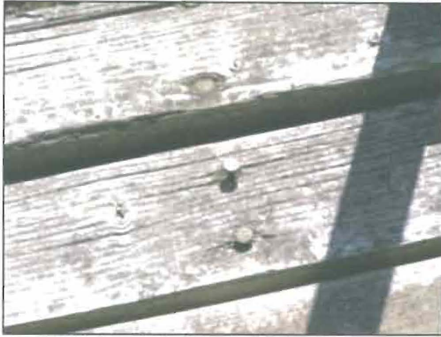
2.4 Picture 4 Replace decking on front porch
