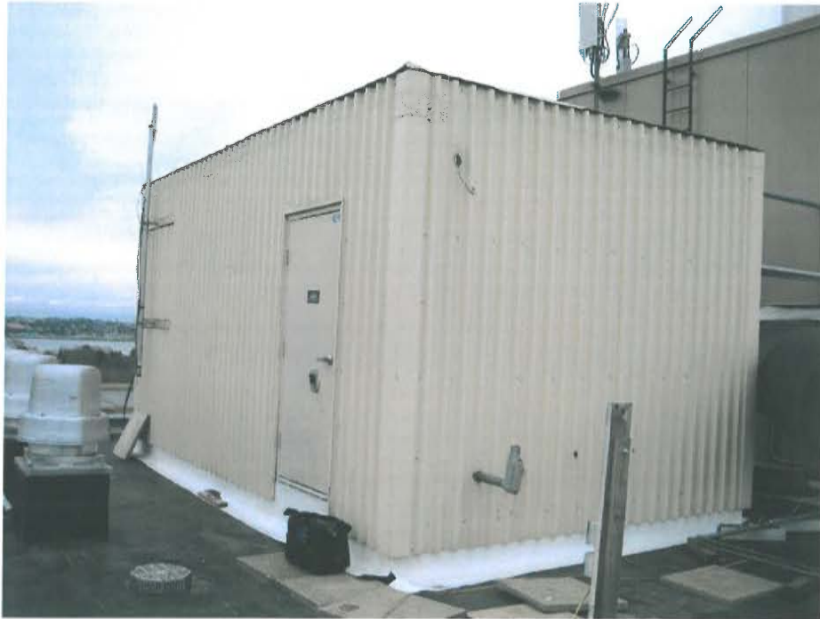
Photo 1: Sample photo illustrating the existing equipment shelter.
