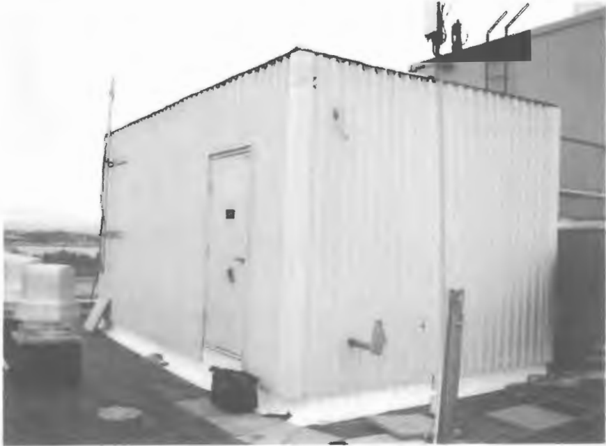
Photo 1: Sample photo illustrating the existing equipment shelter.
