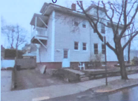
Driveway and terrace
