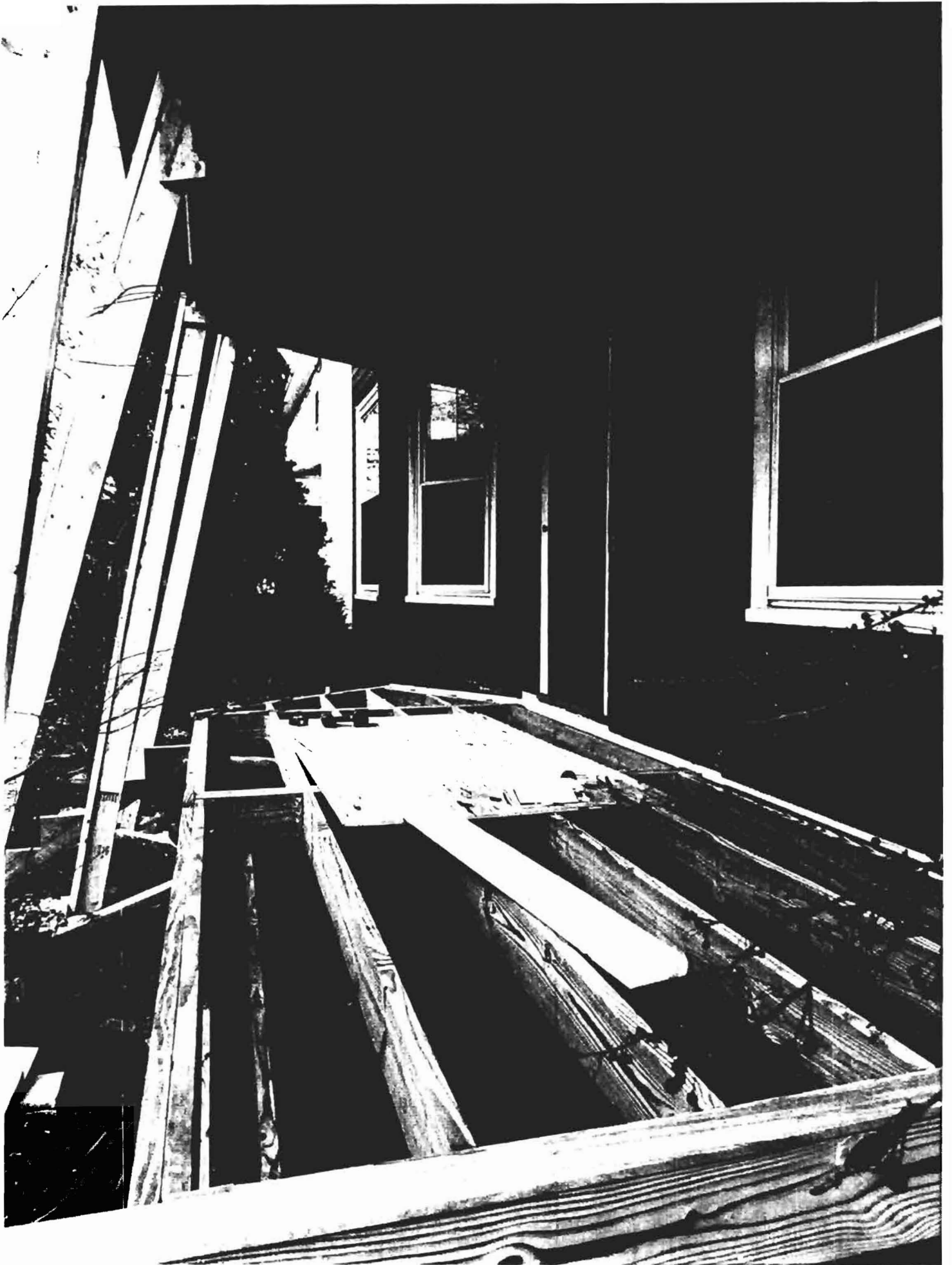
NEW 2x8 P.T. JOISTS IN PLACE.JPG
