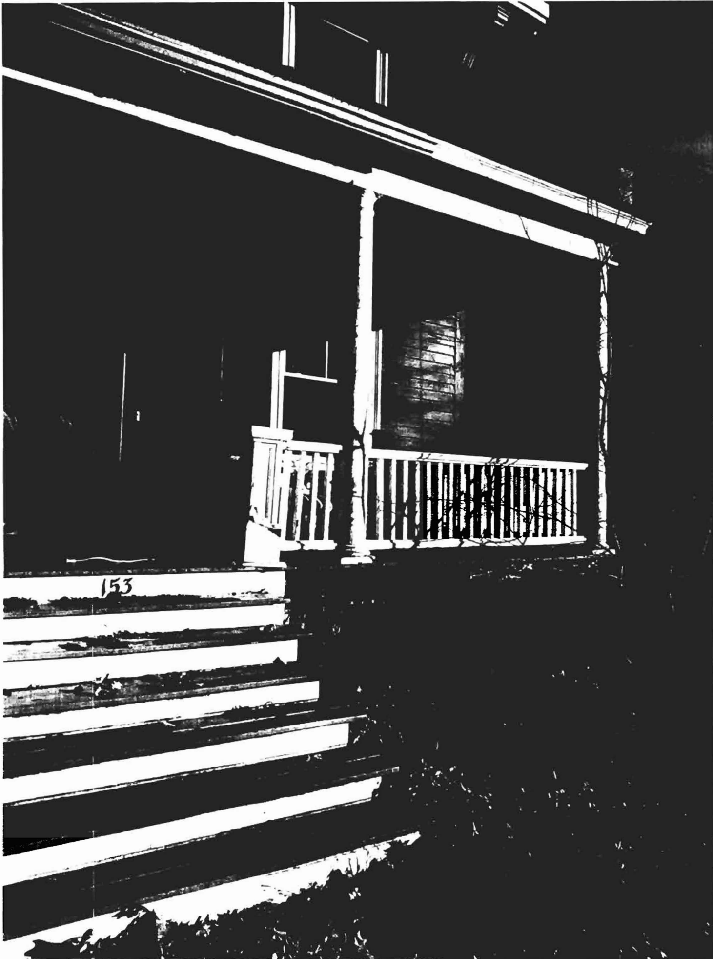
EXISTING PORCH WITH SKIRTING REMOVED.JPG
