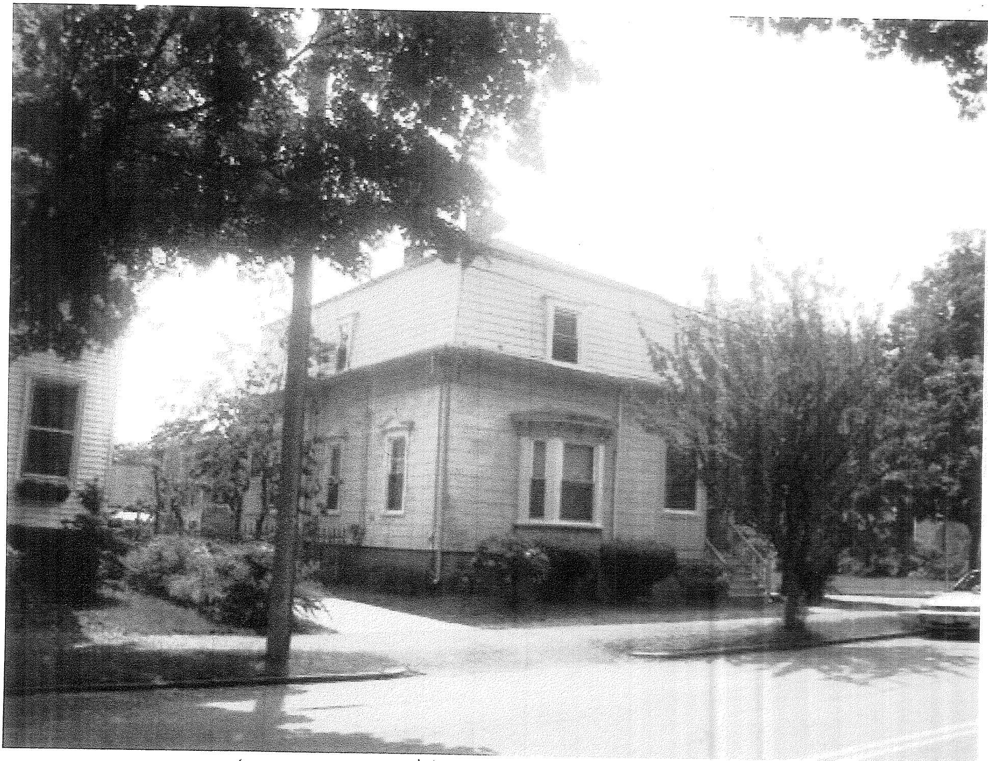
142 PLEASANT AVE SHOWING SIDE OF HOUSE WHERE NEW STAIR WILL BE.
