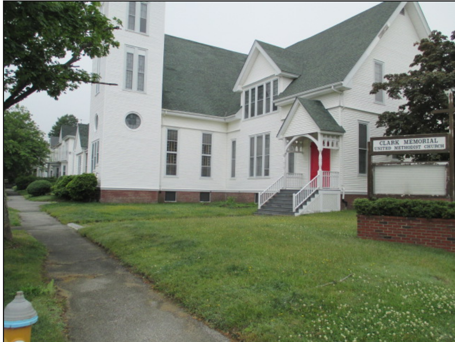
PHOTO 7 – Existing Church Building from Corner of Pleasant Avenue and Forest Avenue
