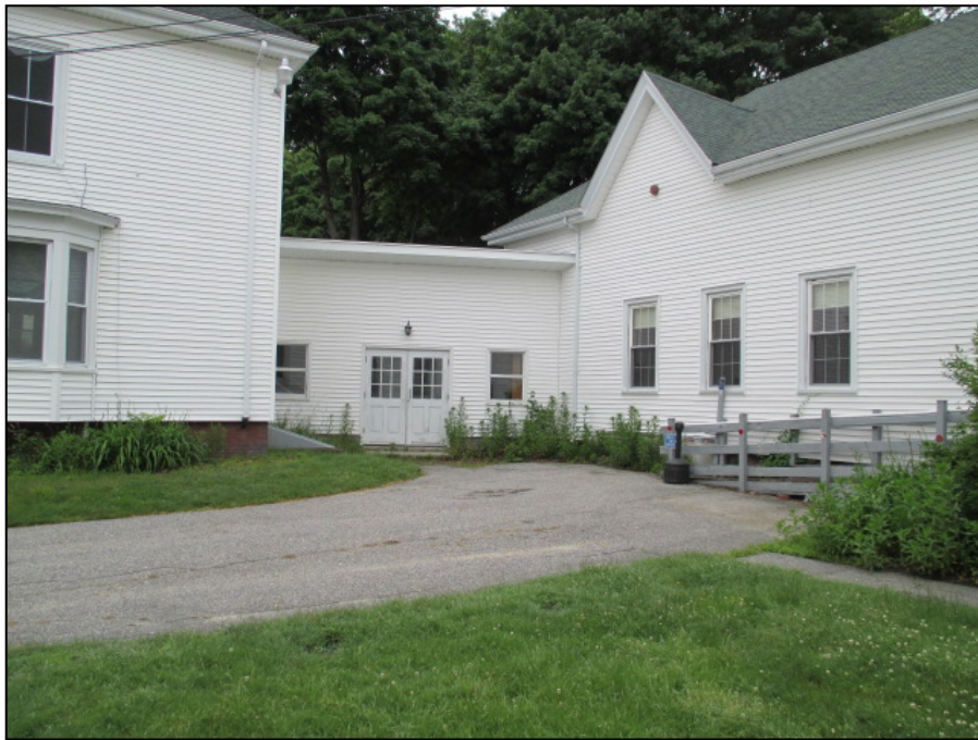
PHOTO 4 – Existing Breezeway Connecting Church and Rectory
