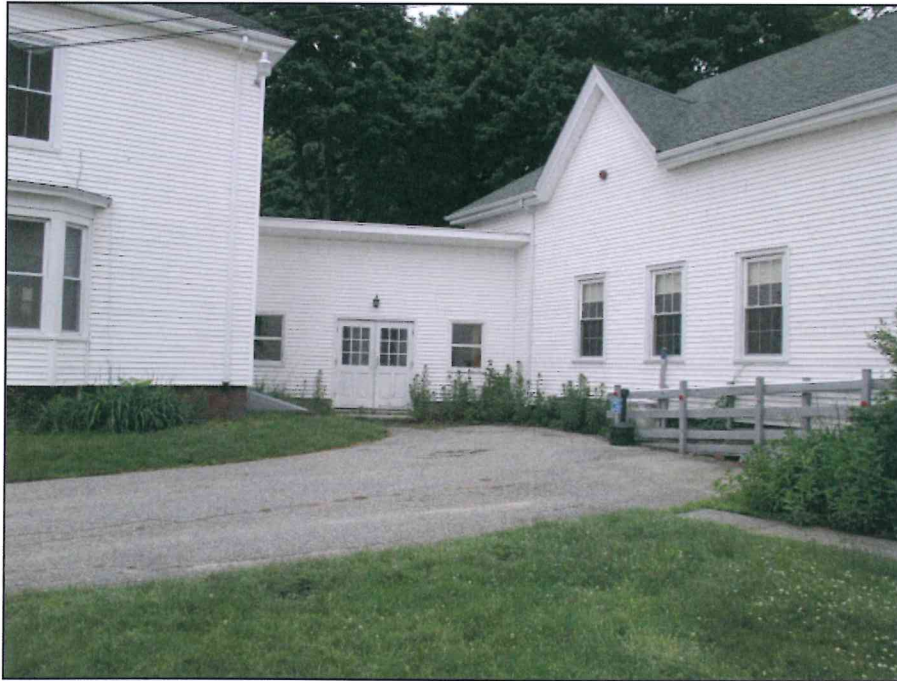
PHOTO 4 – Existing Breezeway Connecting Church and Rectory
