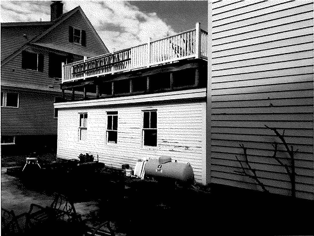
Ladder currently provides ground level egress
