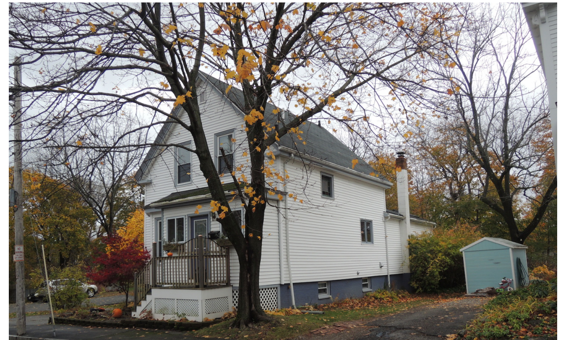
④ West Side
