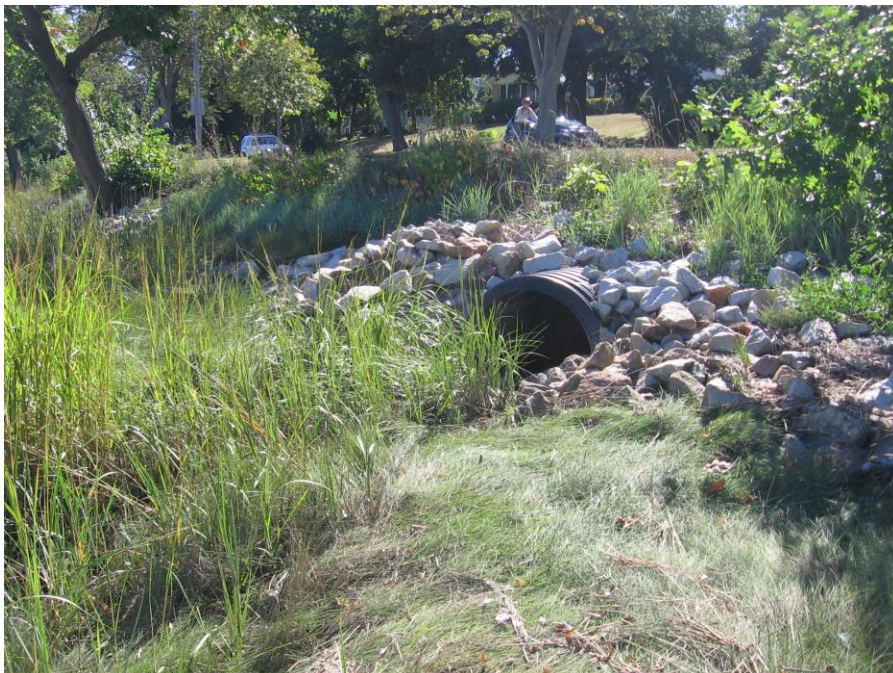
Image 4: Looking Southwest at the existing 36" outfall pipe (taken by Gary Fullerton on 9/16/16).
