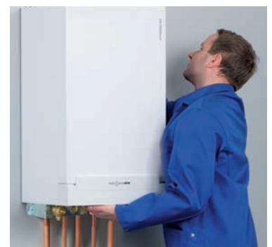
2. Mounting the boiler
