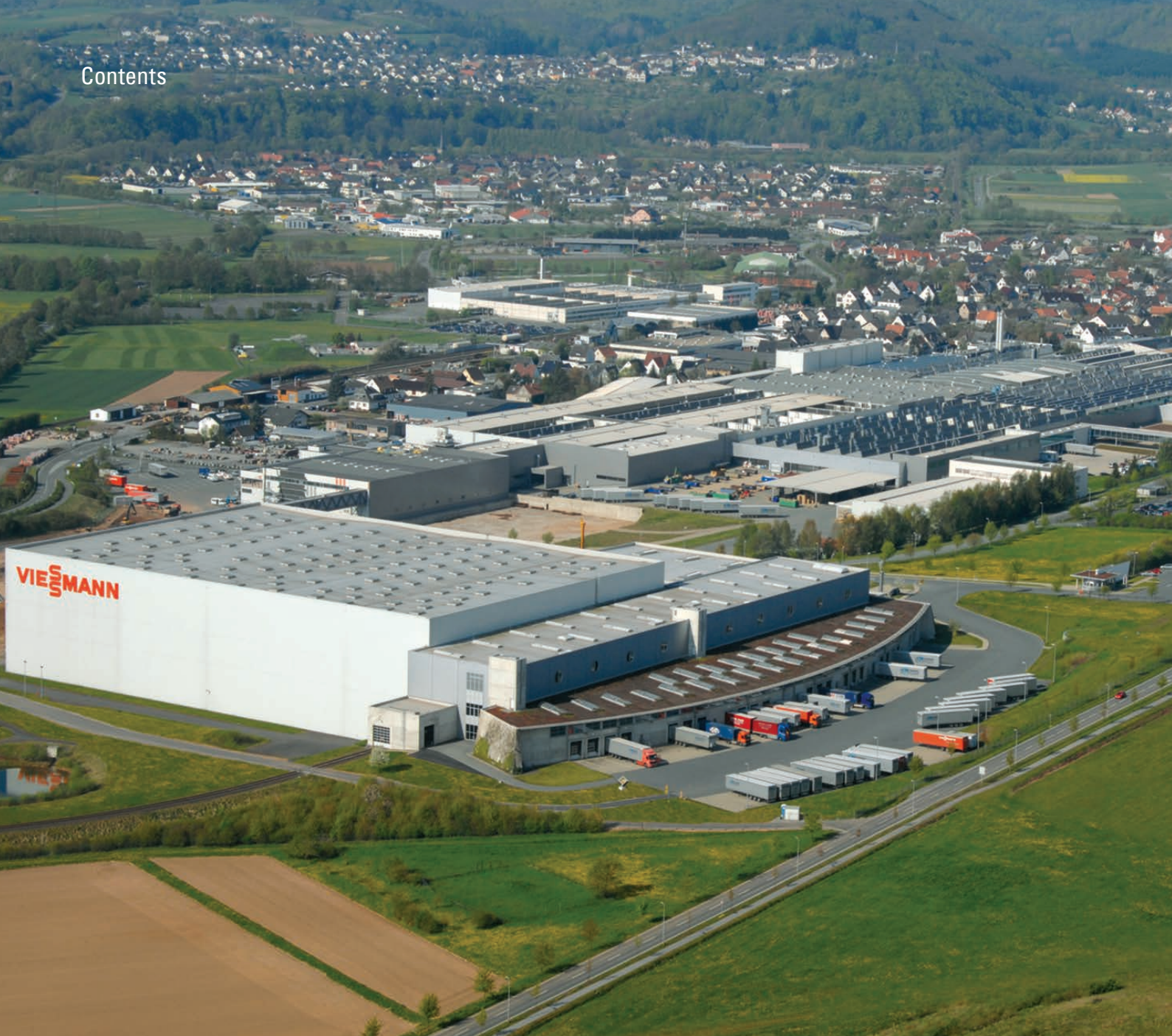
Viessmann Headquarters, Allendorf (Eder), Germany
