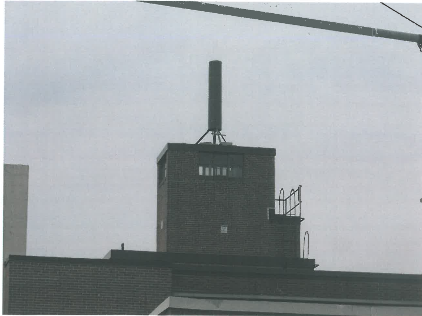
Photo 1: Sample photo showing the existing ballasted canister to be removed and replaced.
