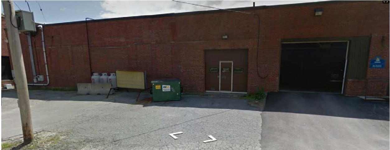
Rear of Property (Small overhead door)
