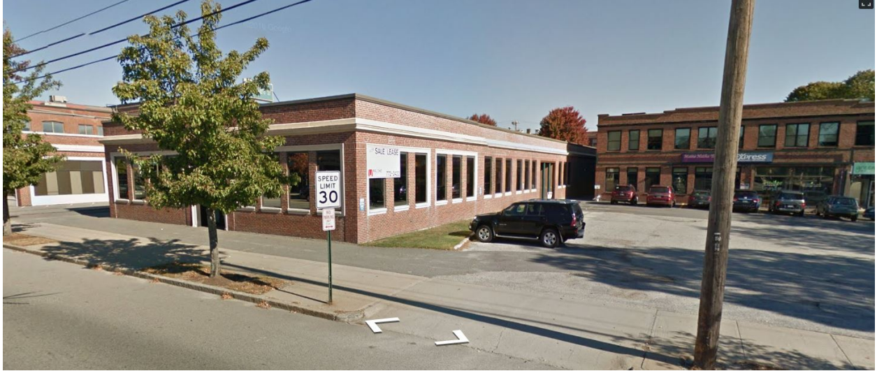
Side of Building (Retail)
