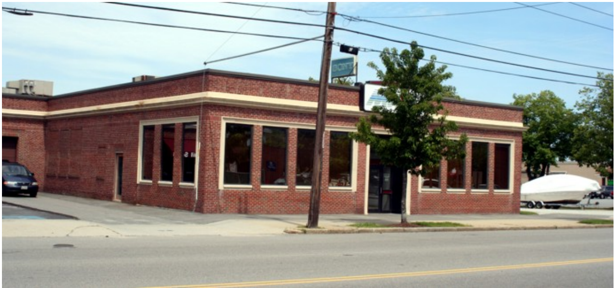
Side of Building (Retail)
