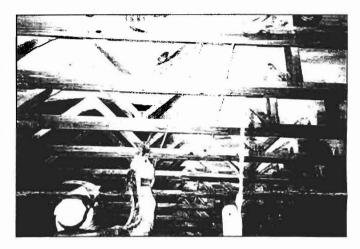
**Ideal for New and Retrofit Construction.** Heatlok 217-4 is a spray-applied cellular plastic that forms a continuous, monolithic insulation and air barrier on walls, around corners and on contoured surfaces.
