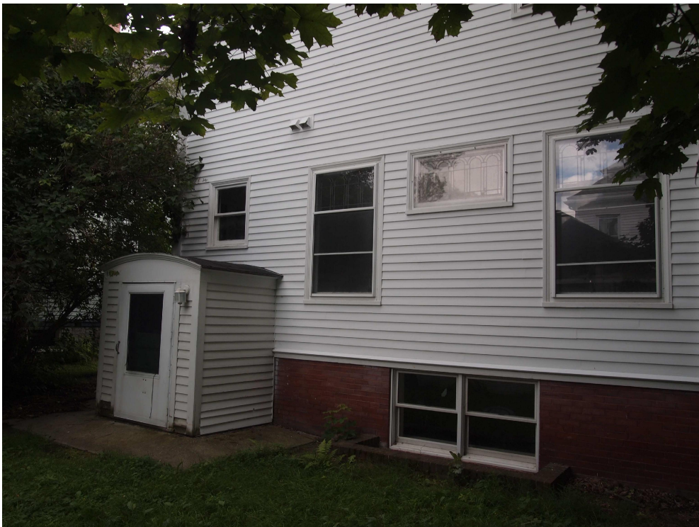
Back of house. The rear yard is boxed in on all sides with garages set on the property line.
