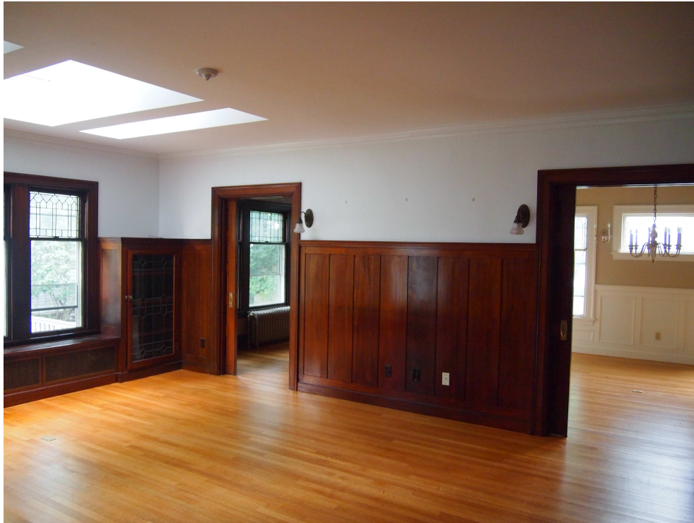
Living room looking into the dining room that will become the kitchen
