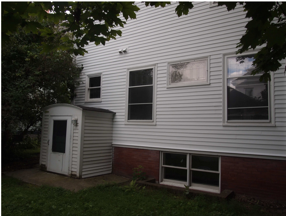
Back of house. The rear yard is boxed in on all sides with garages set on the property line.
