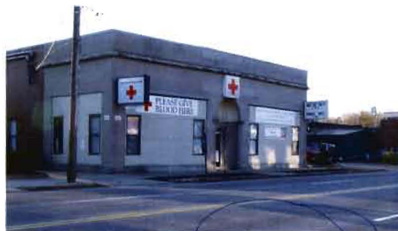
(2) 4' X 6' D/F ILLUM. PROJECTING SIGNS TO BE REMOVED (1) 4' X 4' S/F ILLUM. WALL MOUNT SIGN TO BE REMOVED
