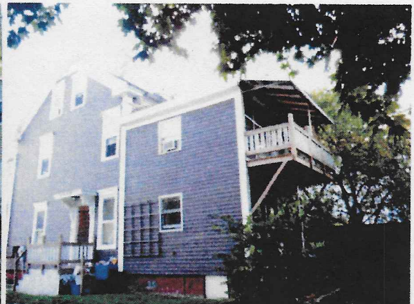
Back Exterior, Unit #4
