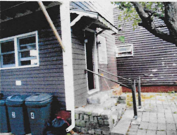
Main Door, Unit #4
