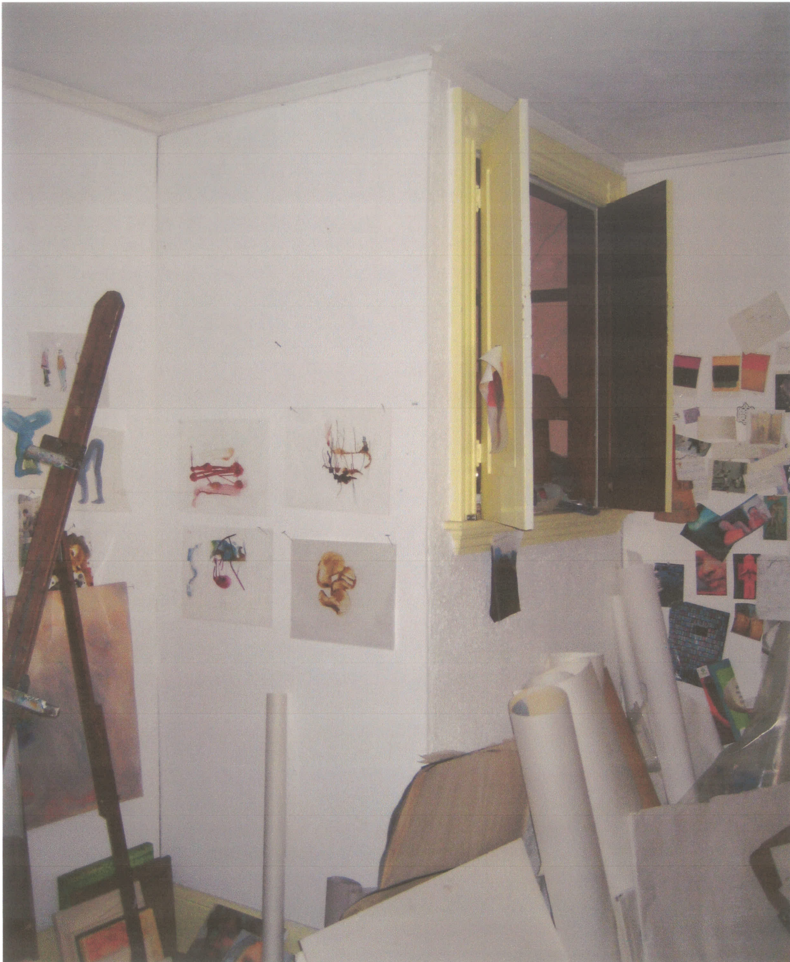
TOP FLOOR - REMOVE WALLS SHEETROCK MOVE W/D CLOSE IN FLOOR PLUMBING
