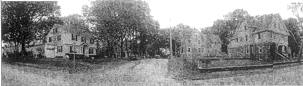
SEELEY AVENUE ENTRANCE FROM RACKLEFF STREET
