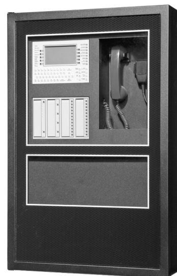
DVC Shown using CA-2 mounting option, SBB-C4, and ADDR-C4 door.
