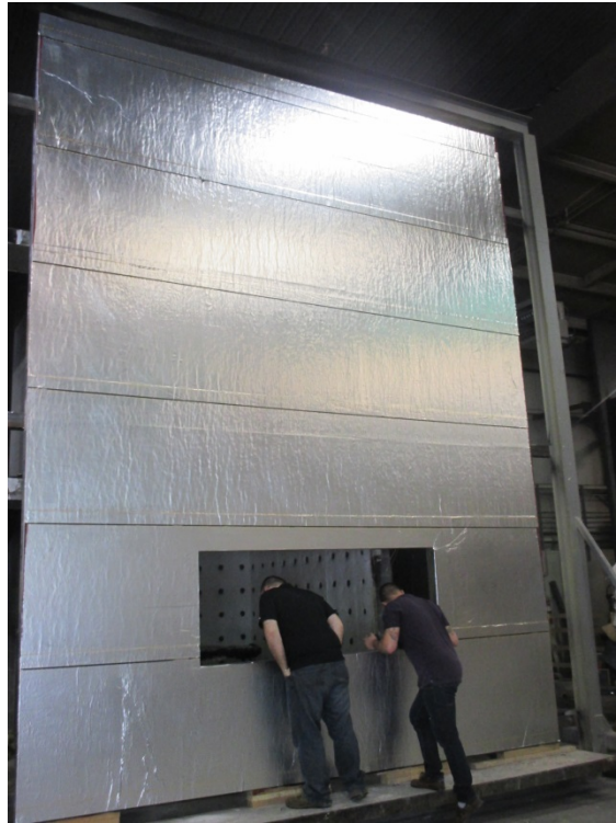
Photo No. 3 Complete installation of CCW 705-FR-A
