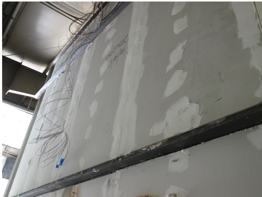
Photo No. 14 Second-story Interior Surface (Post-test)
