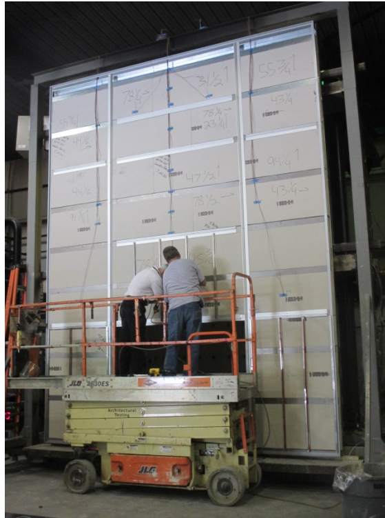
Photo No. 7 Installation of AL13 Spacers, Horizontal, Vertical, and End Extrusions
