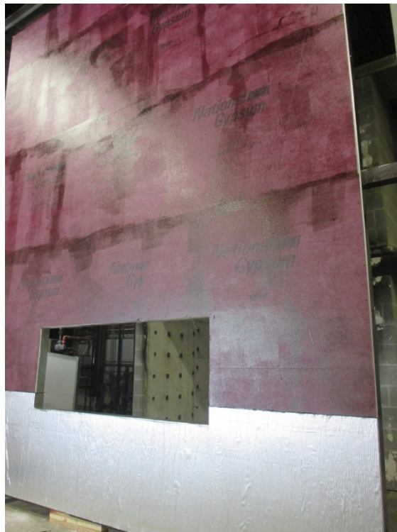
Photo No. 2 Installation of CCW 705-FR-A over CCW-702LV www.archtest.com
