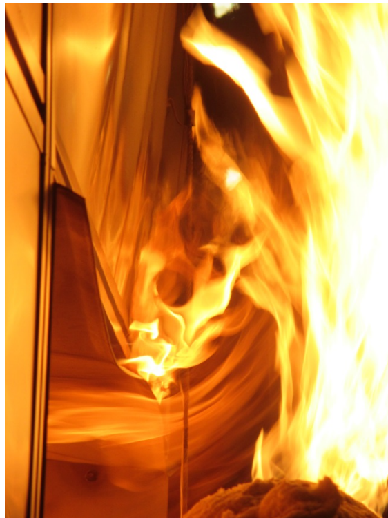
Photo No. 12 Ignition at the Window Opening Burner www.archtest.com
