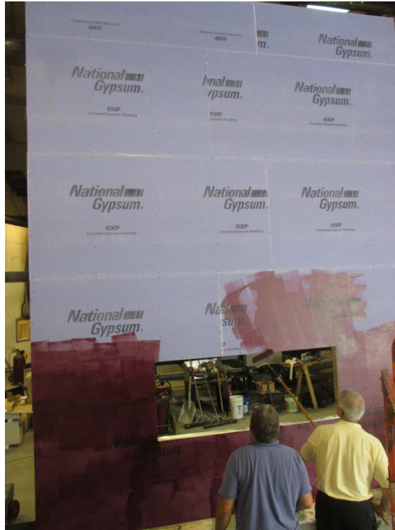
Photo No. 1 Application of CCW-702LV
