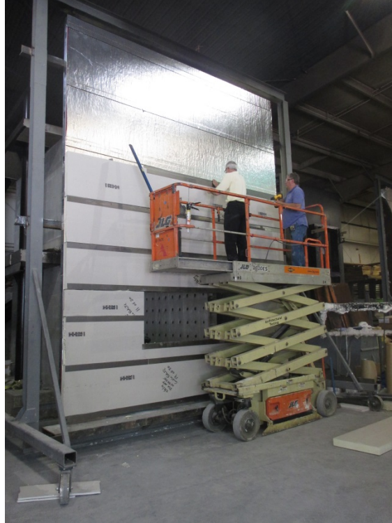
Photo No. 5 Insulation Installation
