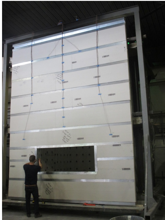
Photo No. 6 Complete Insulation Installation www.archtest.com
