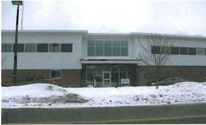
Existing Hannaford Entrance Side - Main
