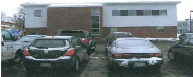
Existing Back Side - Parking
