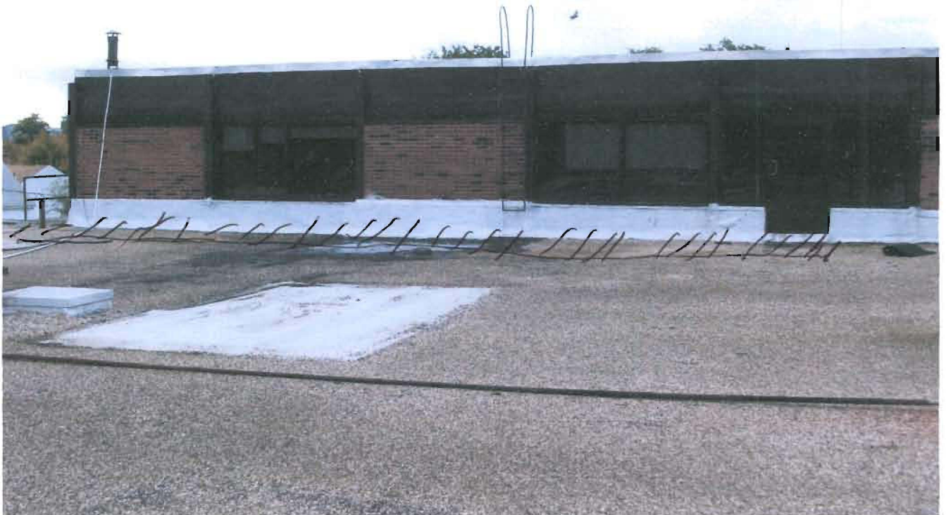
AREA OF WALKWAY
