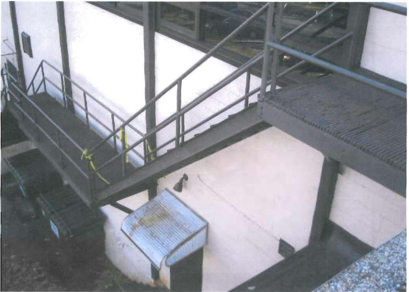
EXISTING FIRE ESCAPE STAIRWAY
