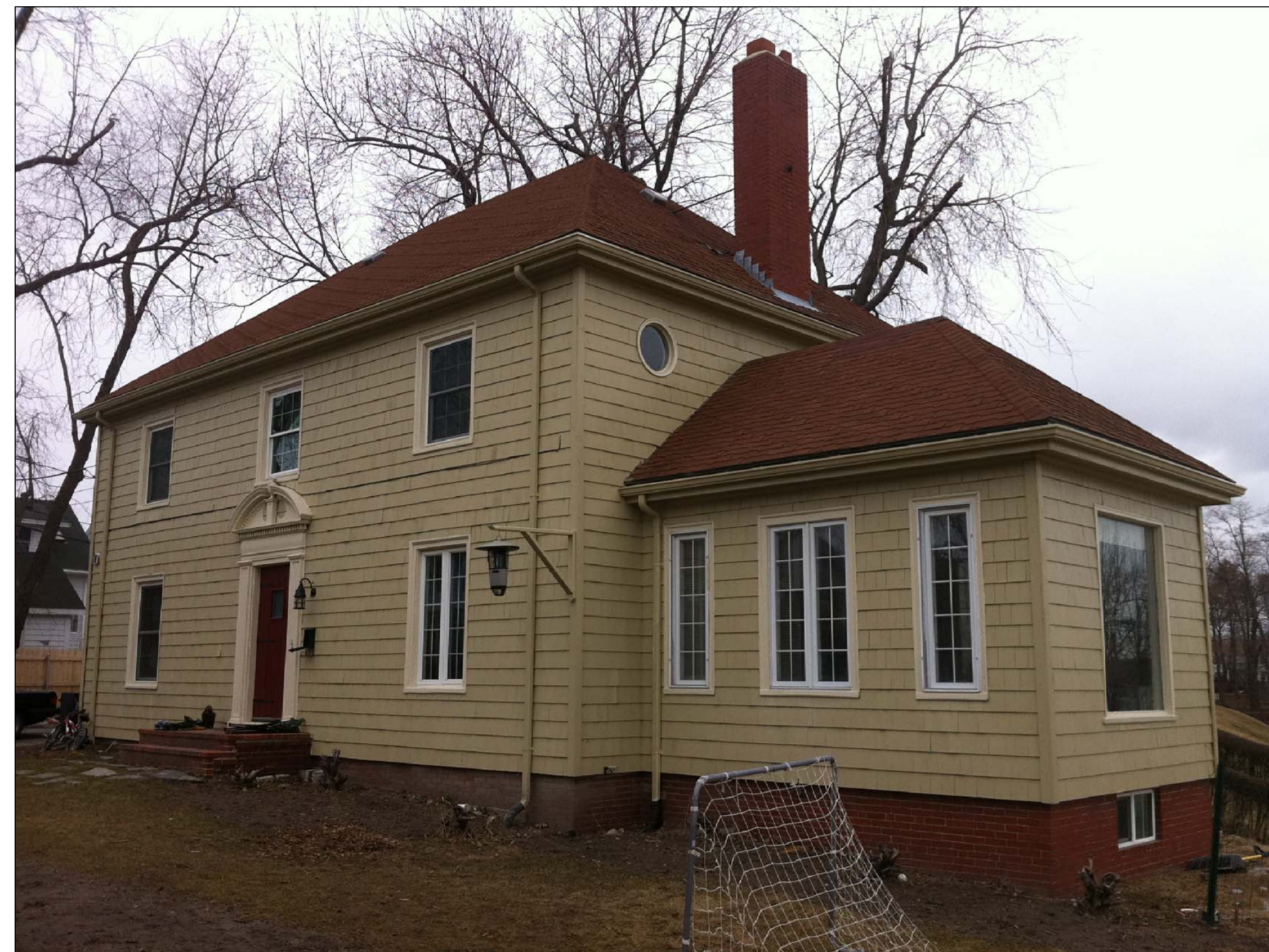
PHOTOGRAPH OF EXISTING SOUTH FACES
