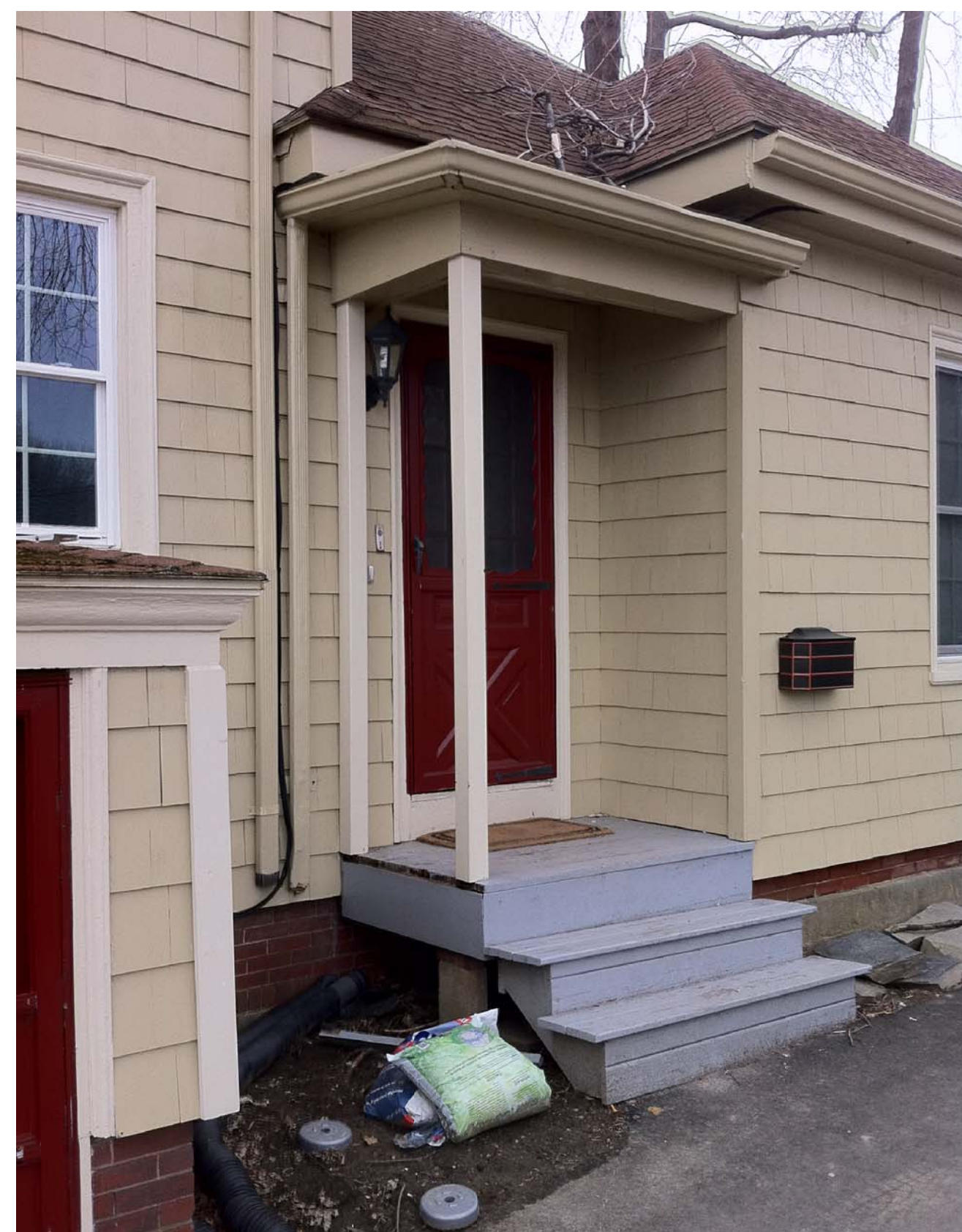
PHOTOGRAPH OF EXISTING NORTH BACK ENTRANCE TO BE REMODELED
