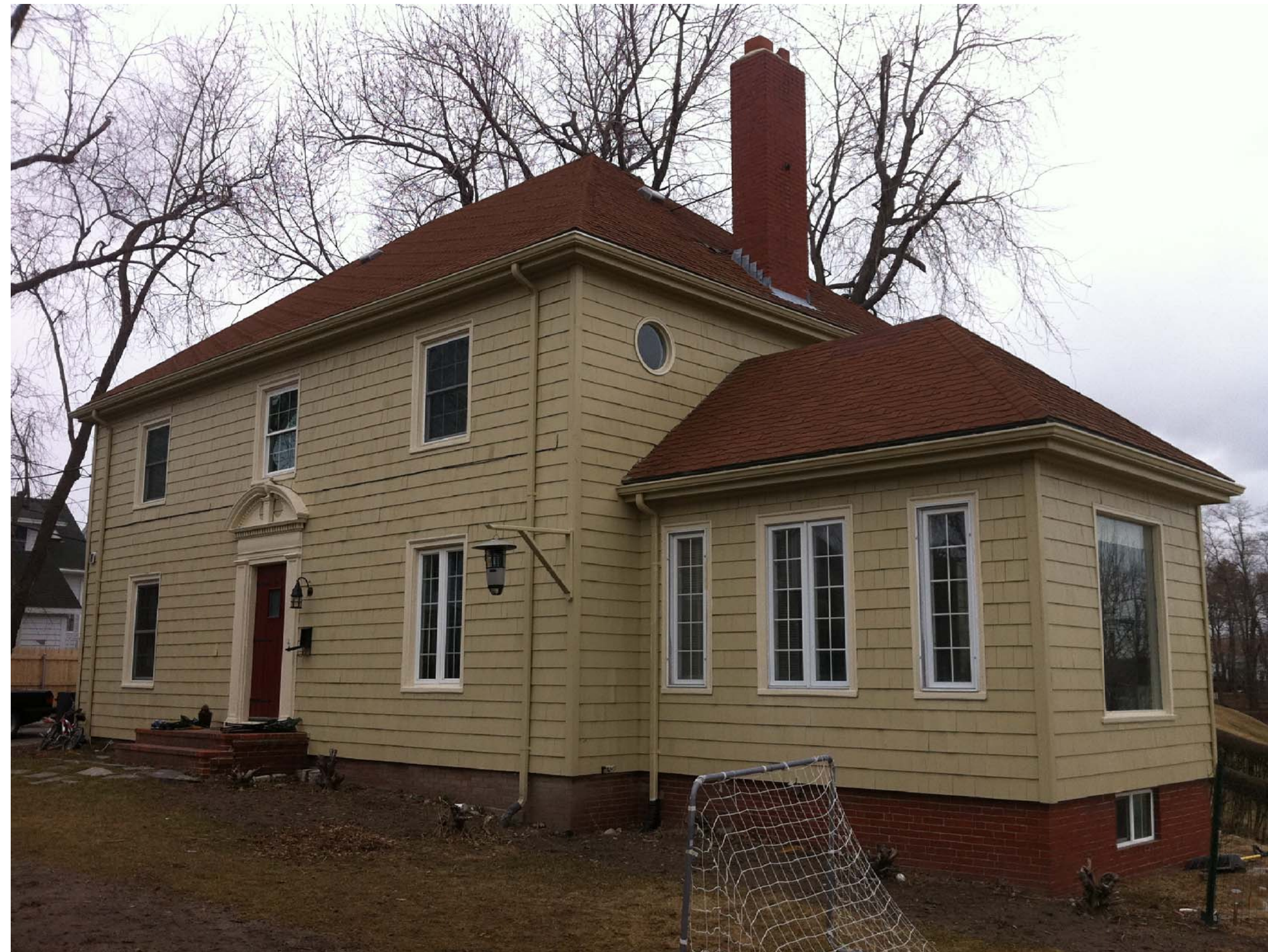
PHOTOGRAPH OF EXISTING SOUTH FACES
