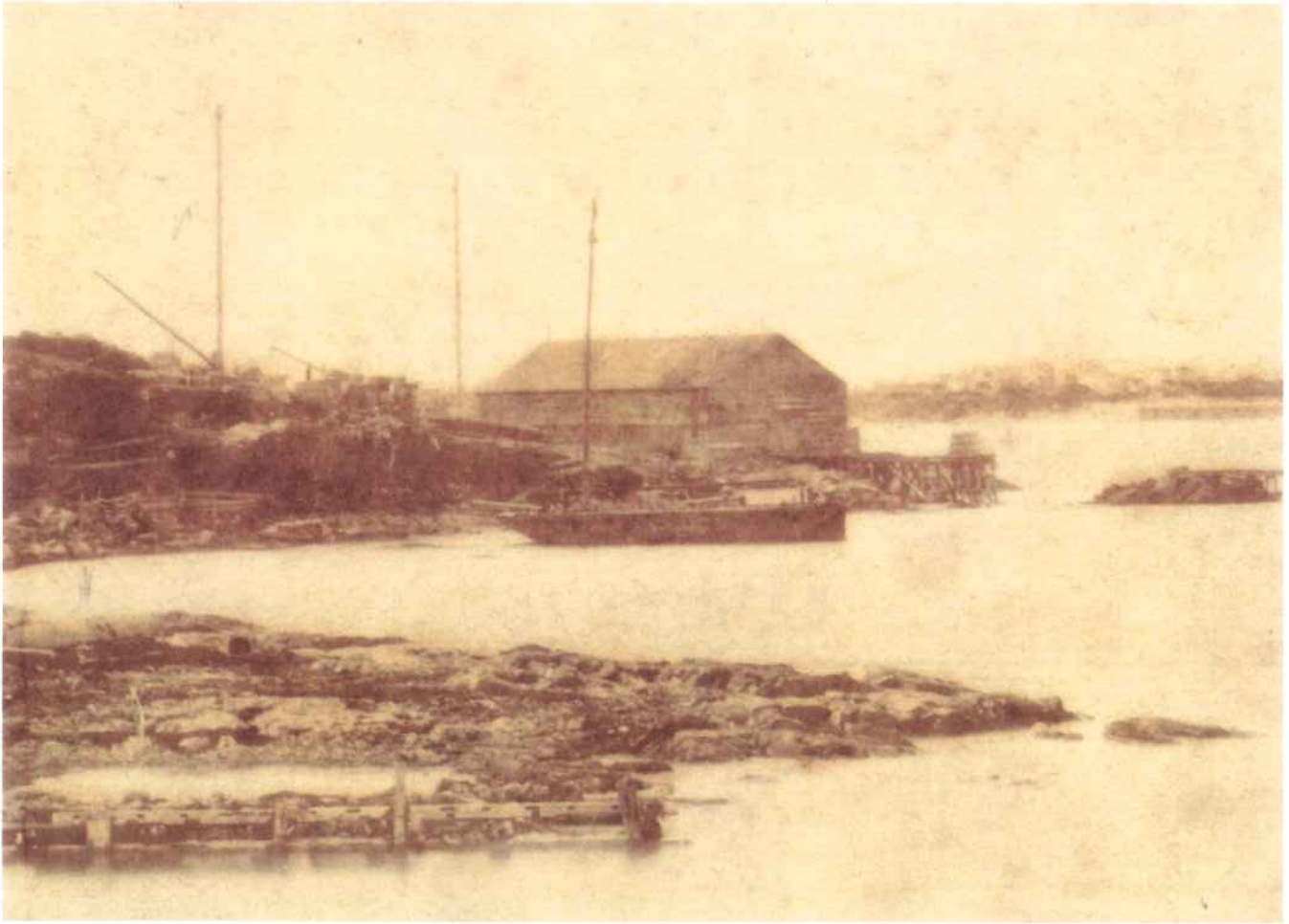
Image of a sloop near the Granite Cutting Shed (map location N) and the Old Wharf (M) a wood structure over stone cribbing. Courtesy of Kenneth E. Thompson, Jr.
